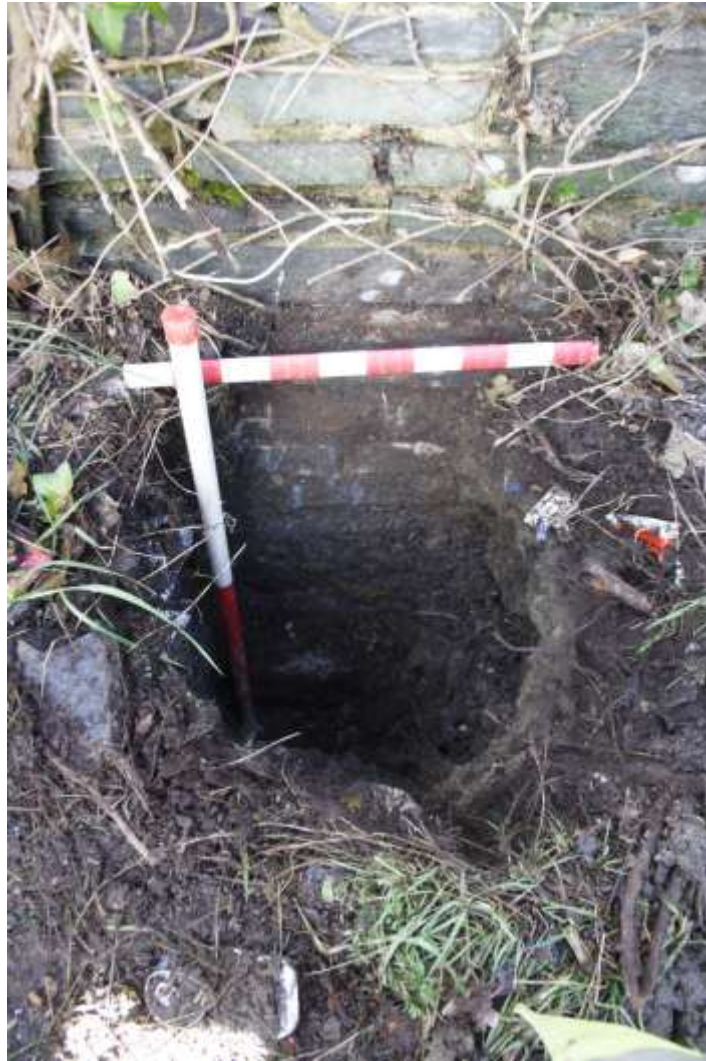
Photo 15: Test pit excavated adjacent to wall on south side of The Strand, showing foundations of 1970s built wall viewing north
