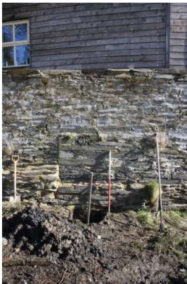
Photo 16: Test pit excavated adjacent to Cardigan Bathroom Centre wharf, showing different phases in construction
