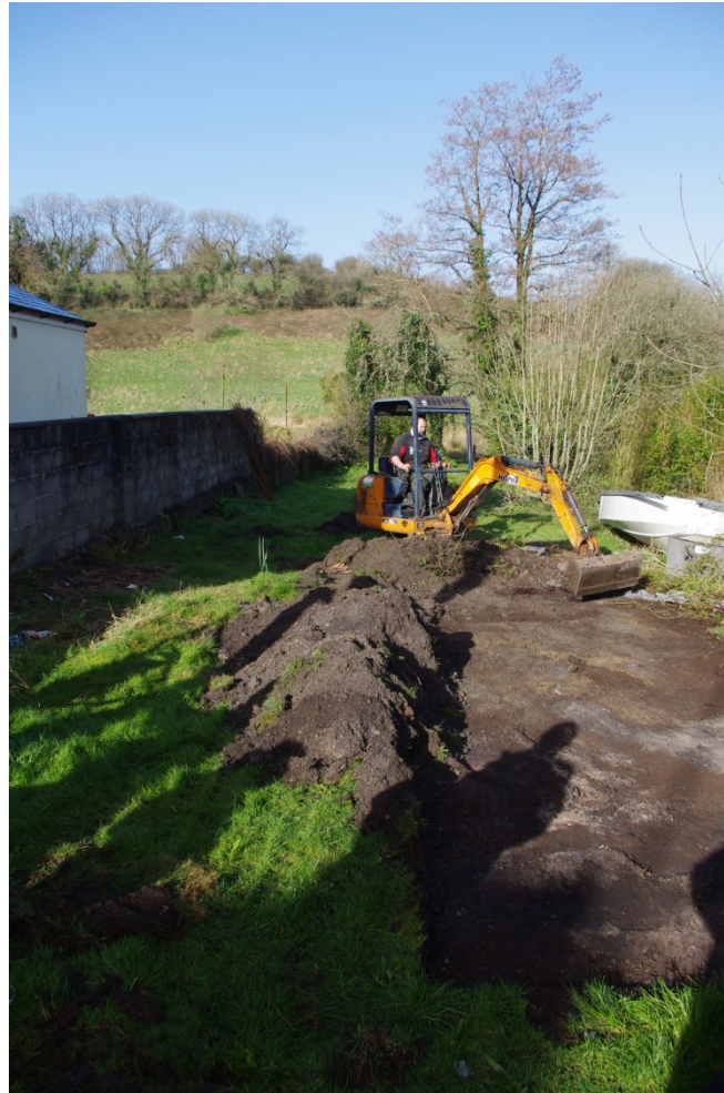
Photo 8: Topsoil stripping across site area, viewing west across Plot 1, Eldon from Clifton Street entrance
