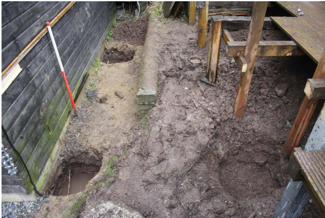
Photo 2: View north showing pits for the foundation pads. 1m scale.
