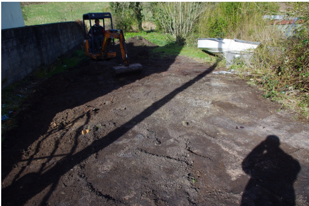
Photo 11: Completed topsoil strip of Plot 1, Eldon viewing west.
