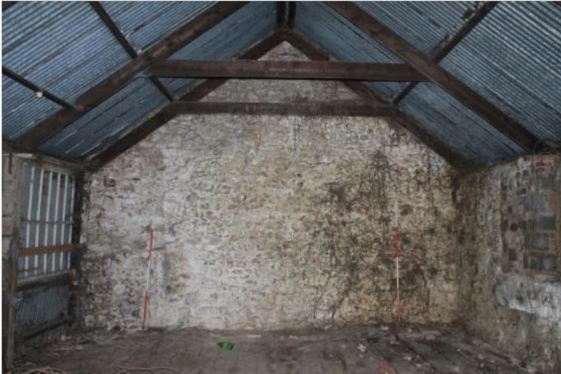
Photo 3: South wall of barn and corrugated iron roof (2x2m scales).
