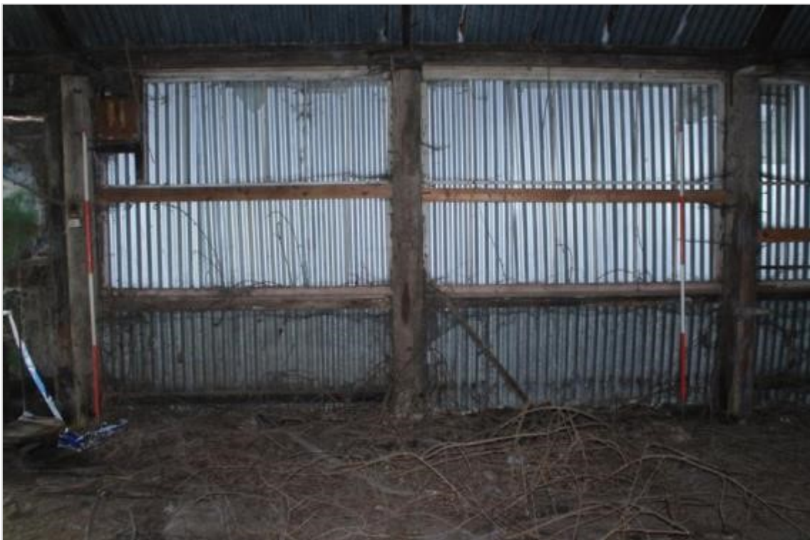
Photo 6: East facing view of post and corrugated iron side of barn (1m scale)
