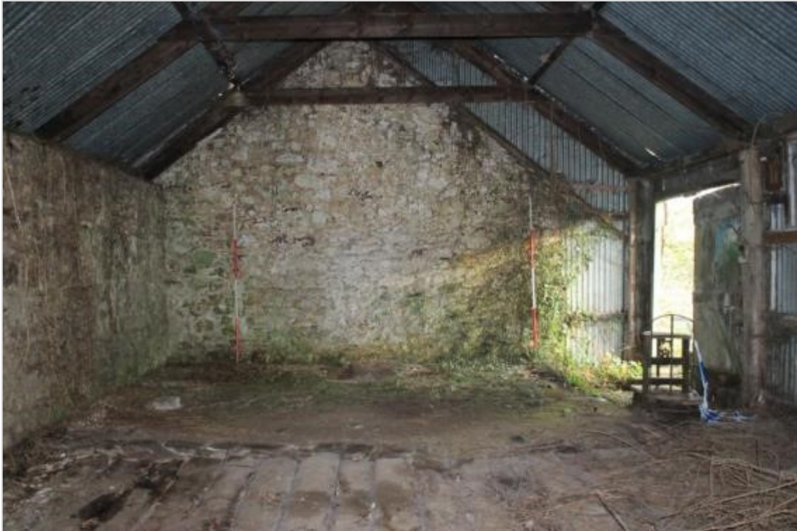
Photo 5: North wall of barn utilising narrower gable wall of adjacent building with corrugated extension (2x2m scale).
