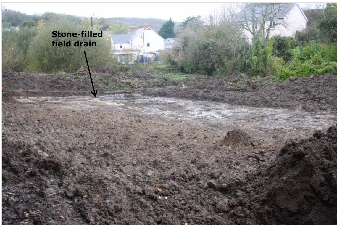
Photo 2: View northeast – Plot 1 after removal of topsoil at west end of development. Field drain can be seen as yellow linear in middle-ground.
