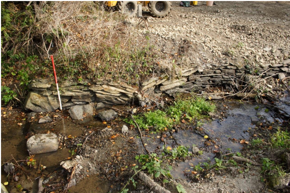
Photo 10: View north – south facing section of partly collapsed wall of canalized stream. 1m scale
