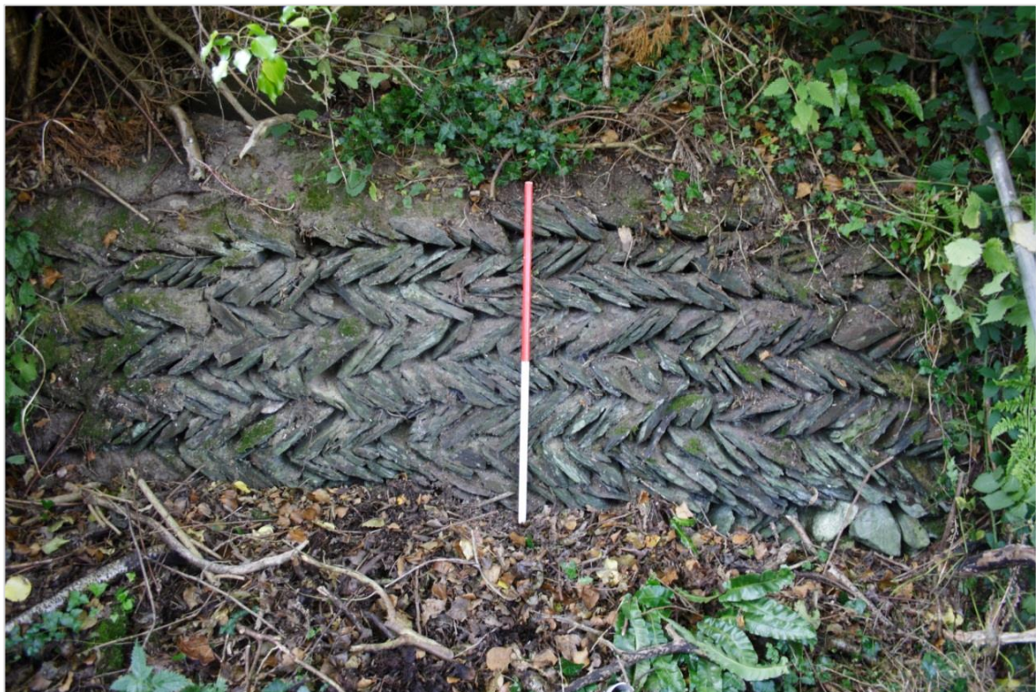
Photo 8: View north – south facing section of 'herringbone' constructed wall. 1m scale
