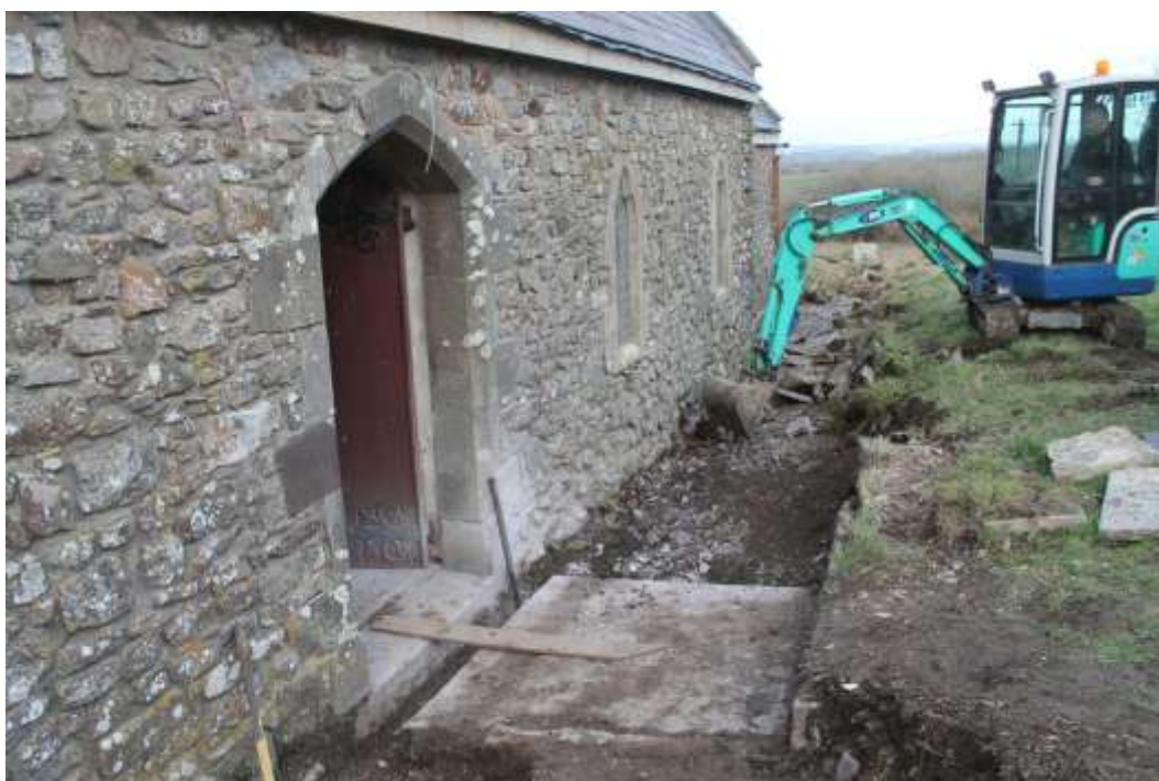
Photo 16: Excavation of drains along southern wall of St Ishmael Church
