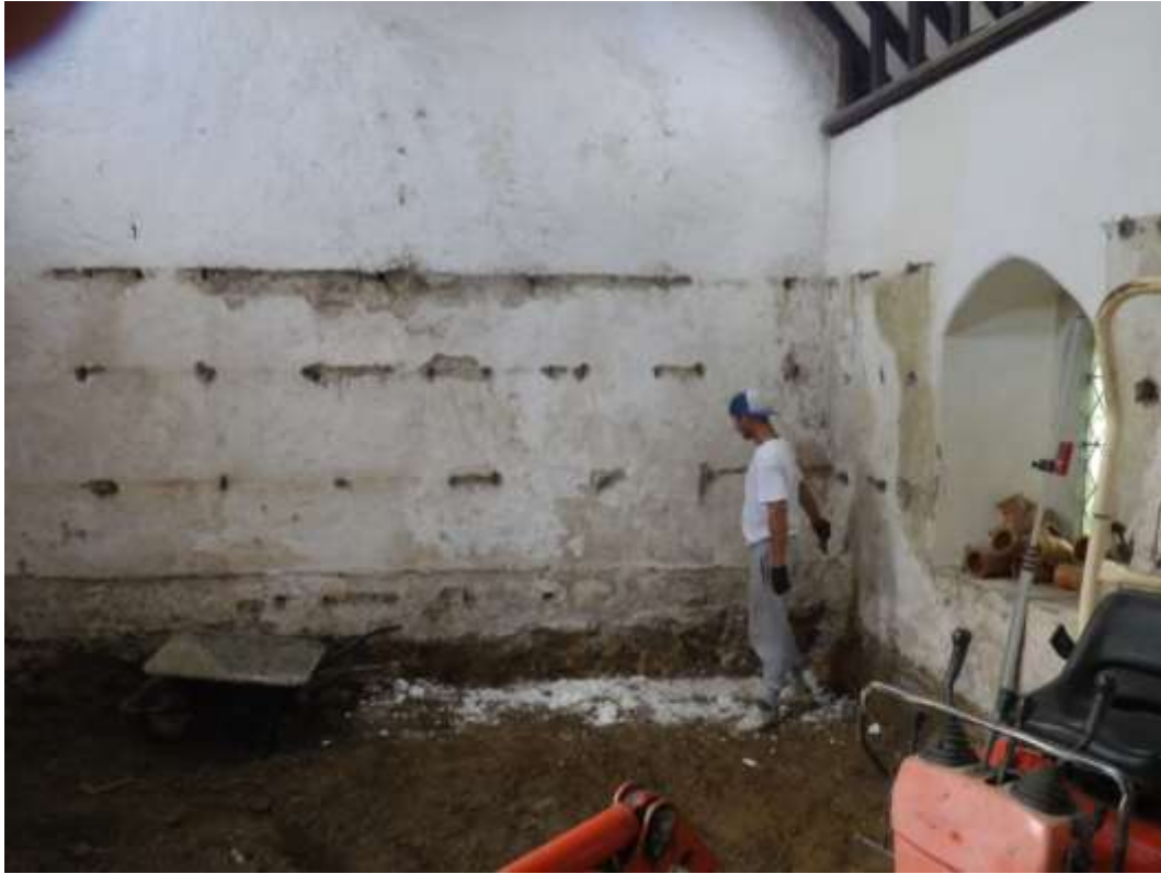
Photo 12: Plaster removal begins on the south wall at the east end of the church
