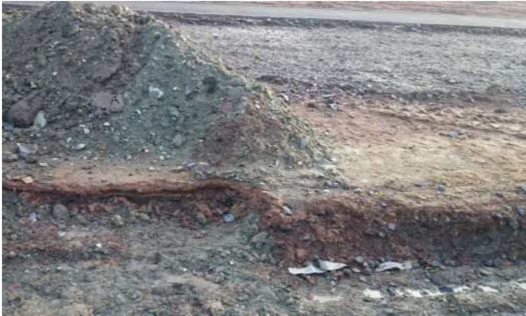
Photo 2: A vertical section through the groundworks shows the mix of fine grey and red gravels in layers making up the old surfaces of the hockey pitch
