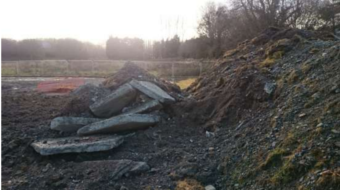
Photo 4: Looking south: An example of the spoil heaps scattered around the site, showing light sandy topsoil and turf mixed with former surface gravels, and broken concrete slabs
