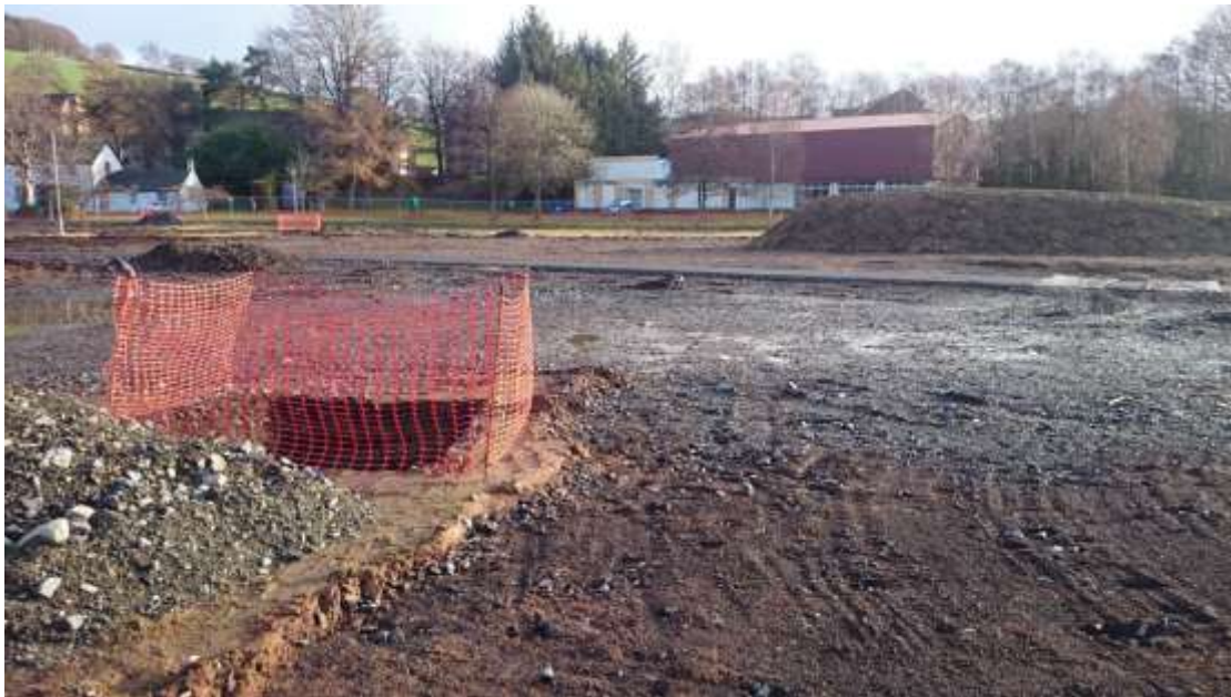
Photo 3: Looking east: One of the larger drainage holes of approximately 1.5m x 1.5m that had been dug within the area, possibly for soakaways
