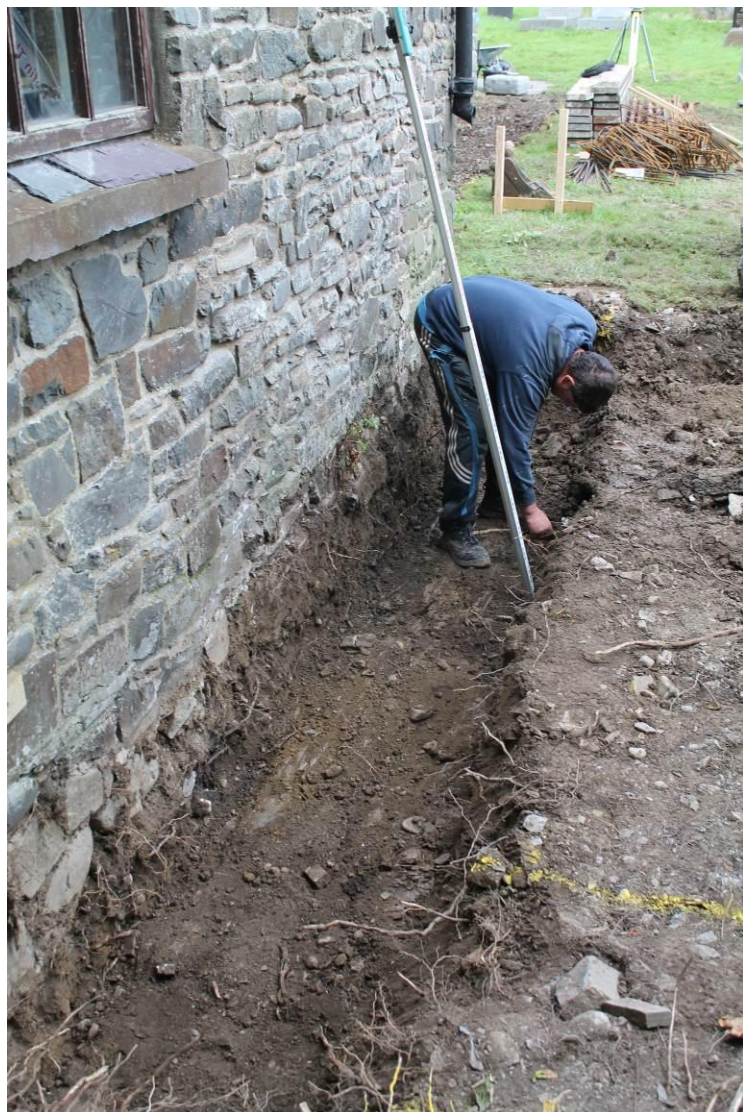
Left- Photo 2: The excavation of the foundation trench for the walls of the church extension. Photo taken facing west.
