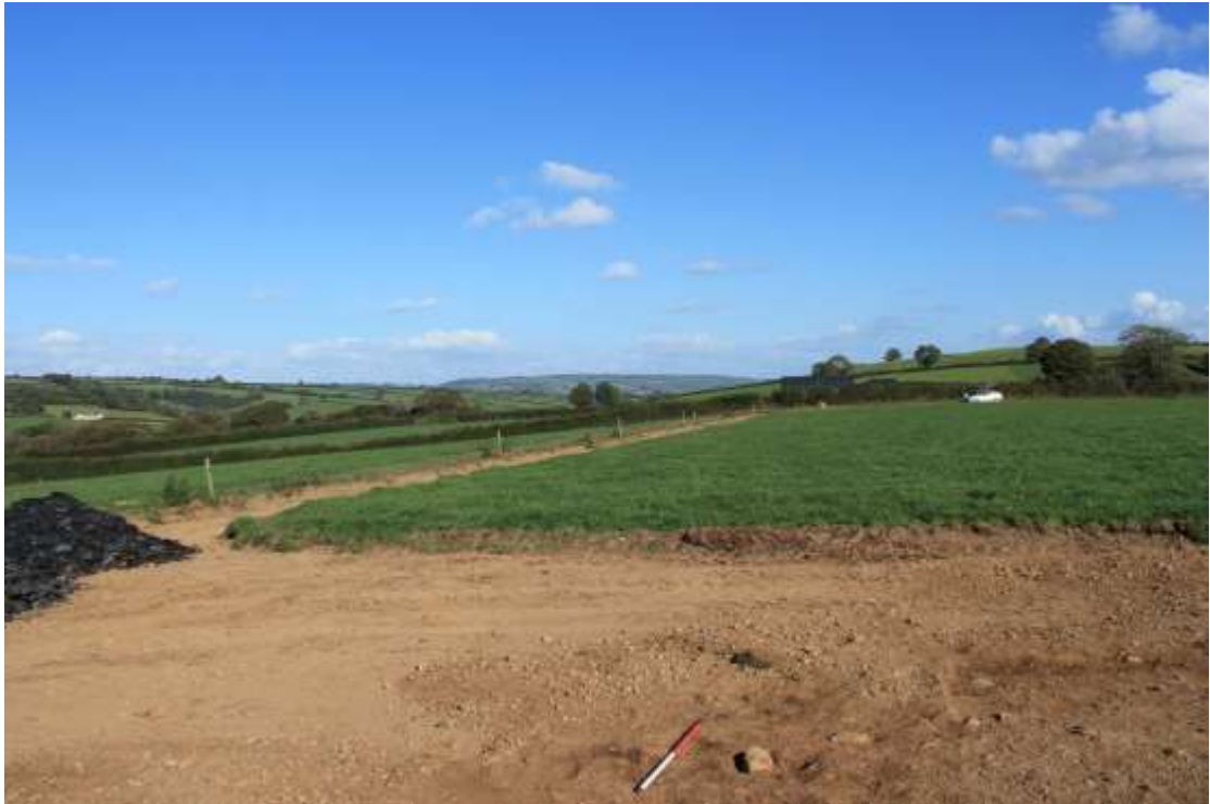
Photo 4: Proposed turbine area facing north-east. Notice the shale being used to fill in the access route to make a road.
