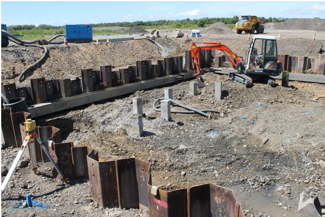
Photo 3: Sheet piles around the area of the proposed pumping station
