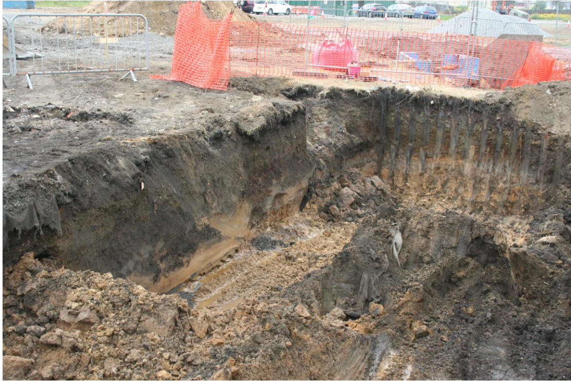
Photo 1: View of excavated area showing disturbed upper layers of 'built material' caused by site levelling.
