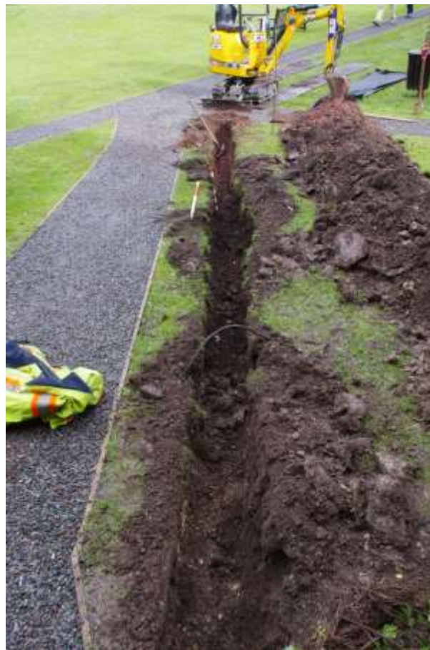
Photo 20: Northeast view along Section 8 showing loose brown soil across most of the trench, with the red sandstone bedrock at the northeastern end
