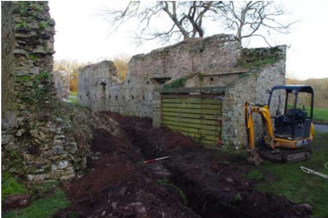
Photo 7: View southeast at western end of barn showing cable trench and line of observed wall (marked by the 1m scale)
