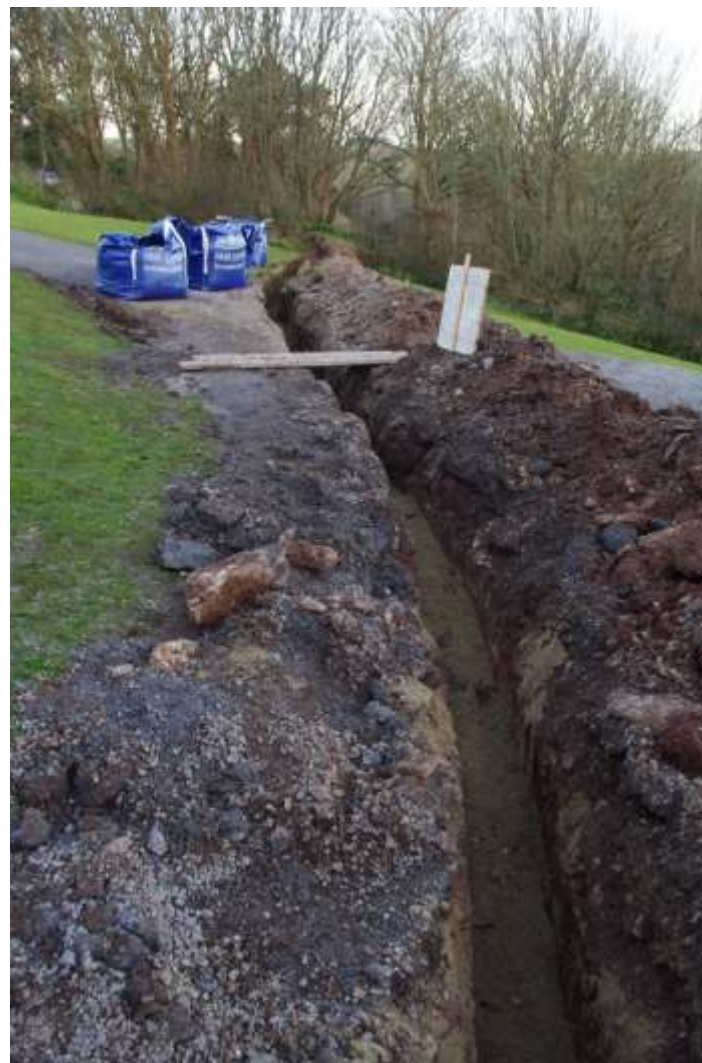
Photo 4: View southwards along Section 2 of cable trench across grassed area and driveway to castle towards woodland (following sand infill in readiness for cable)
