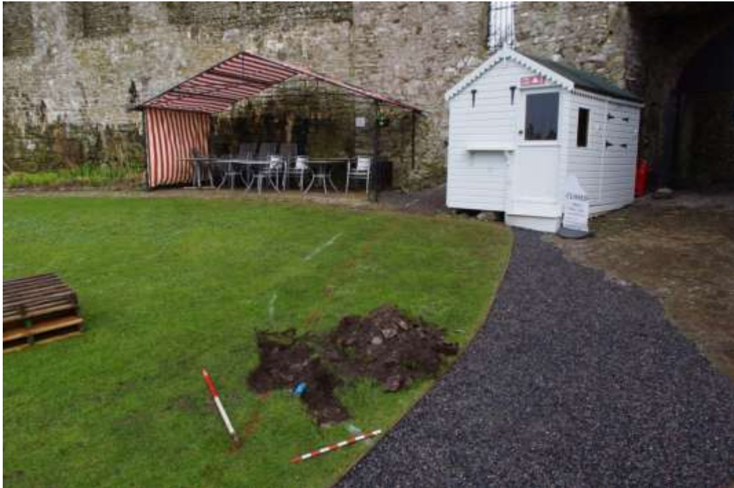
Photo 14: Section 6 of the cable run across the lawn within the inner ward of the castle. Note the test pit with visible existing service. Looking northeast.
