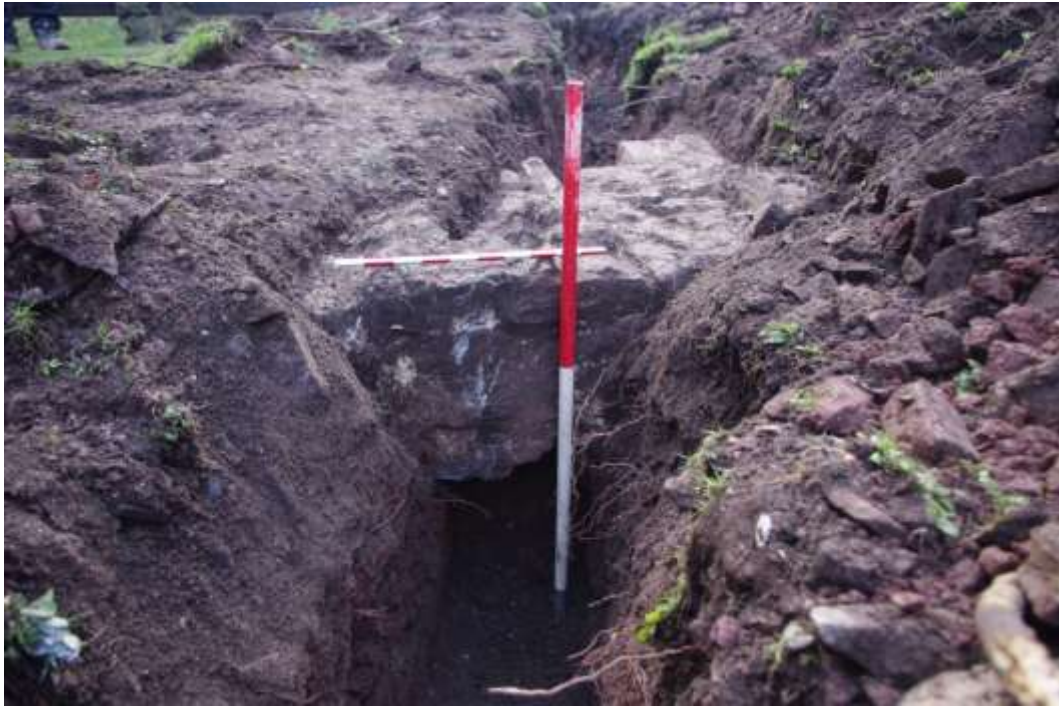
Photo 10: View east of exposed western wall of barn in Section 3 of cable trench showing shallow depth of wall and the void for the cable excavated beneath
