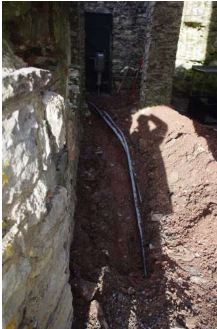
Photo 13: Cable run through buildings on inside of inner curtain wall, following the route of existing services, looking northeast
