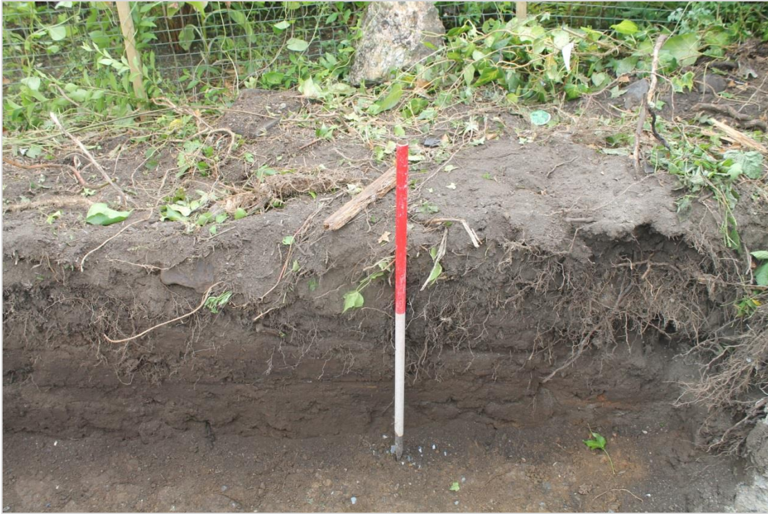
Photo 9: Photograph taken looking east showing the machine excavated wall foundation trench. Note the homogenous loamy garden soil above the natural yellow clay subsoil seen at the bottom of the trench. 1m scale
