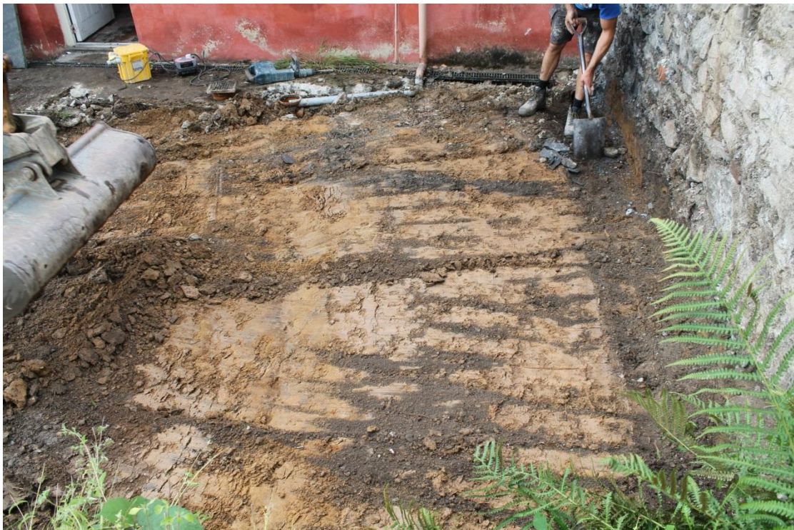
Photo 2: Photograph taken looking south showing the natural yellow/brown clay subsoil revealed after the removal of the stone paving. A modern drainage trench runs parallel with the west wall.
