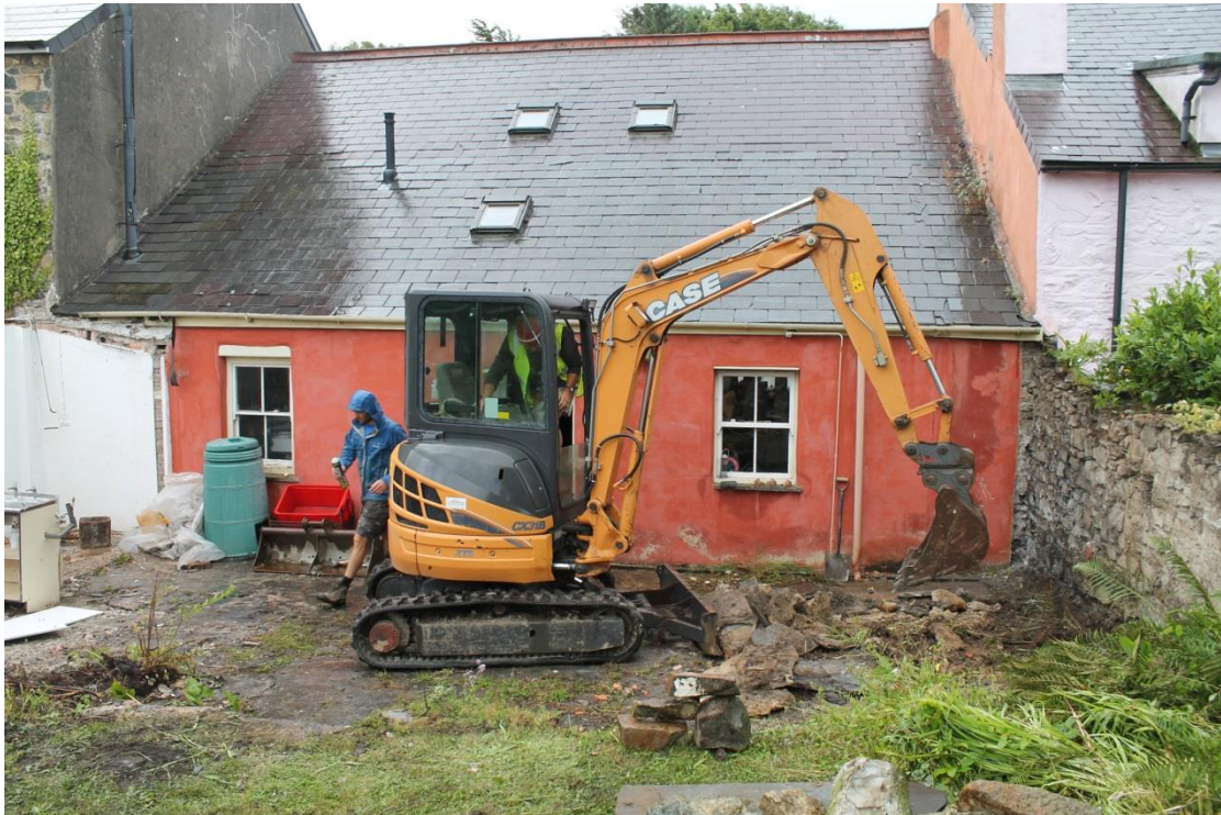
Photo 1: Photograph taken looking south showing the machining of the stone paving.
