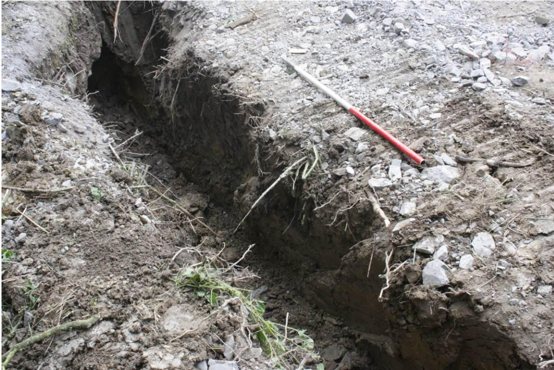
Photo 2: Excavation of drainage trench (Phase 2).
