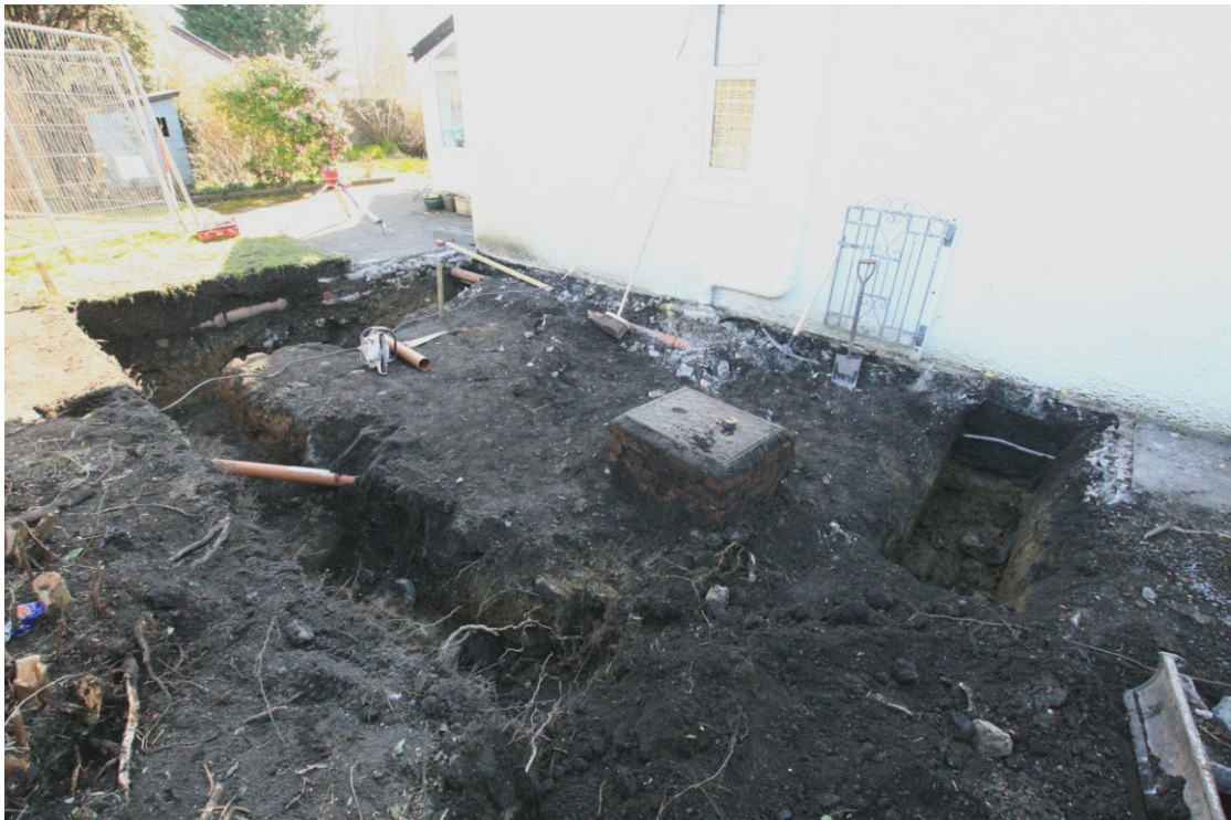
Photo 2: Southwest facing view of development area showing the foundation trench excavated for the footings of the extension.
