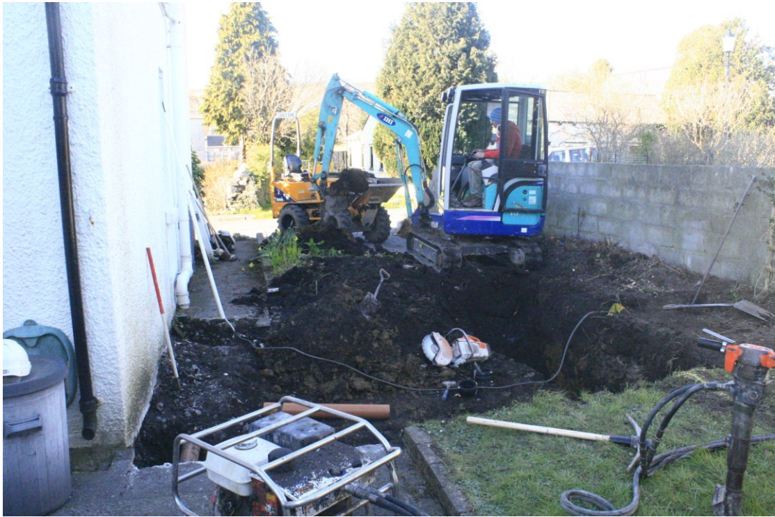
Photo 1: North facing view showing machining of foundation trench in progress.
