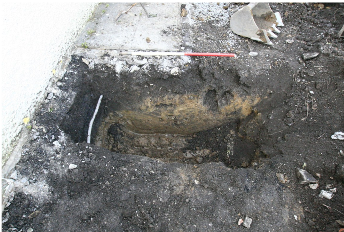
Photo 6: South facing section of northern side of foundation trench where it meets the wall of the property showing the shallow depth of topsoil (200) and subsoil (201) above the natural clay (202).
