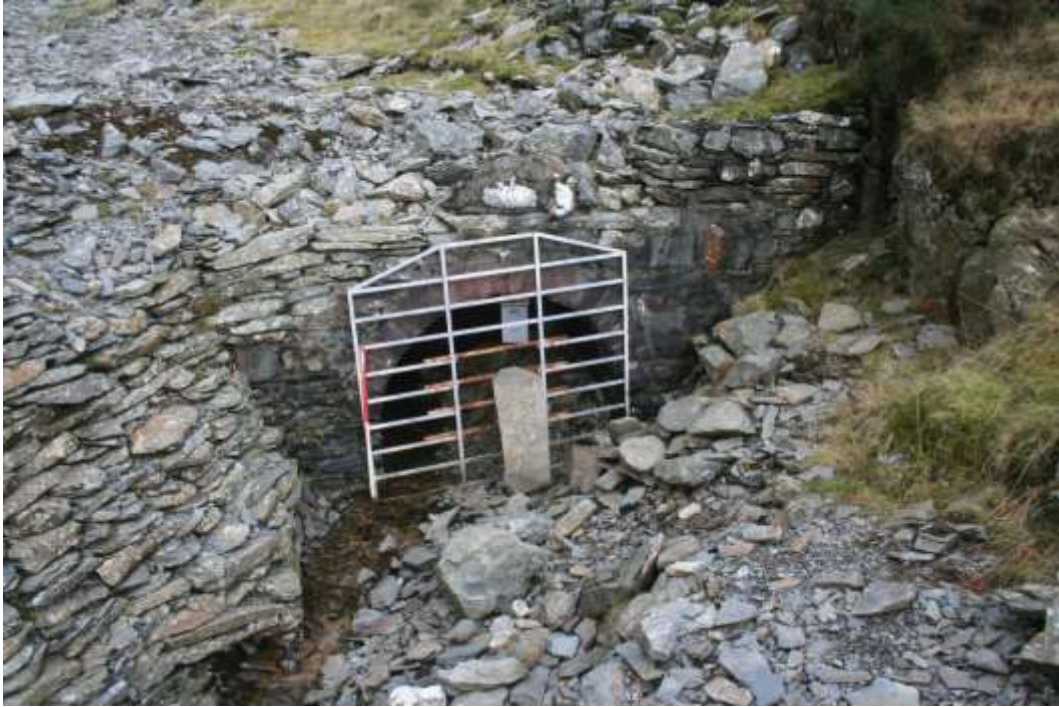
Existing inappropriately placed barrier to Taylor's Level
