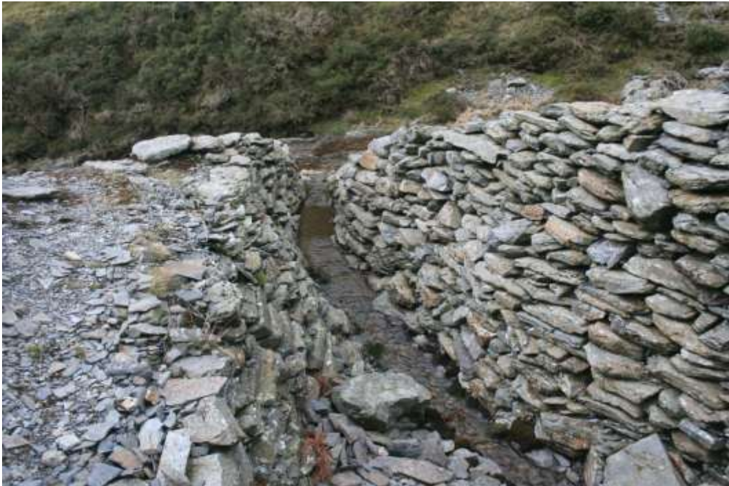
Dry stone packwall entrance to Taylor's Level
