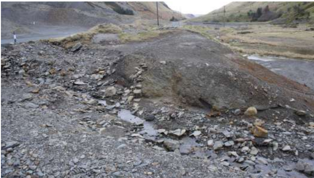
Photo showing eroding slimes dump south of the road
