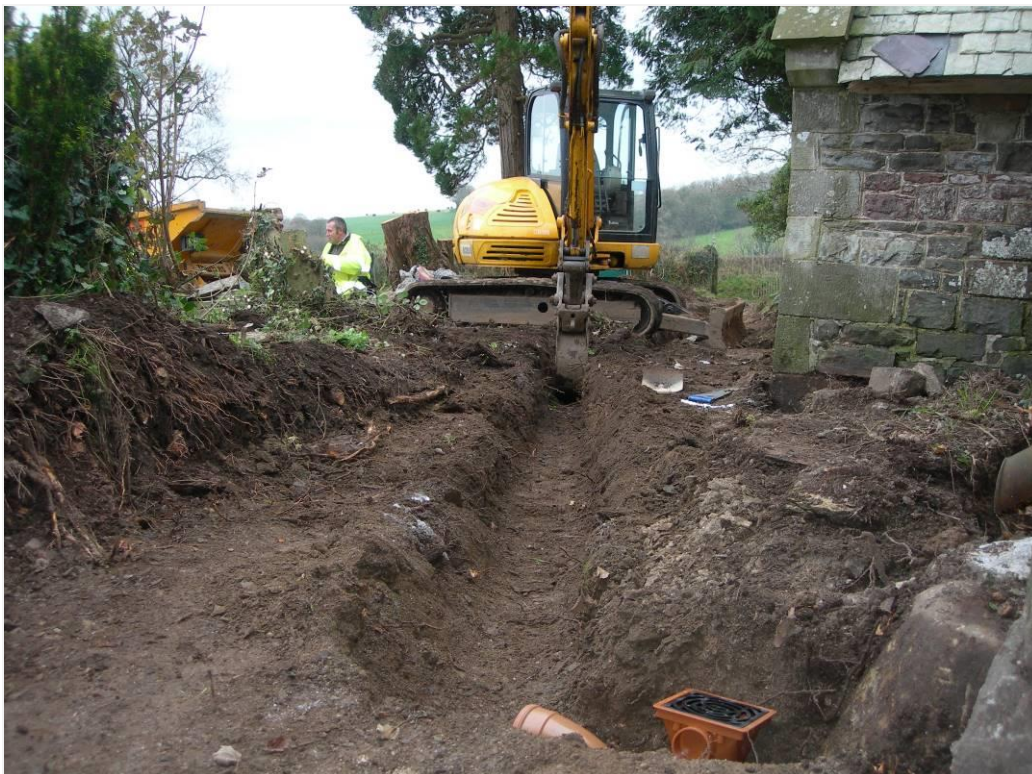
Photo 29: The machine excavation of the perimeter drainage trench south of the church. Facing east
