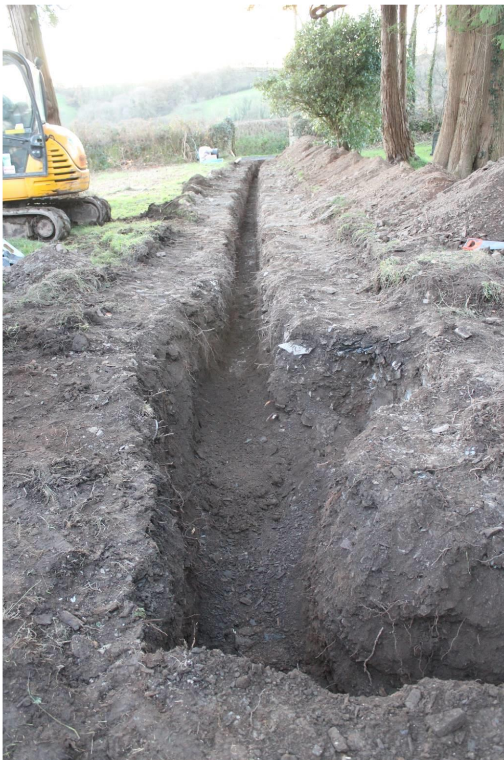
Photo 45: The machine excavated drainage trench that ran from the church to the west gate. Facing west
