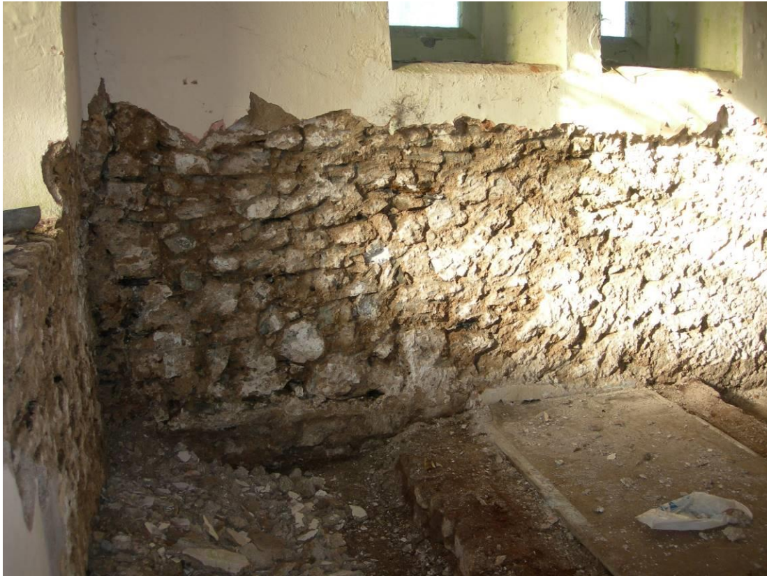
Photo 40: The west end of the church after removal of the wall plaster showing the rough stone wall construction underneath.
