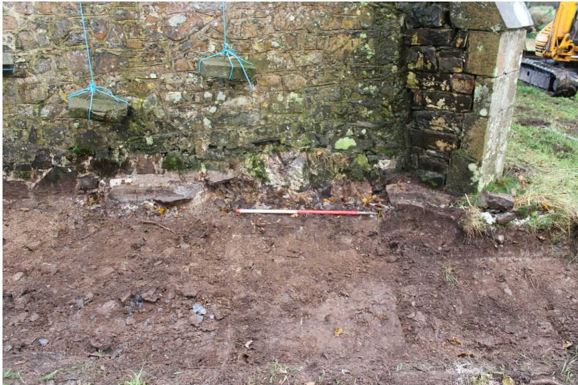
Photo 28: The large foundation stones protruding from beneath the north wall of the church building. Facing south. 1m scale
