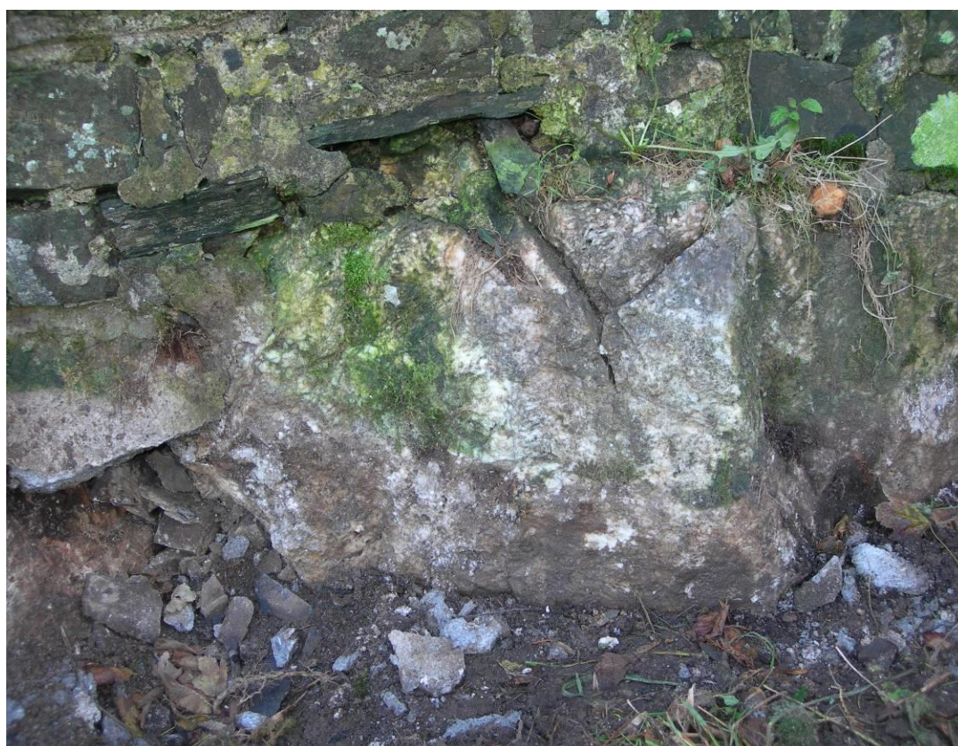
Photo 3: View of quartz blocks within later wall structure of nave.
