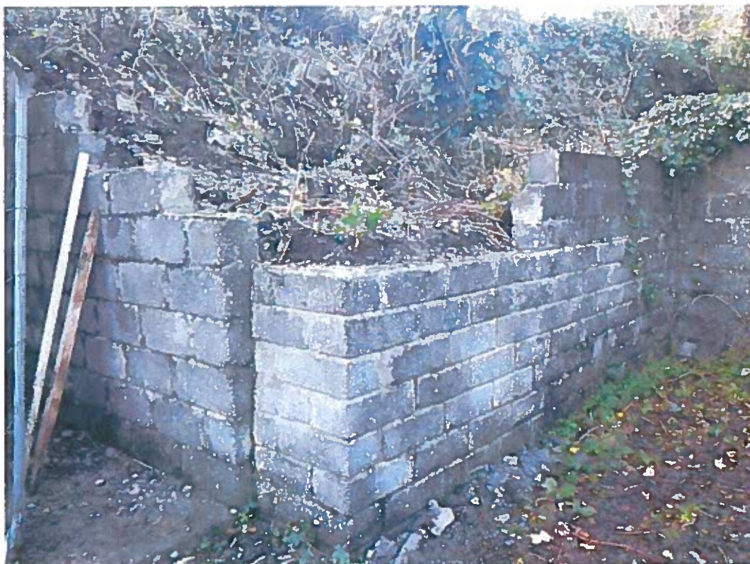
Photo 2: Dog-leg in revetment wall with lower level terraced area
