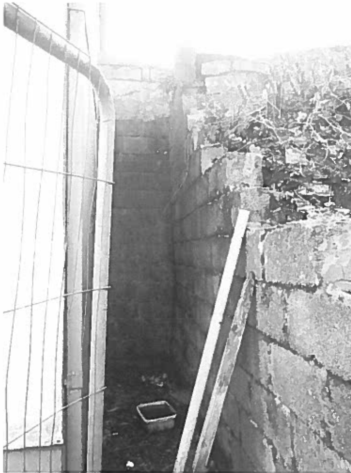
Photo 1: Area of failing breeze-block revetment wall adjacent to neighbouring property
