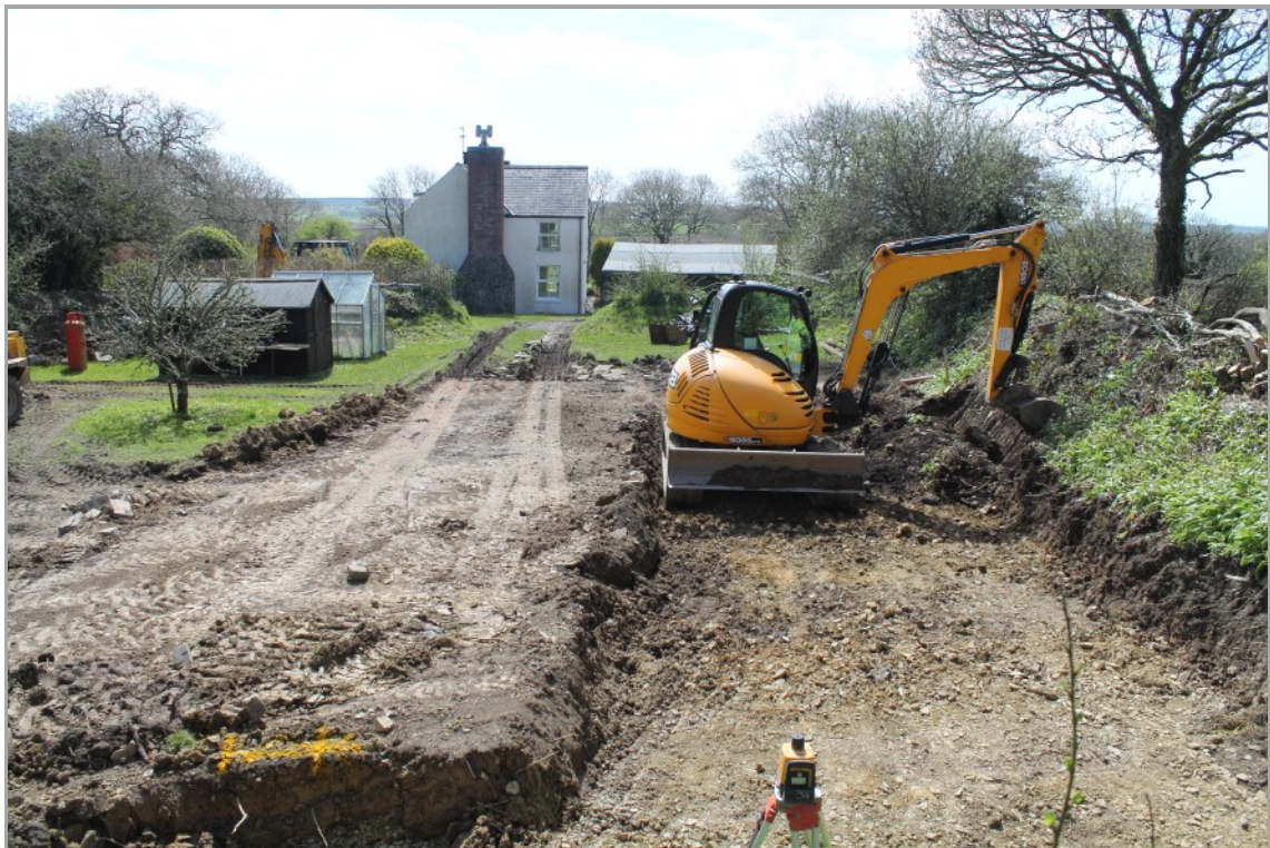
Photo 6: Looking southwest across the development site during the excavation to formation levels. A naturally-occurring stony subsoil/fragmented bedrock is visible throughout. Park Cottage can be seen in the background.
