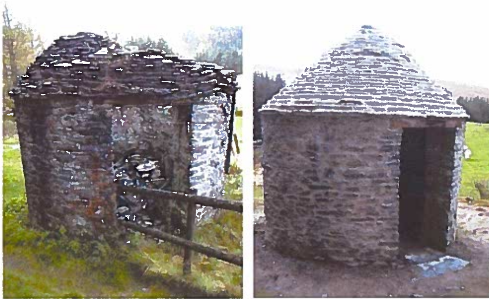
Figure 17 Llywernog mine gunpowder magazine before and after restoration as part of Spirit of the Miners Project.
