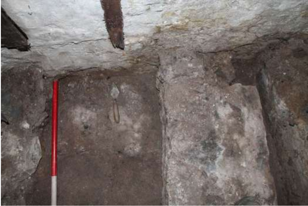
Photo 5: Foundation of wall on the inside of the south wall of the tower (with trowel upon it), with the gap in the foundation to the west with the large fragment of masonry upon it, and plinth wall to west (view south)
