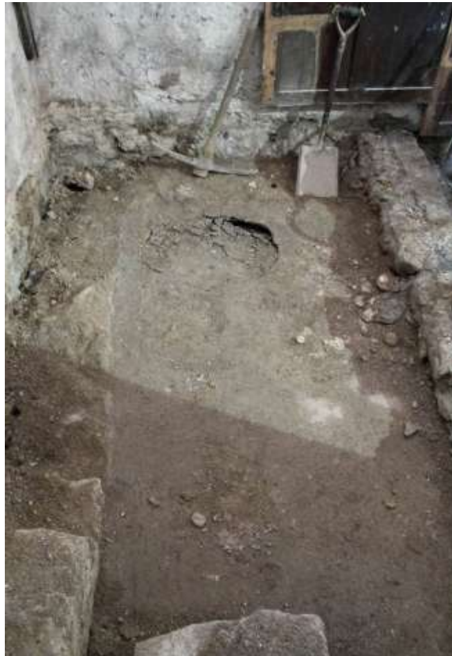
Photo 6: Collapsed area in mortar floor in northwest corner of tower
