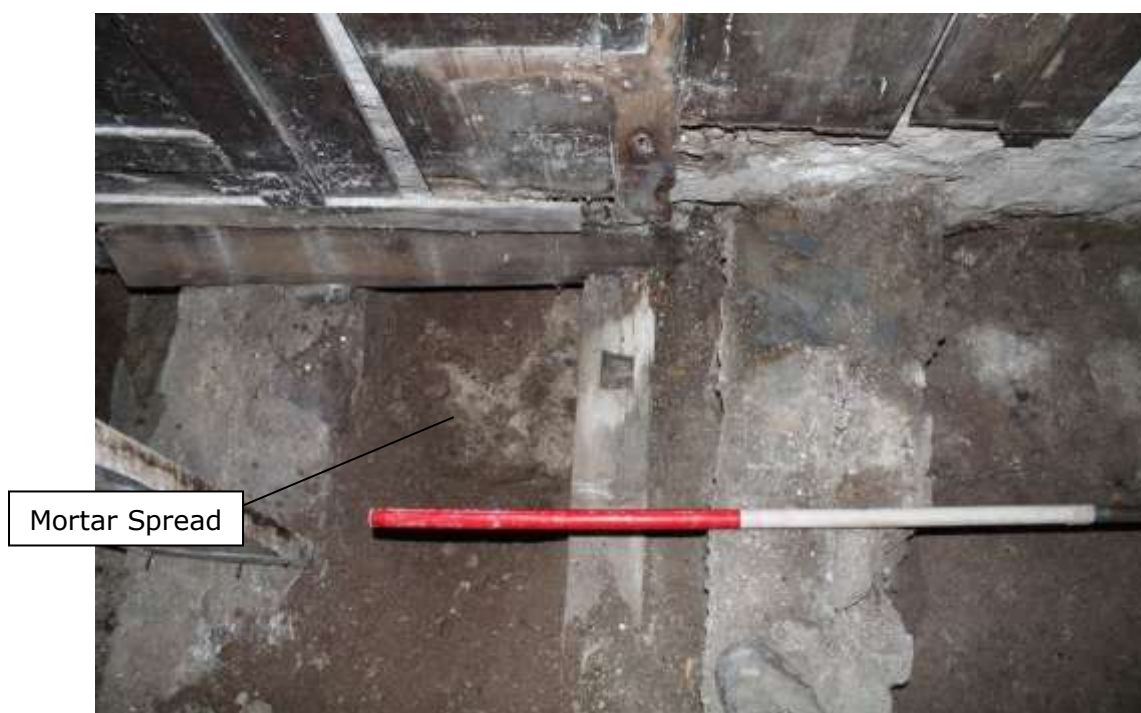
Photo 7: Remains of foundations for southern wall around the inside of the tower, with fragmentary mortar spread to east of sleeper wall (view south)
