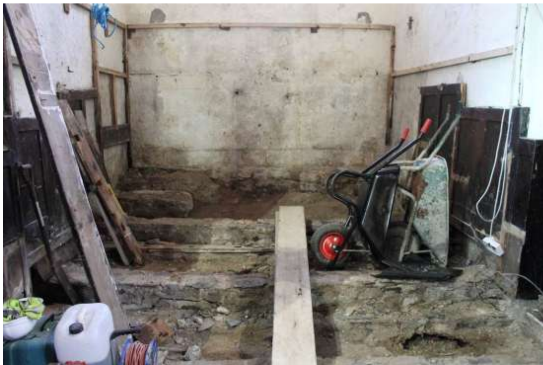
Photo 1: The inside of the West Tower at the start of the works showing the stepped nature of the floor and sleeper walls
