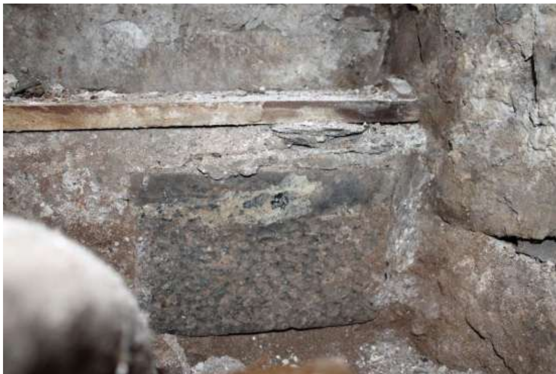
Photo 8: Dressed stone block aligned with northern wall around the inside of the tower, with rough rubble sleeper wall above (view west)
