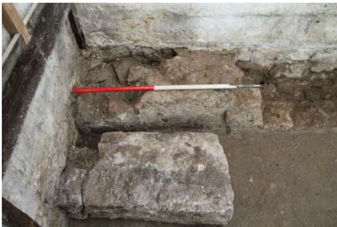
Photo 4: Surviving part of superstructure of western plinth wall and adjacent fragment of loose masonry on mortar floor (view west)
