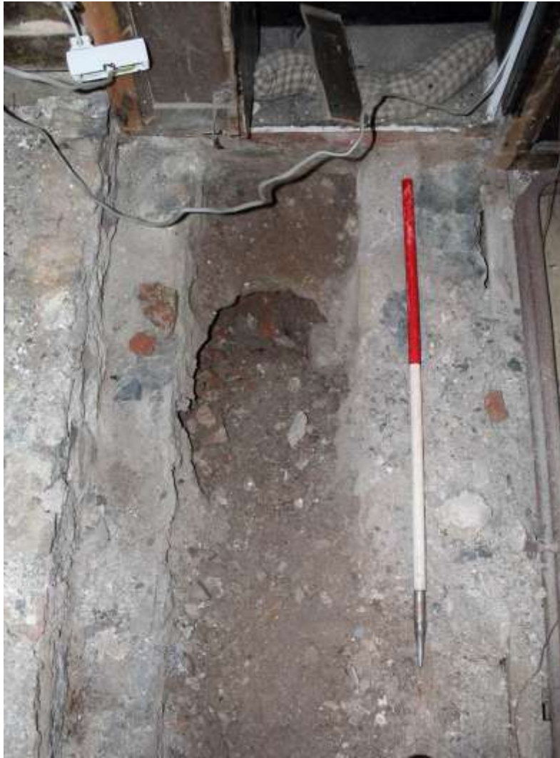
Photo 9: Collapsed area in third step down within church tower adjacent to stair tower doorway (view north)
