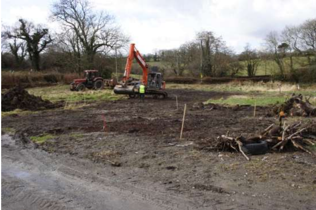
Photo 1: Topsoil stripping of the building footprint facing southwest
