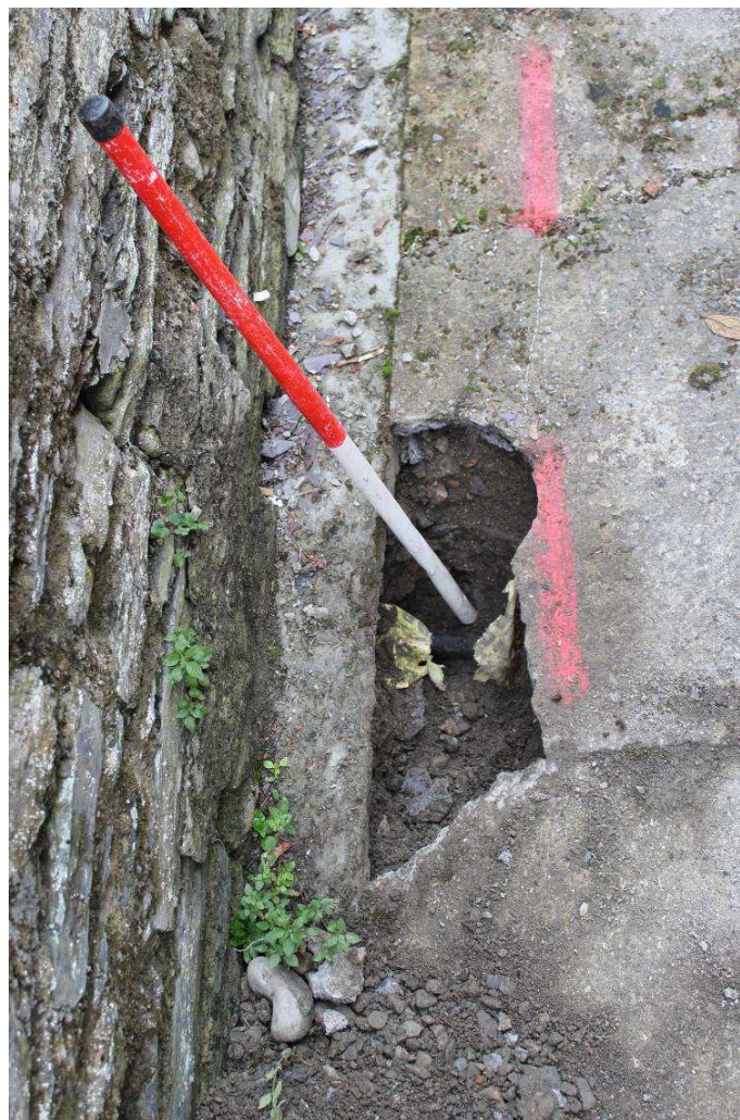
Photo 4: Small excavation to locate services
