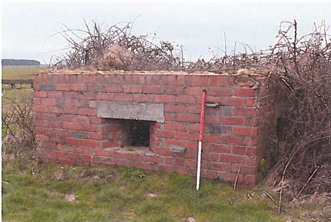
Figure 23: Pillbox on the sea wall at Pembrey, note metal access treads in brickwork
