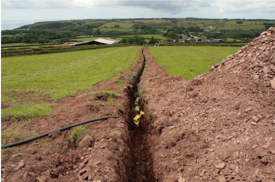
Photo 4: South facing view of excavated cable trench
