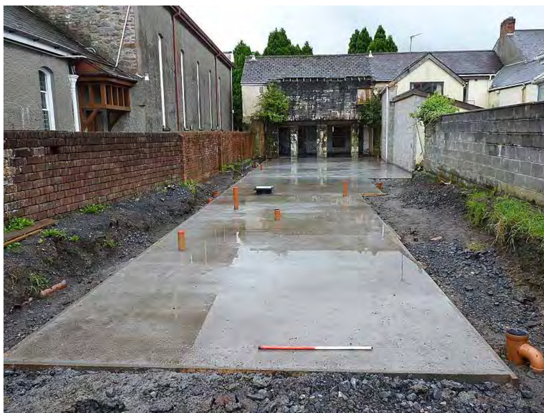
Photo 8: Southeast facing shot of the completed foundation raft to the rear of the street frontage. 1m scale.
