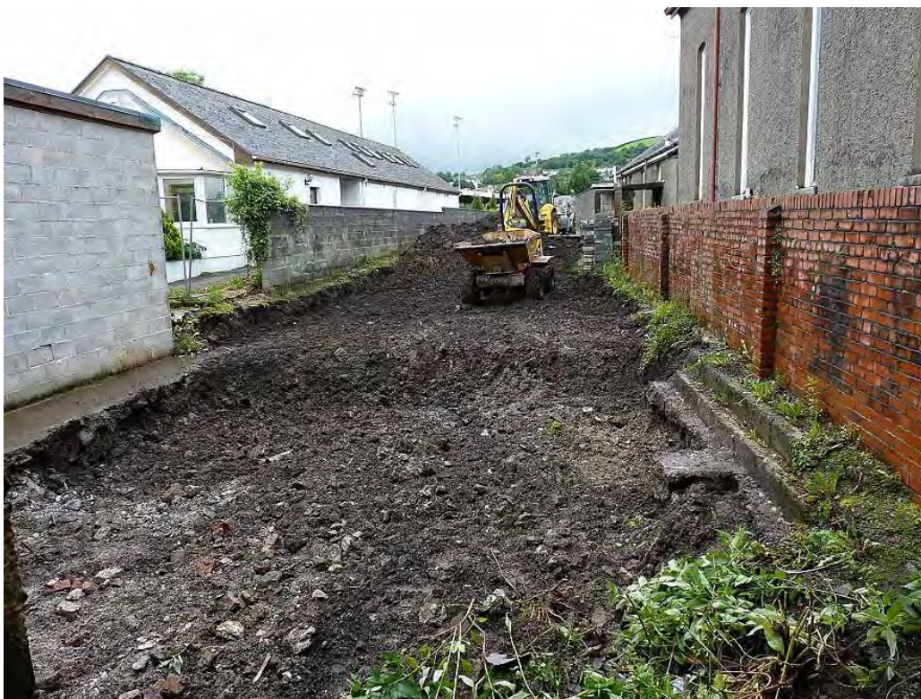
Photo 1: General shot looking northwest during excavation of the foundation raft to the rear of the existing street-front property.
