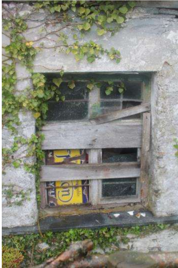
Photo 6. Beneath the modern reinforcements, the original window frame, panes and lead comes are still visible. (Photo: M. Bell).
