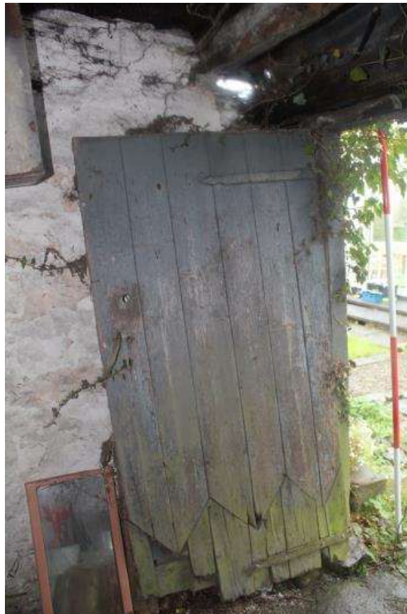
Photo 5. The single plank wooden door. Note the splicing repair work at the bottom of the door and the small hole handle substitute towards to top left of the door. (Photo: M. Bell).
