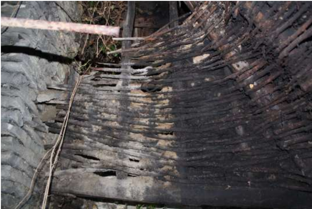
Photo 9. Interior shot of the wattle chimney-hood showing the soot blackened larch wattle. Note the absence of daub on the interior of the hood (Photo: M Bell).
