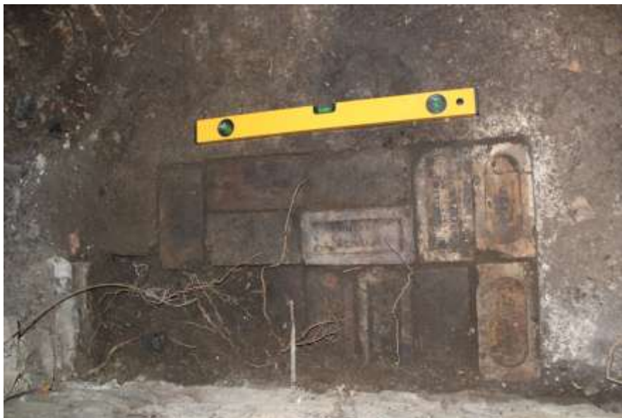
Photo 8. The frogged fire bricks in the hearth. (Photo: M Bell).
