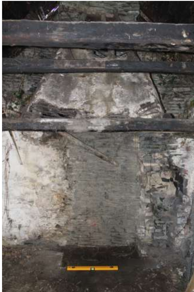
Photo 7. The brick lined hearth visible beneath the larch wattle chimney-hood resting on the cross beam. Note the daub on the exterior of the hood. (Photo: M Bell).
