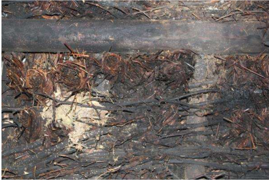
Photo 4. Knotted bunches of straw indicate a thrust thatching technique. The wattle woven larch foundation layer provides a convenient home for a swallow's nest! (Photo: M.Bell).
