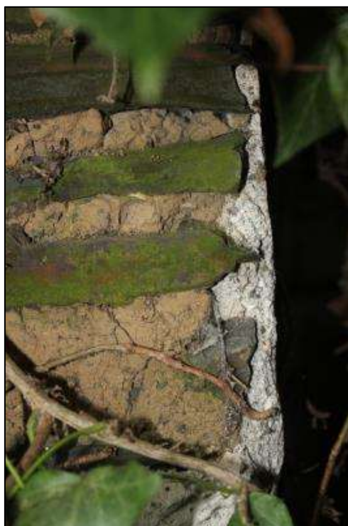
Photo 3. Viewed in cross-section; this image shows the rubble shale walling, clay/mud bonding and lime plaster or rendering (Photo; M.Bell).
