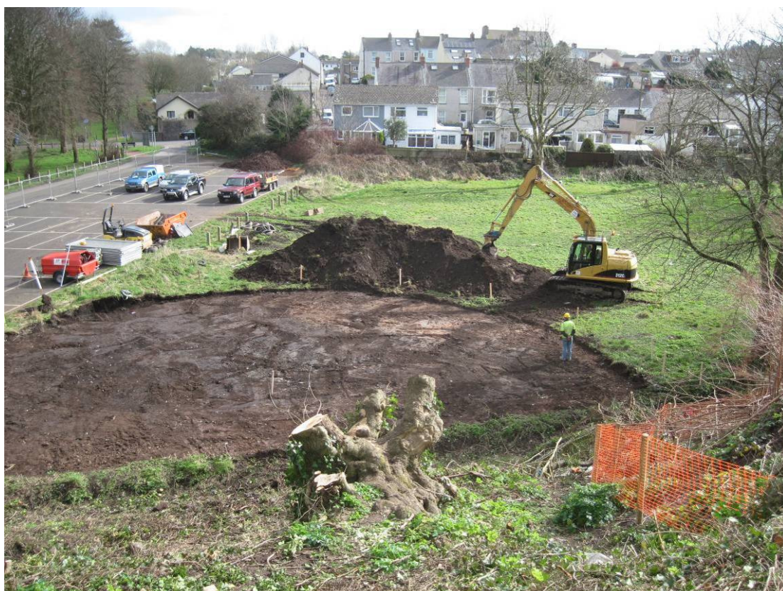
Photo 1: Overview of the topsoil stripped area of the lower part of the Pembroke Cycle Way scheme. View east from the higher part of the site.
