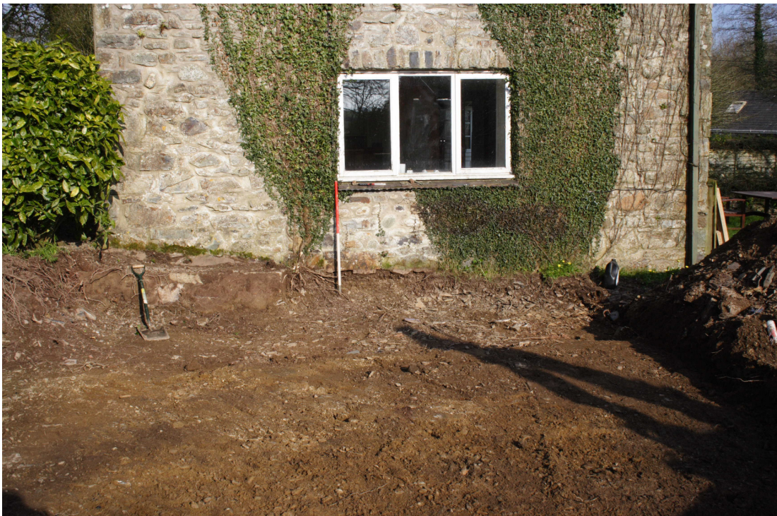
Photo 6: View towards western gable end wall of Ivy Court Cottages showing insubstantial footings on 'rab' bedrock
