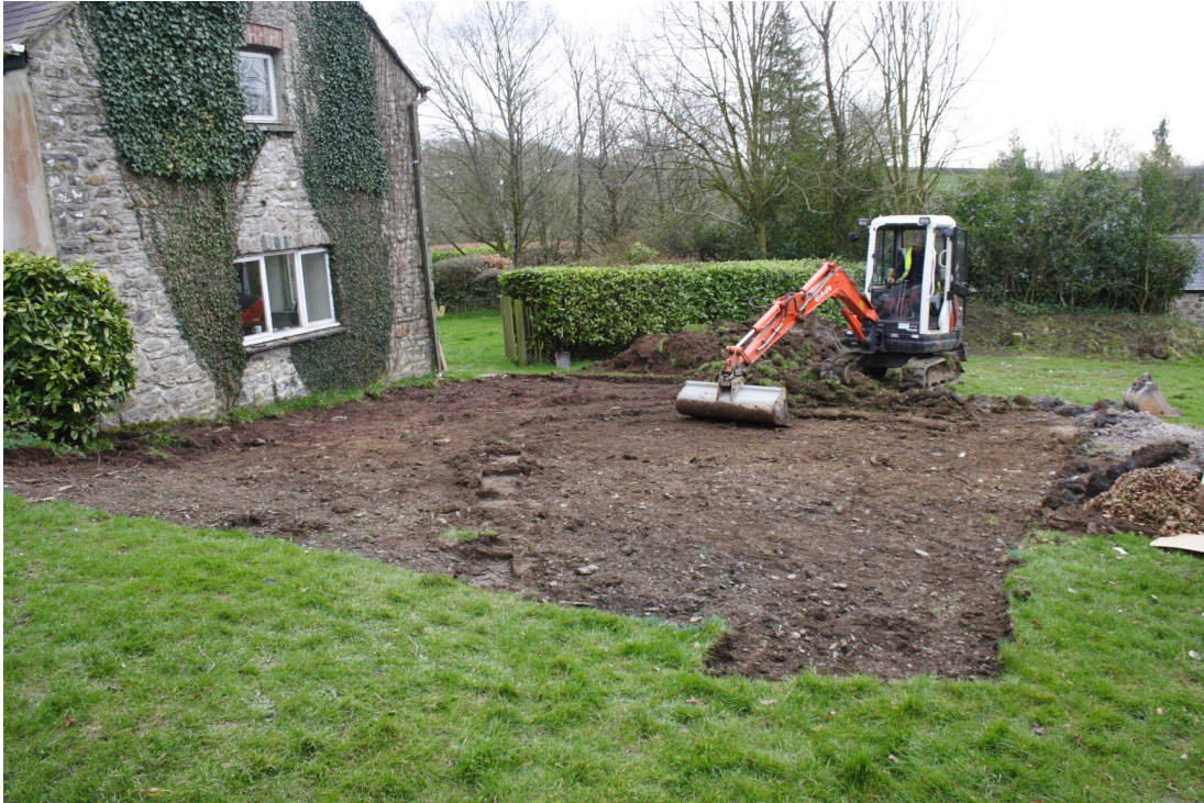
Photo 2: Topsoil stripping of the site area showing line of impressions of concrete flag stones in the excavated surface
