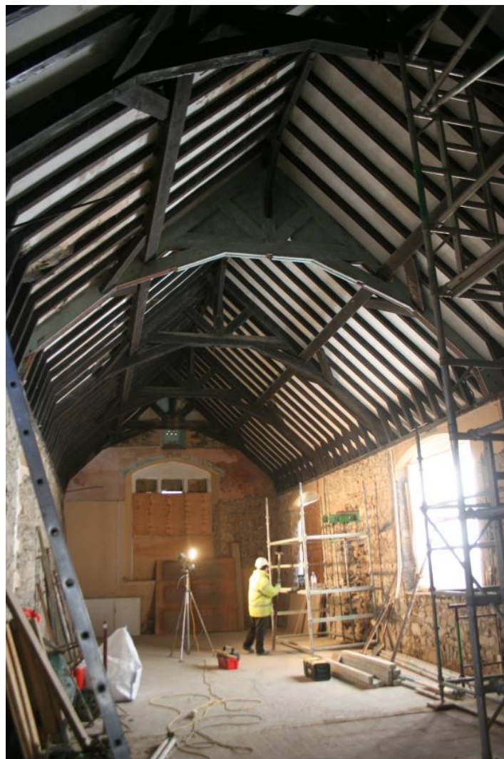
Photo 12: View south; king-post trusses in roof structure.
