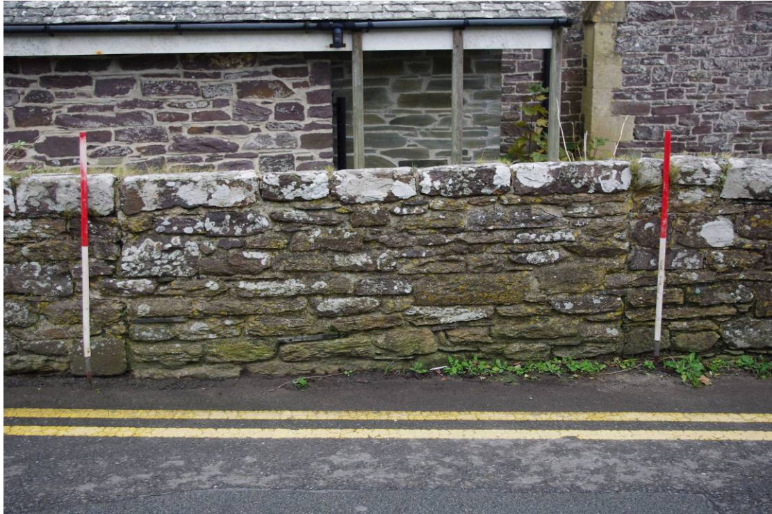
Photo 4: Straight joints seen in wall at southern end of original school building, viewing west (image number 136)
