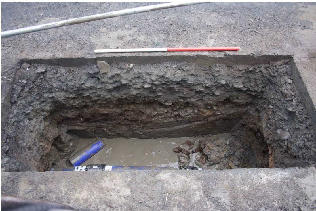
Photo 2: North facing representative section showing road formation layers overlying clays (Area 1)
