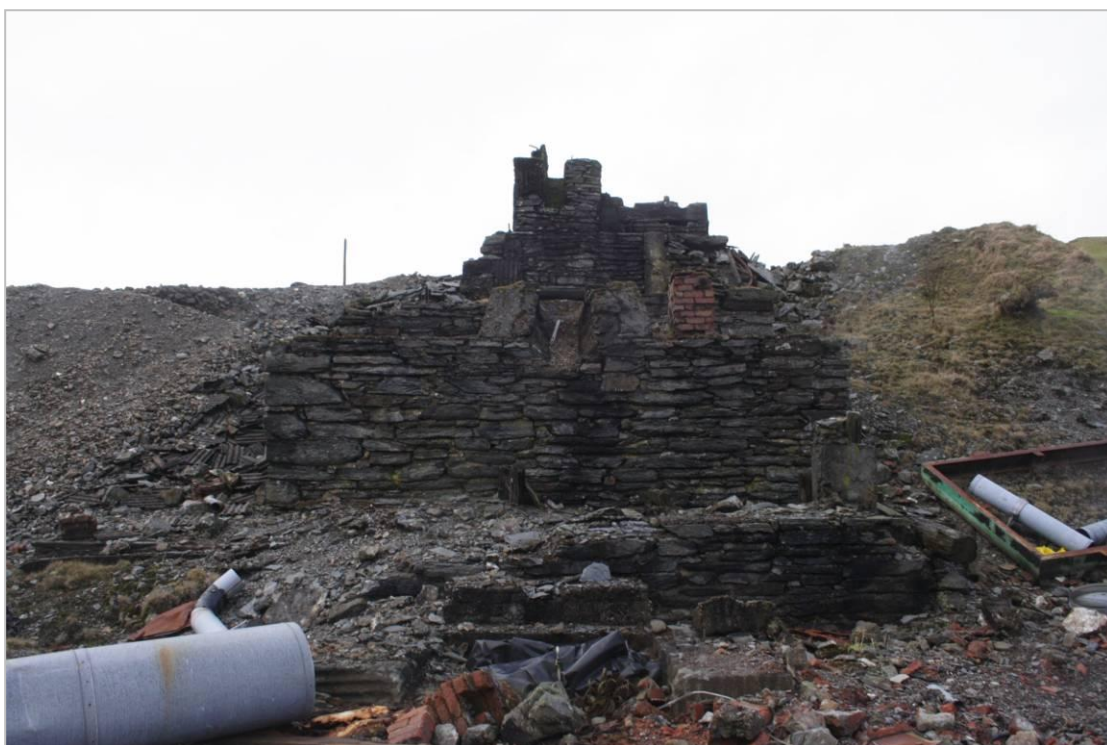
Photo 10: View of red brick and rubble walling supporting loadings on site of head of incline. Looking approximately north.
