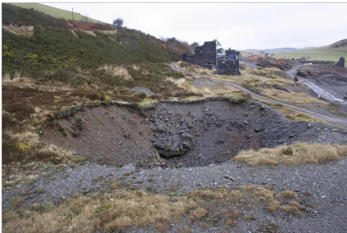
Photo 3: View of subsidence around Williams Shaft that has occurred since last recorded in 1993. Looking north-east.
