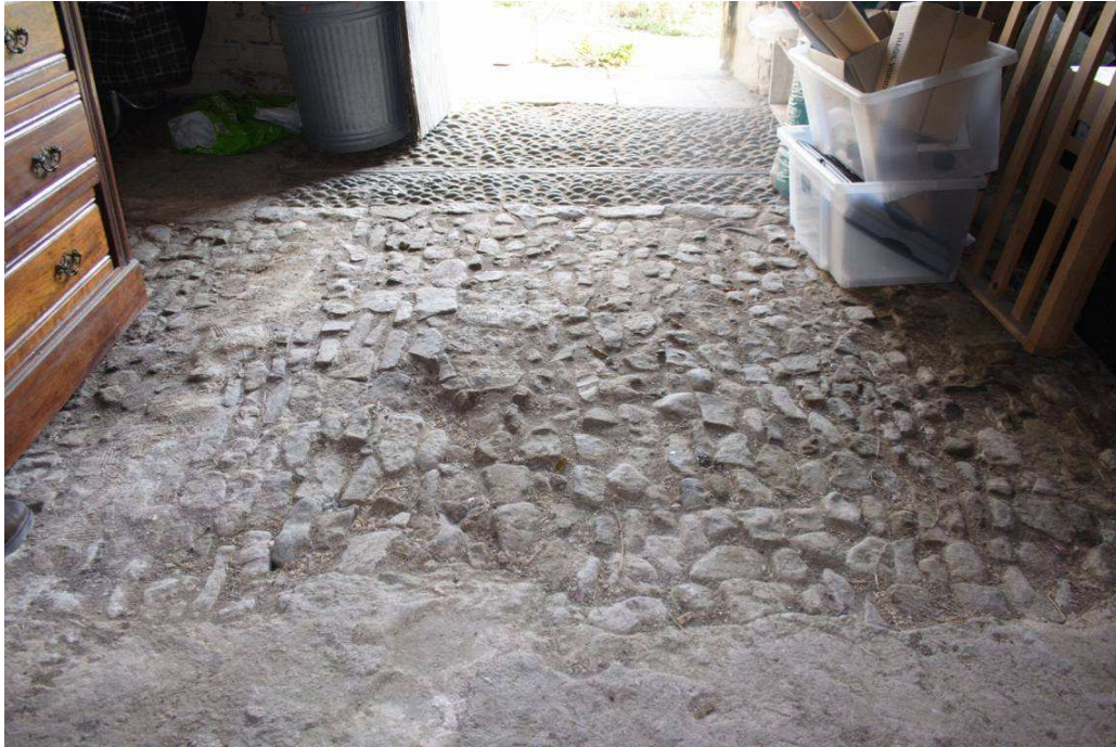
Photo 5: Stable floor - stall platform, gutter and river worn cobbles
