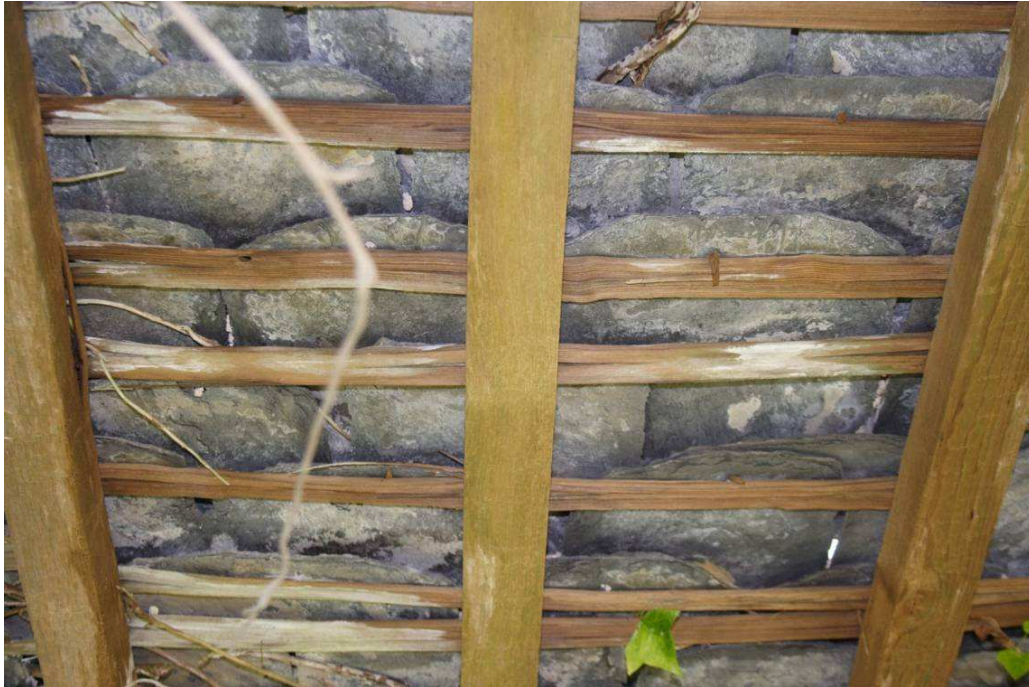
Photo 13: Feed preparation room interior -peg hung slates on split oak battens
