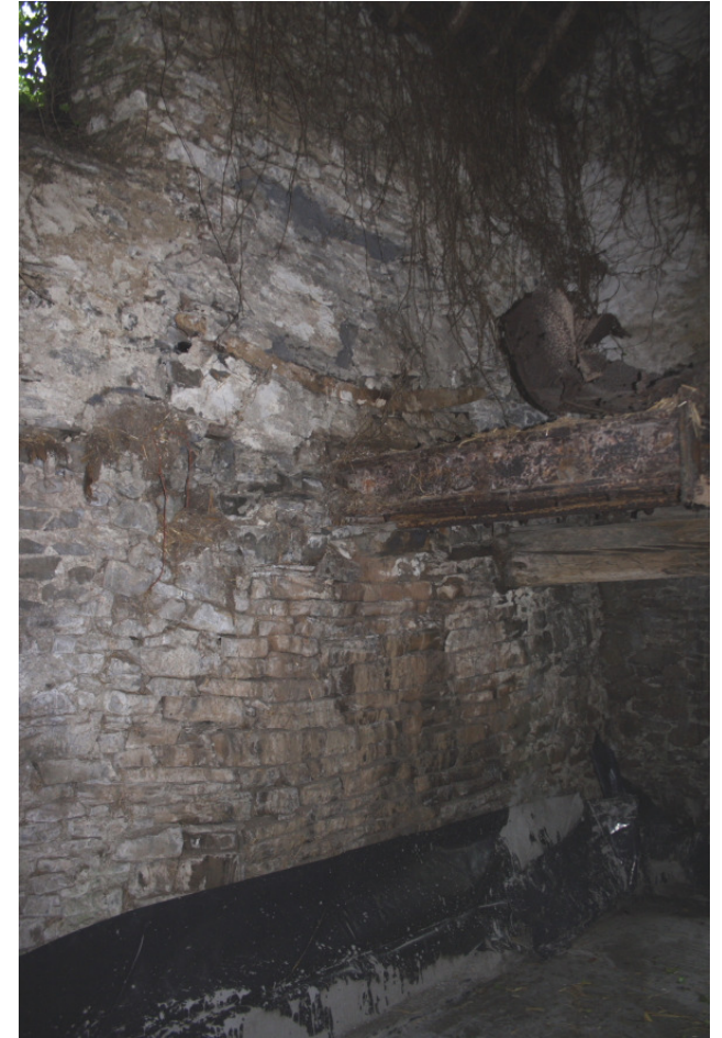
Photo 13: North wall of mill building showing metal inlet from mill pond
