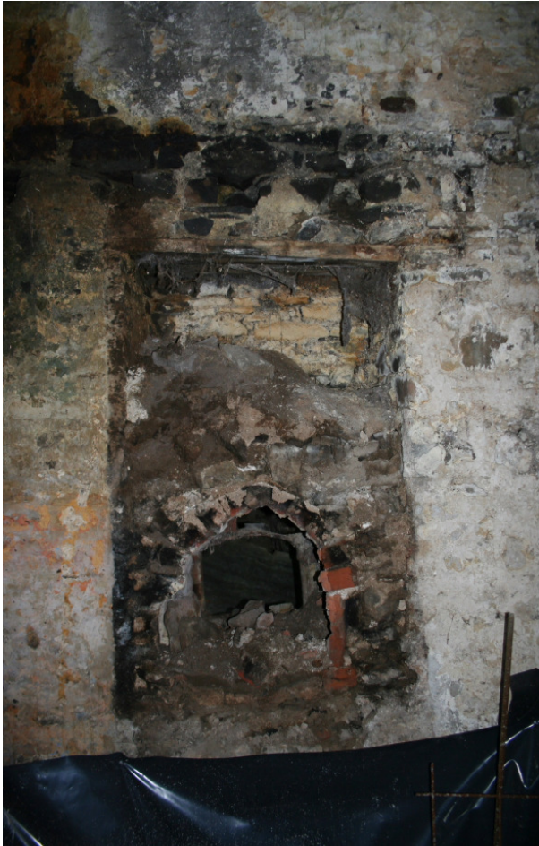
Photo 11: Bread oven in south wall of mill building
