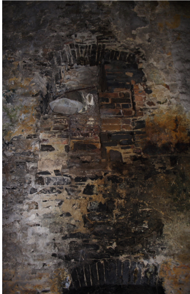
Photo 12: Former fireplaces in south wall of mill building (ground and first floors)
