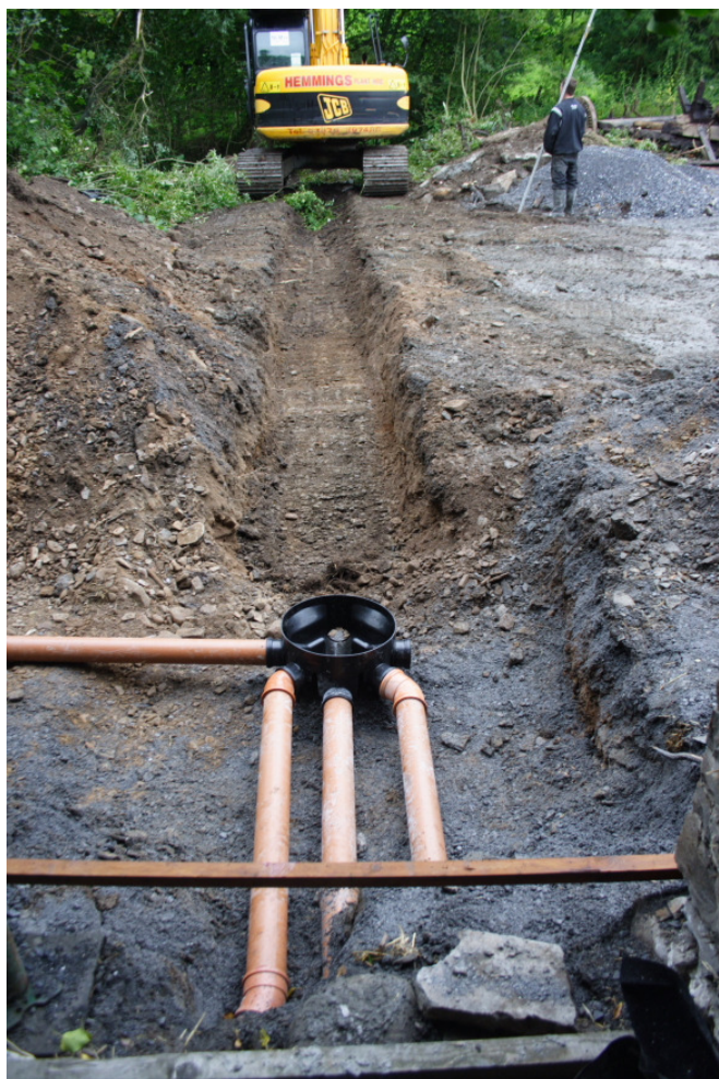
Photo 1: Excavation for drains from mill to stream
