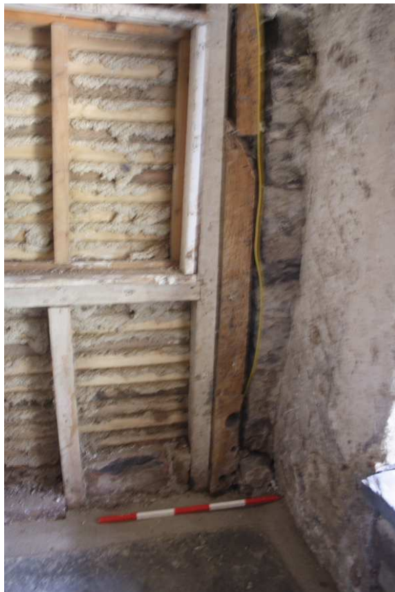
Photo 26: Stairwell looking south (note straight joint to right)
