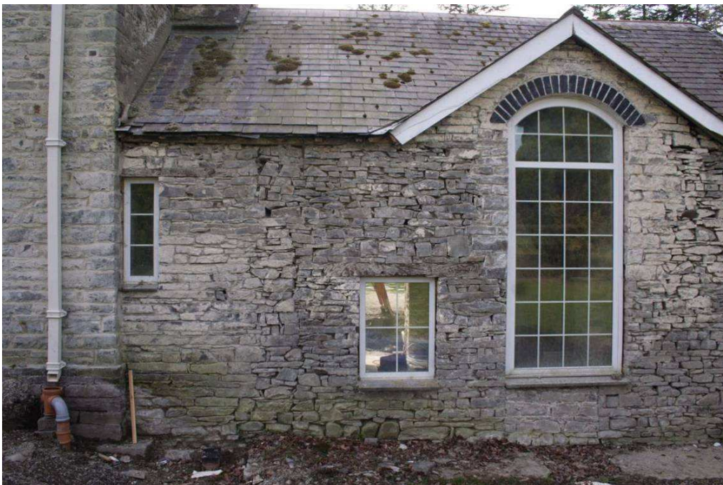
Photo 4: The north end east facing elevation (note differences in stonework and window heights)
