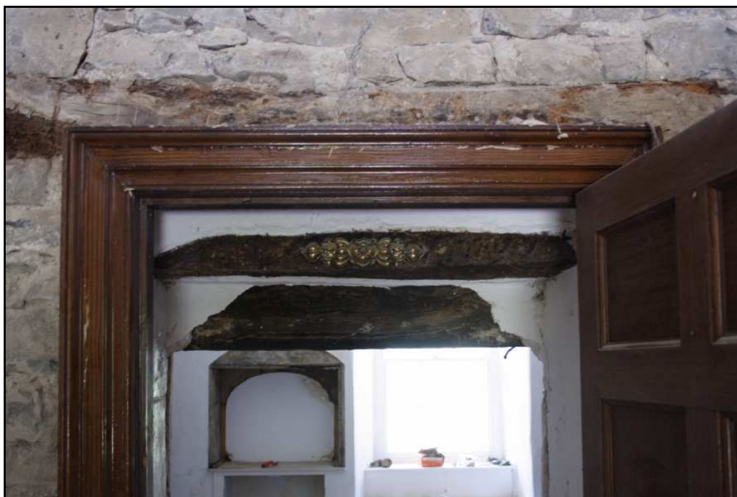
Photo 21: Three door lintels in doorway between dining room and former kitchen (equating to three phases of building?)
