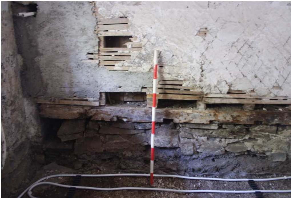
Photo 25: Lath and plaster stairwell division utilising re-used timber (note straight joint to left). Looking north.
