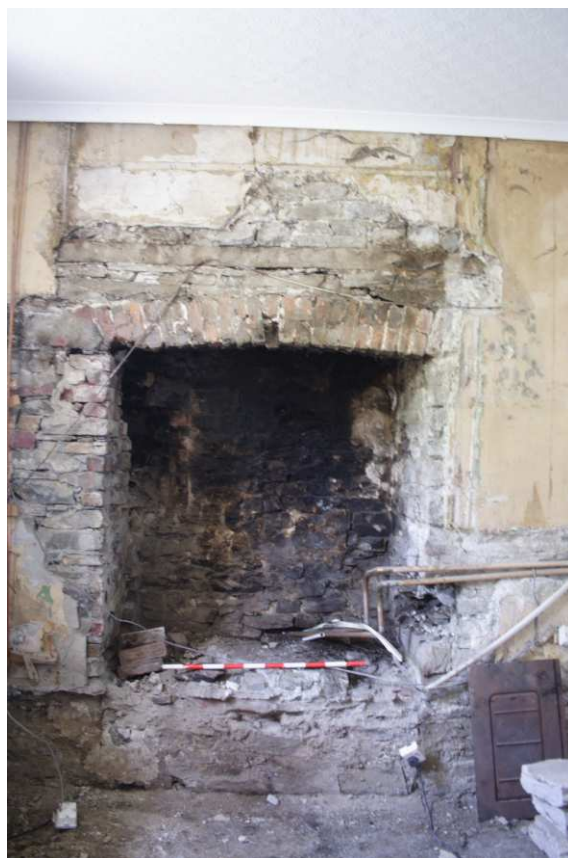
Photo 19: Fireplace on former kitchen (floor levels reduced)
