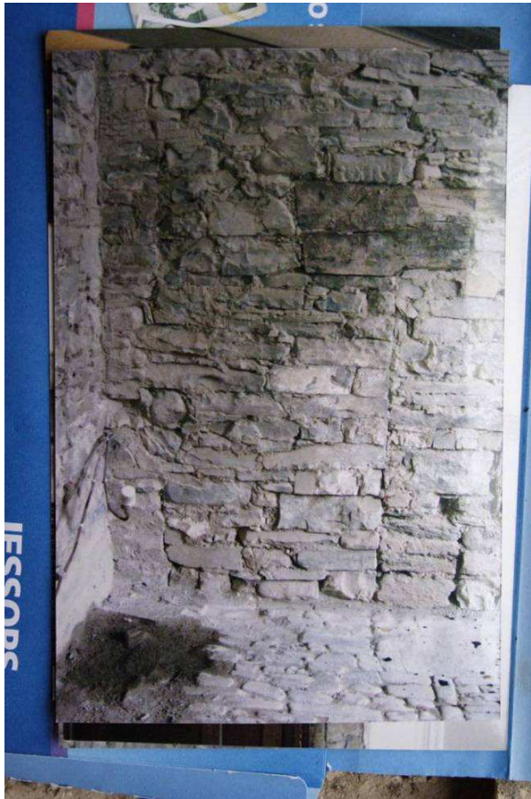
Photo 29: Cobbles in dining room (note hearth stone, blocked fireplace, straight joint to left and missing cobbles against wall)
