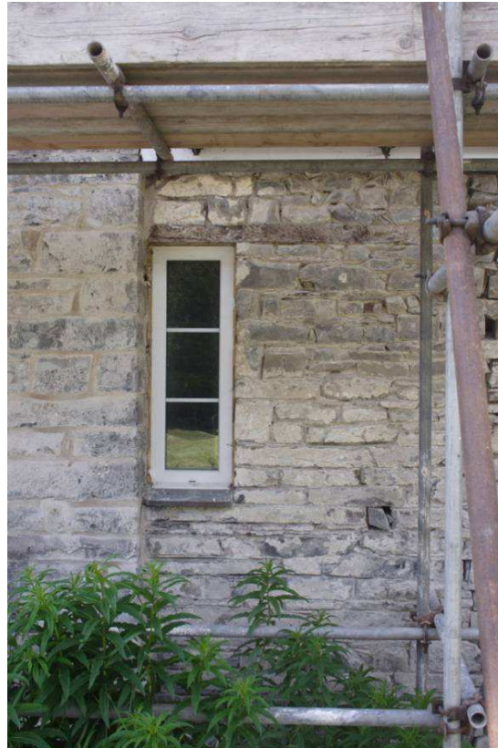
Photo 8: Possible truncated window (in location of former doorway?)
