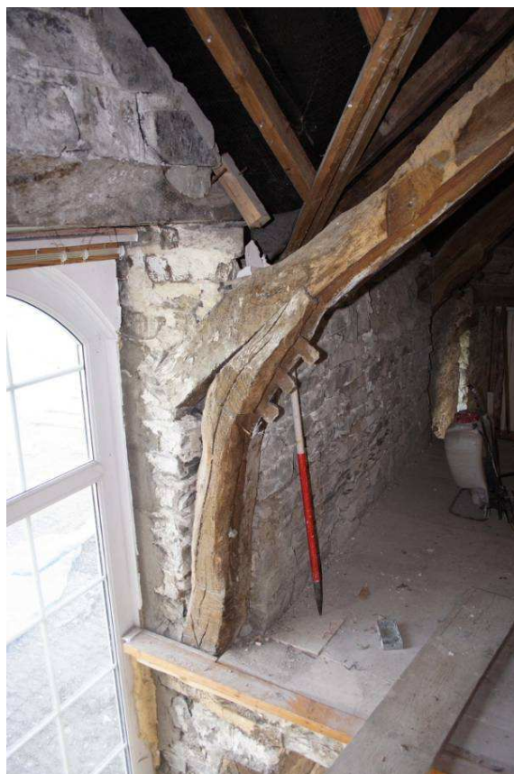
Photo 16: Detail of pegged scarfed cruck
