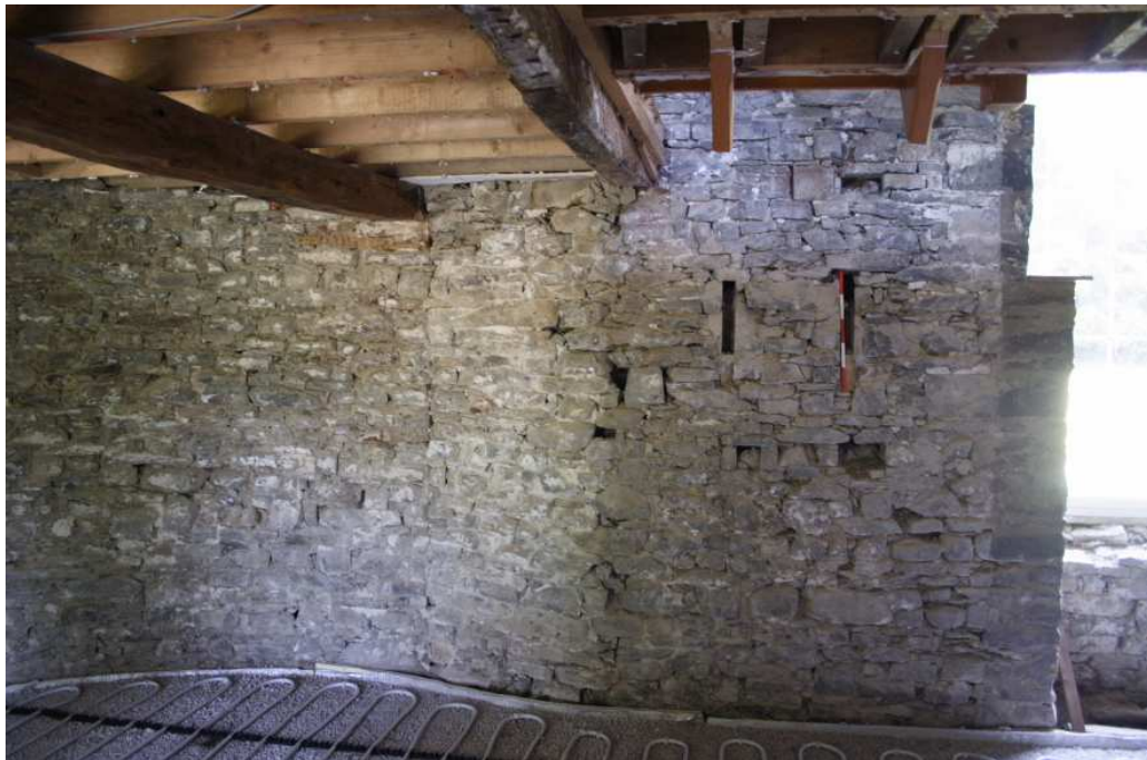
Photo 18: Interior east wall of northern annexe showing recesses in wall and joint to apsidal end
