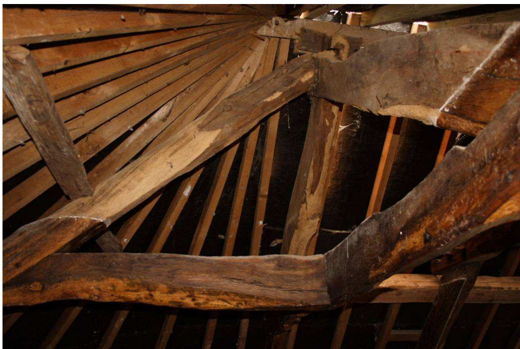
Photo 15: Detail of roof timbers at apsidal end (partially repaired)
