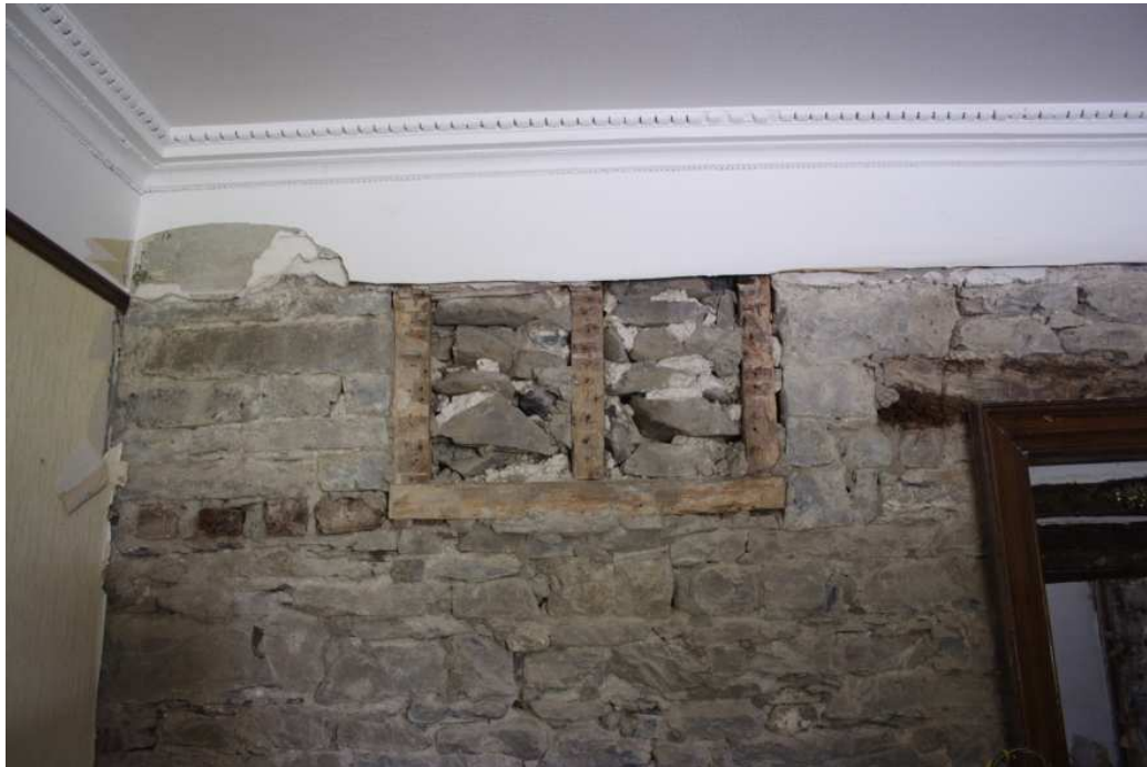
Photo 23: Blocked opening in west wall of dining room (note height in relation to door lintels).
