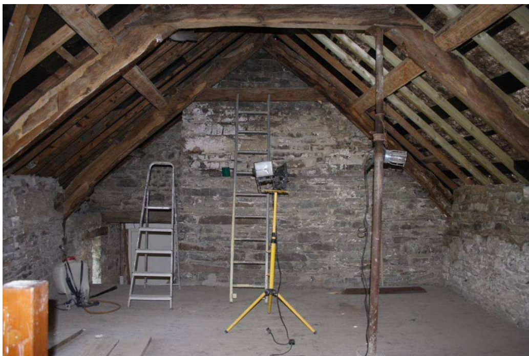
Photo 13: Roof timbers and back-to-back chimney stack. Facing south.
