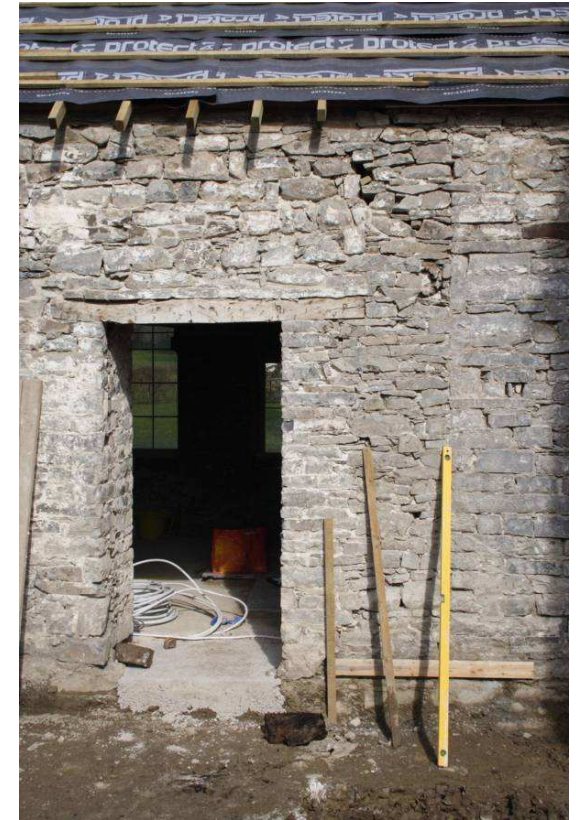
Photo 9: Doorway in west wall of northern annexe (note straight joint with chimneystack)
