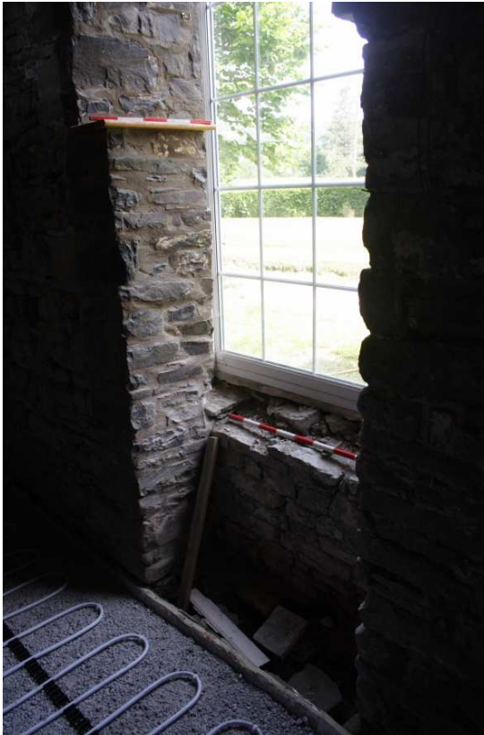
Photo 10: Interior view of arched window opening with 50cm scale resting on location of earlier doorway lintel.
