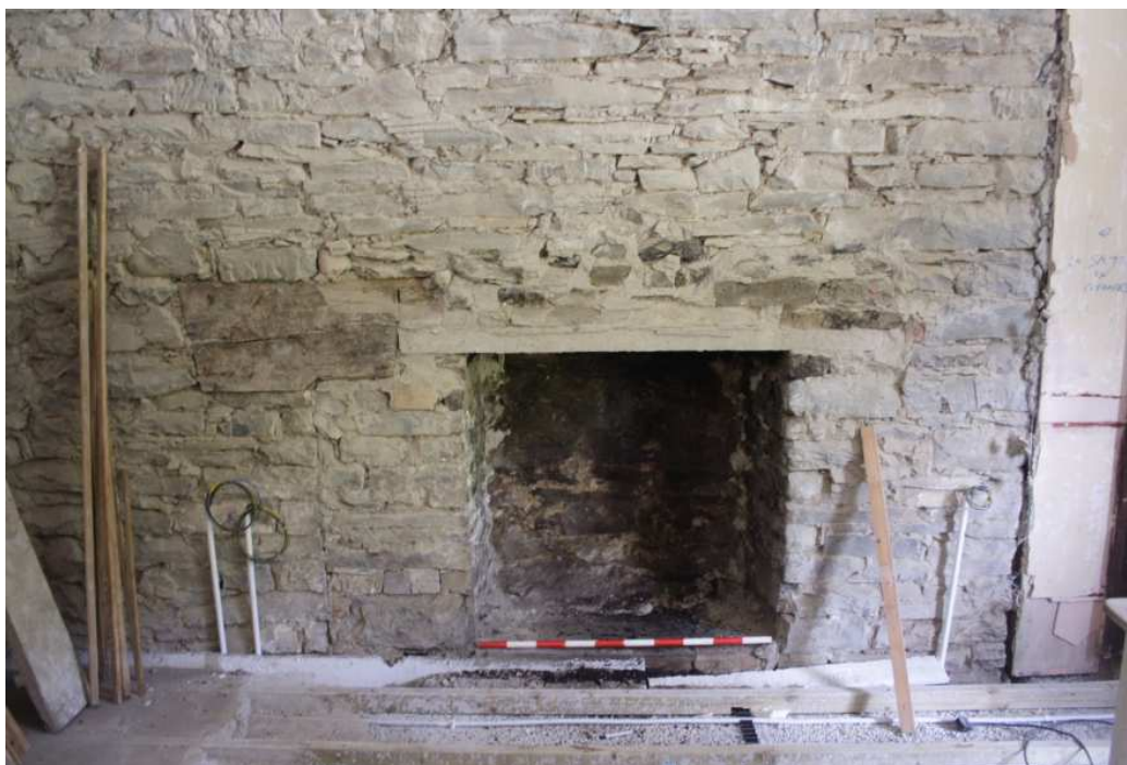
Photo 22: South side of back-to-back fireplace showing truncated bressumer beam and later inserted hearth.
