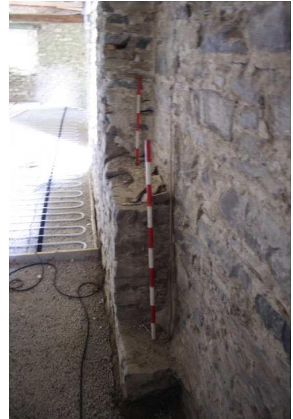
Photo 12: Interior view of interface between early and later walls of east face of northern annexe showing stepped later wall.
