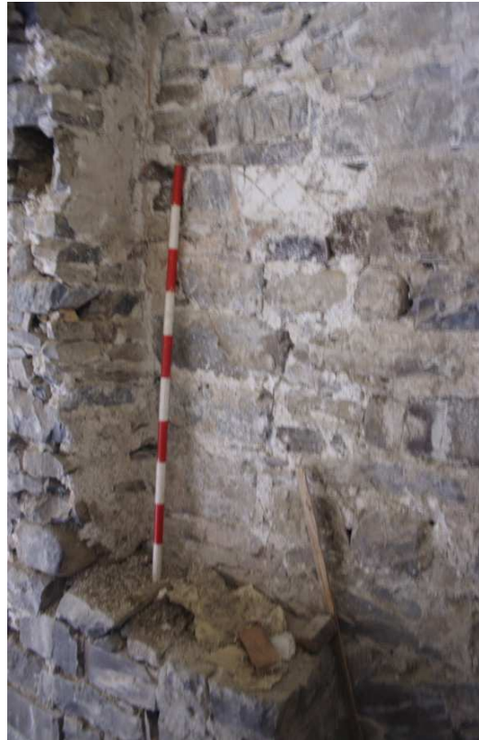
Photo 11: Interior view of interface between early and later walls of east face of northern annexe showing irregular joint in stonework.
