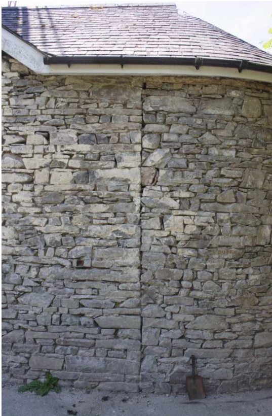
Photo 7: Straight joint between northern annexe and the apsidal end
