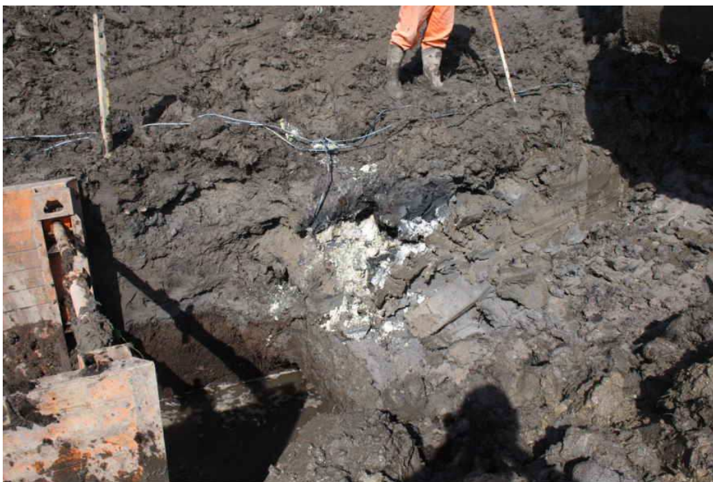
Photo 10: Degraded heavy duty battery and electrical cabling
