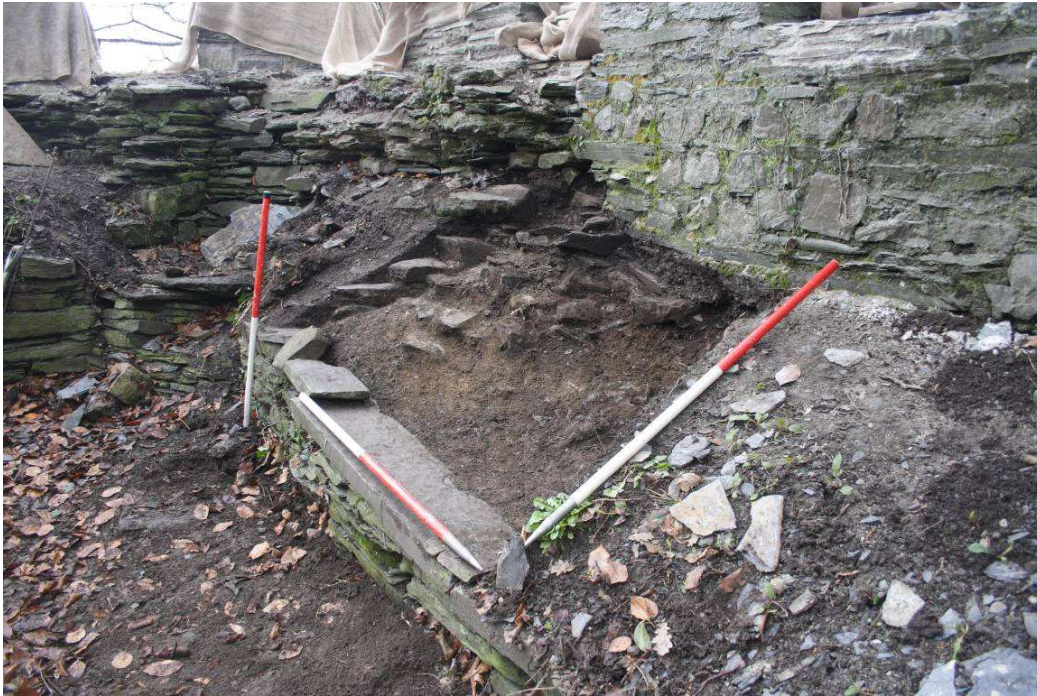
Photo 45: Southeastern side of tower, showing small retaining wall, embanked garden soil and area of rubble core, 1m scales
