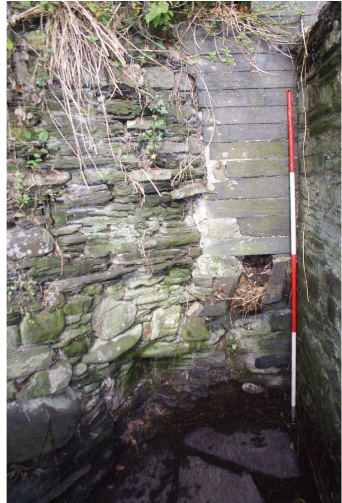
Photo 29: Stone channel through end wall in northern corner of Room 4, 2m scale
