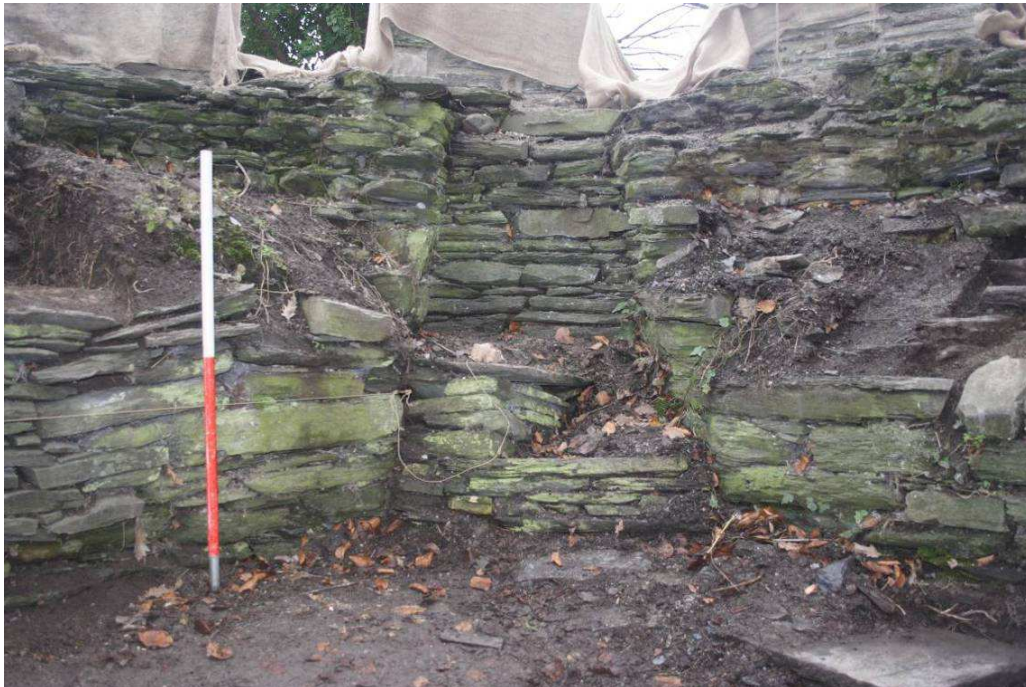
Photo 46: Southern corner of tower, showing thickness of walling, and tapering recess with stepped stone infill
