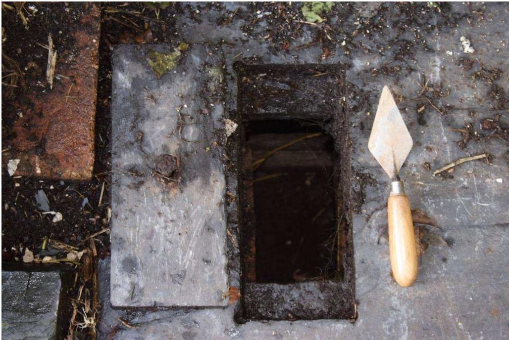
Photo 34: Small slate drain access cover (with 4" pointing trowel)
