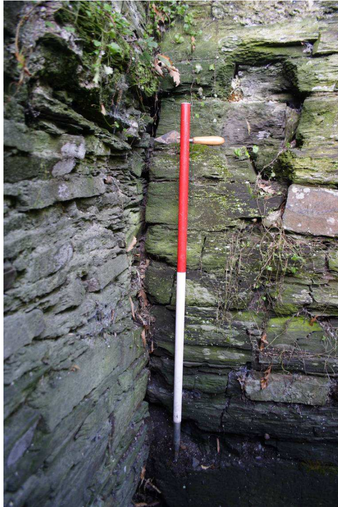
Photo 13: Detail of North east bastion Wall (facing) and the northeastern end wall of Room 1 butting against it, 1m scale
