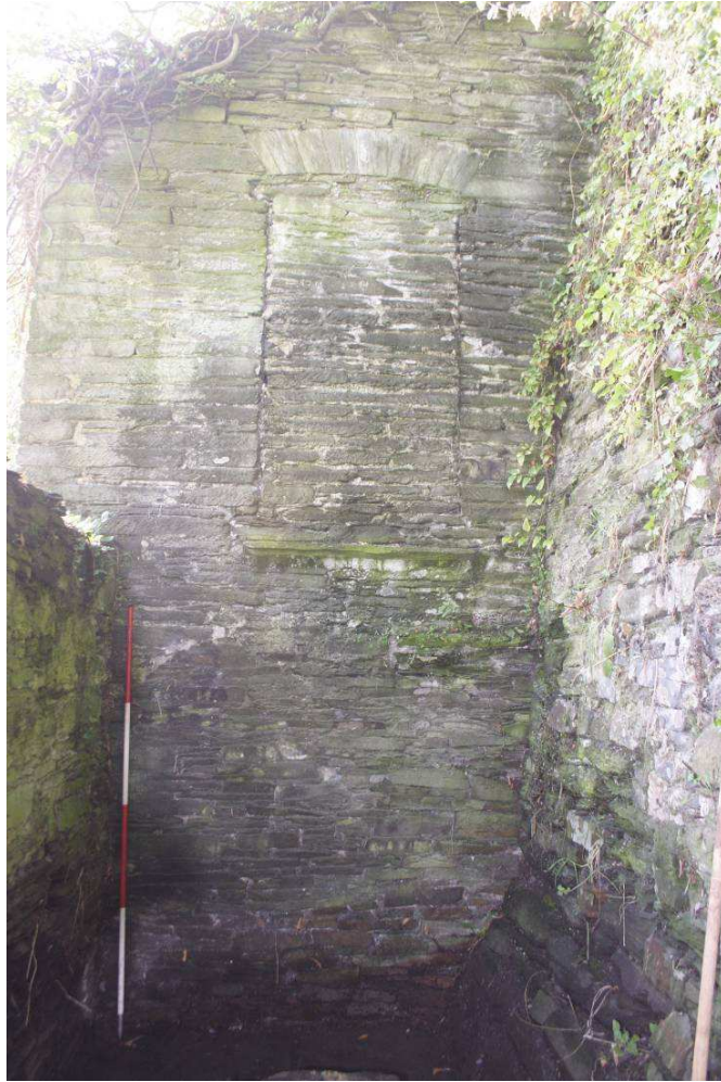
Photo 27: Southwestern wall of Room 4 with blocked doorway at first floor level leading from building of Room 1, 2m scale
