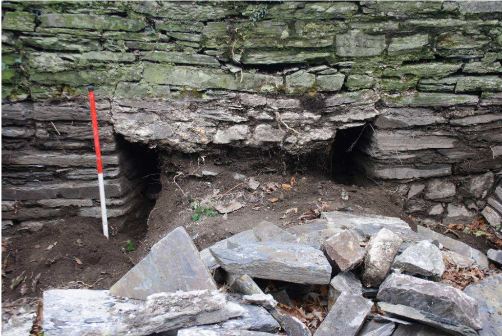
Photo 41: Alcove on inside of North East Bastion wall following removal part of infill prior to rebuild, 1m scale
