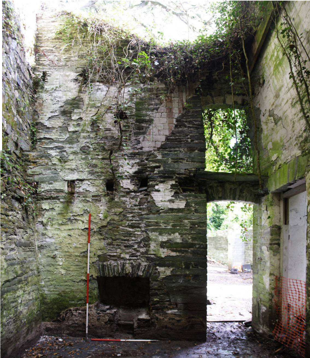
Photo 25: Southwest facing internal elevation of Room 3, showing the adapted end wall of Room 2, and that of Room 5 to the right, 2m and 1m scale
