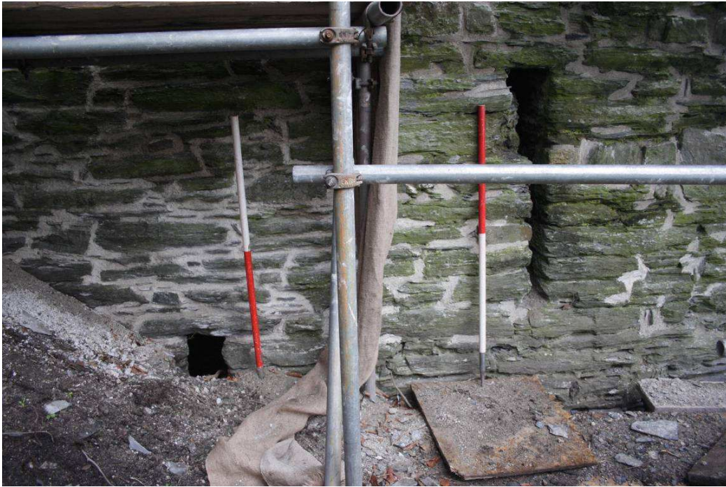
Photo 55: Arrow slit in southwest wall of tower, and lower light to northwest for stairs through wall, 1m scales
