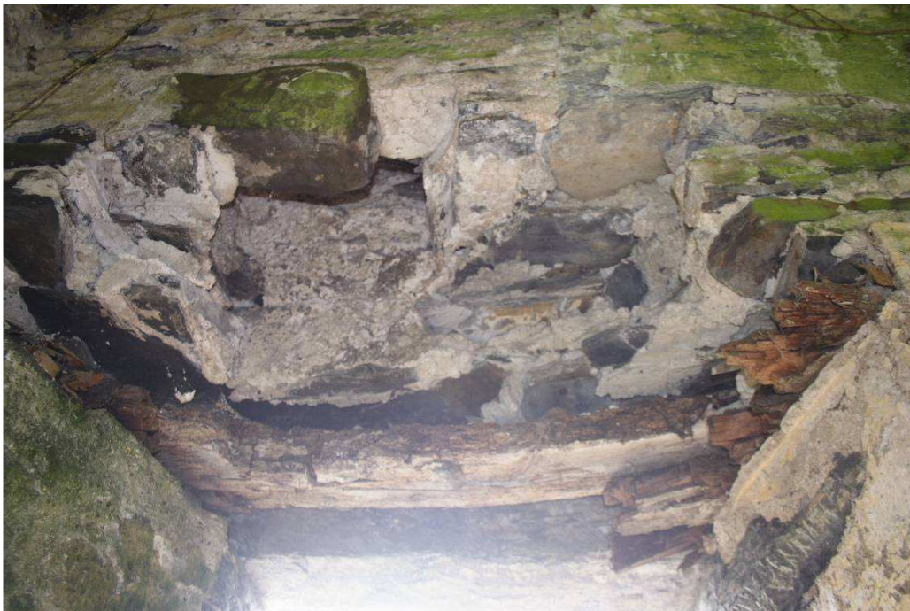
Photo 19: Blocked flue of chimney above decayed wooden lintel
