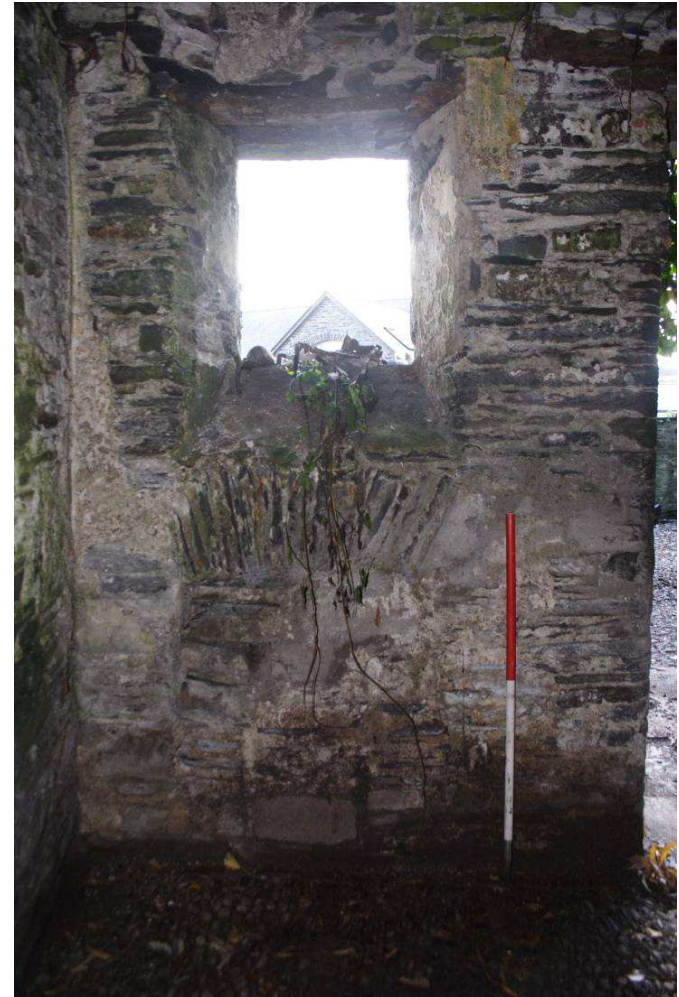
Photo 17: Internal view of window and earlier fireplace, 1m scale
