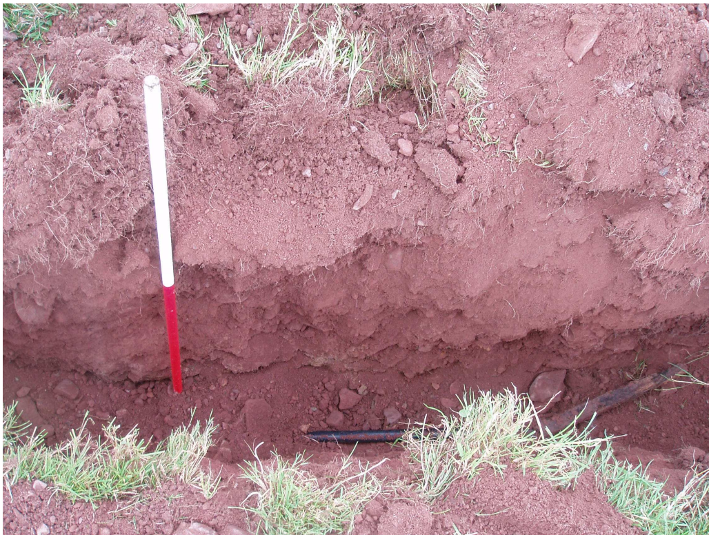
Photo 4: Representative section of cable trench.
