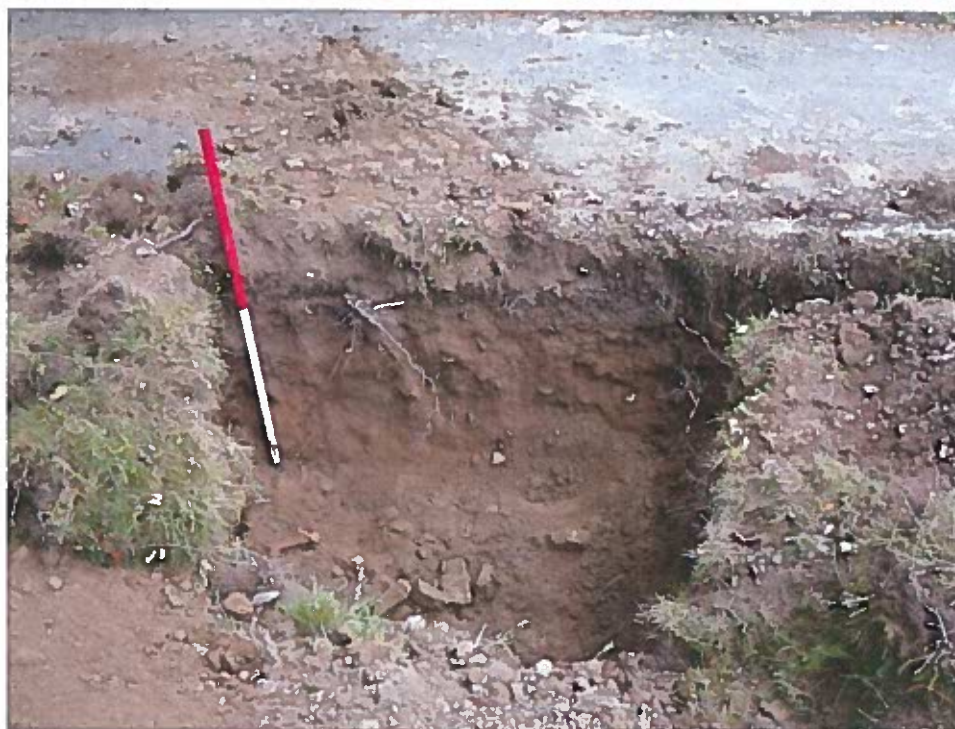
Photo 5: Soakaway on south side of path
