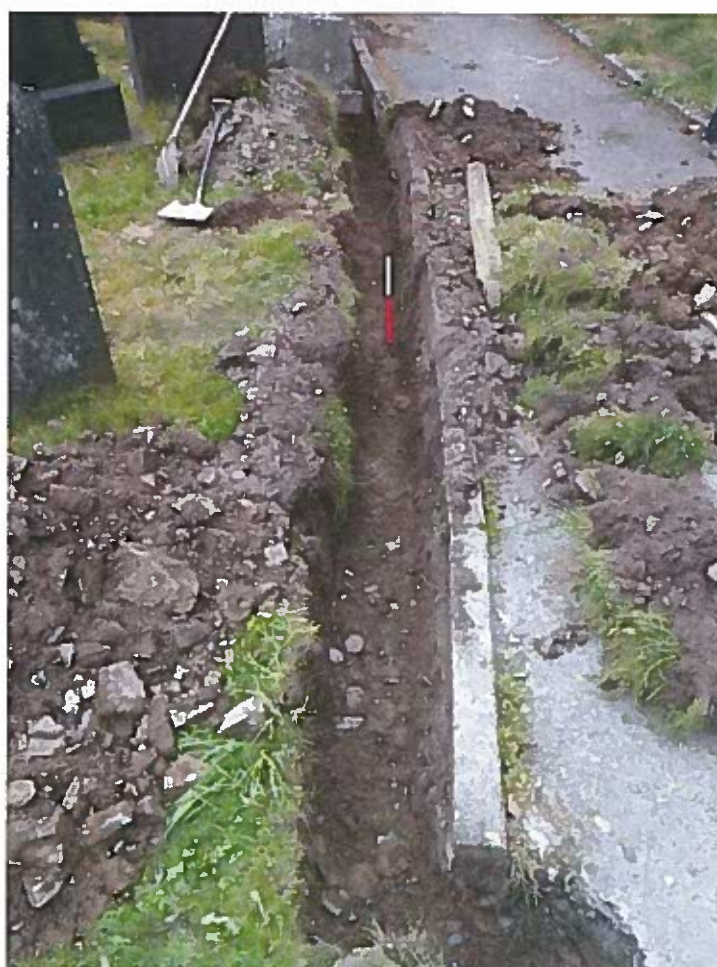
Photo 4: Drainage trench along south edge of path
