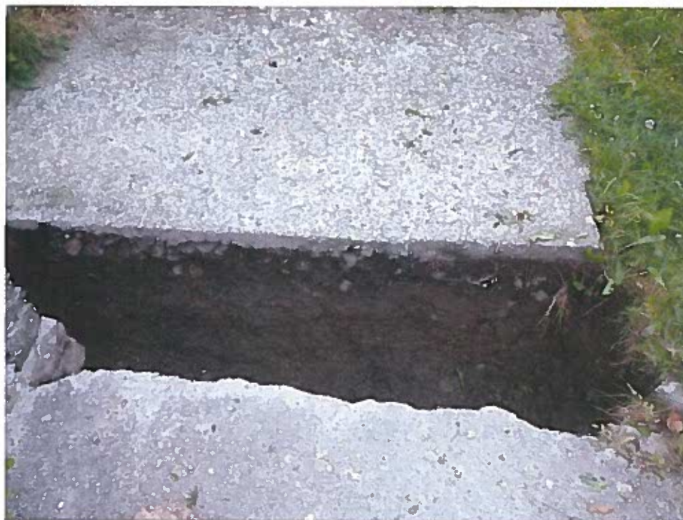
Photo 3: Drainage trench at southwest corner of the church
