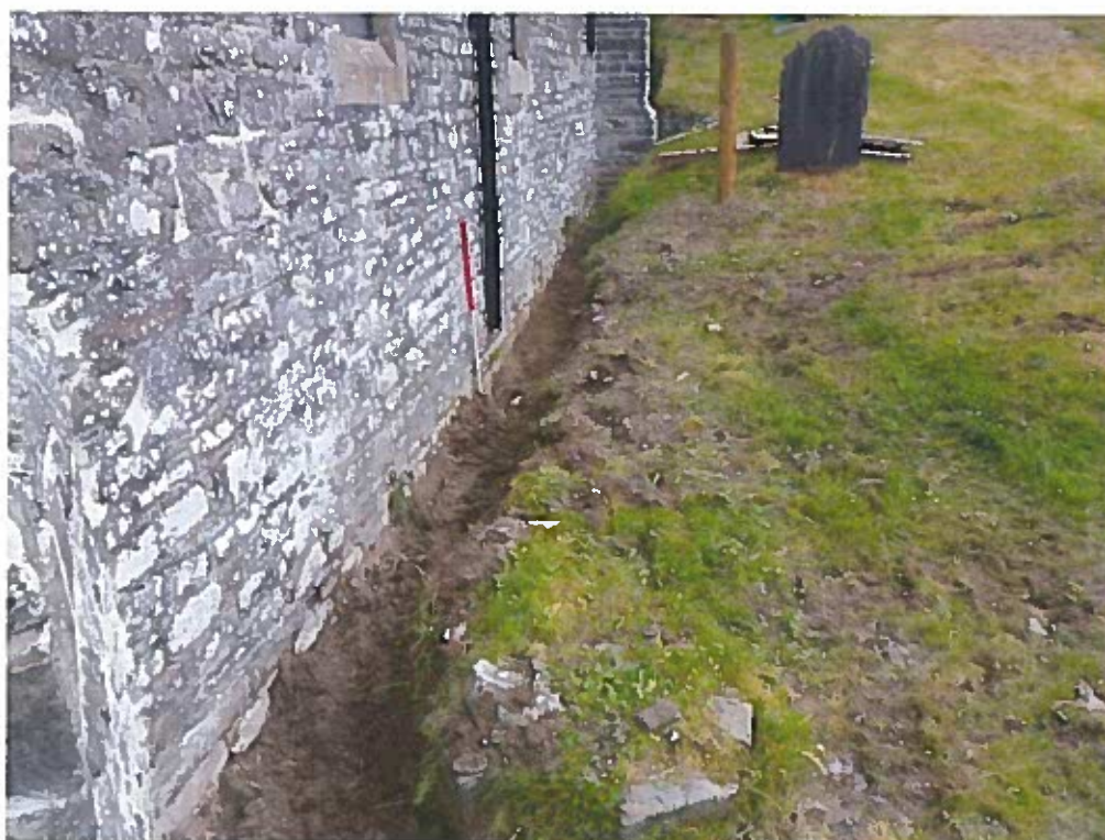
Photo 2: Drainage trench along base of south wall
