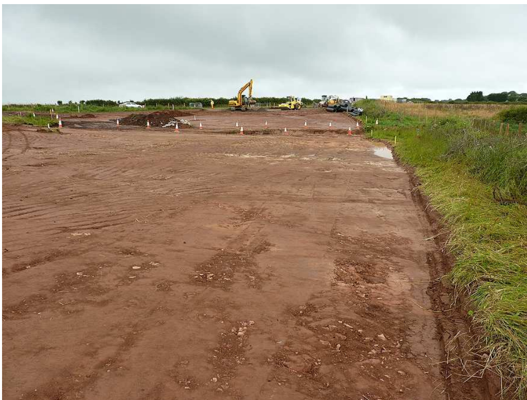
Photo 17: Looking SW at palaeochannel 112 after rolling, still visible as a darker strip that is gathering water
