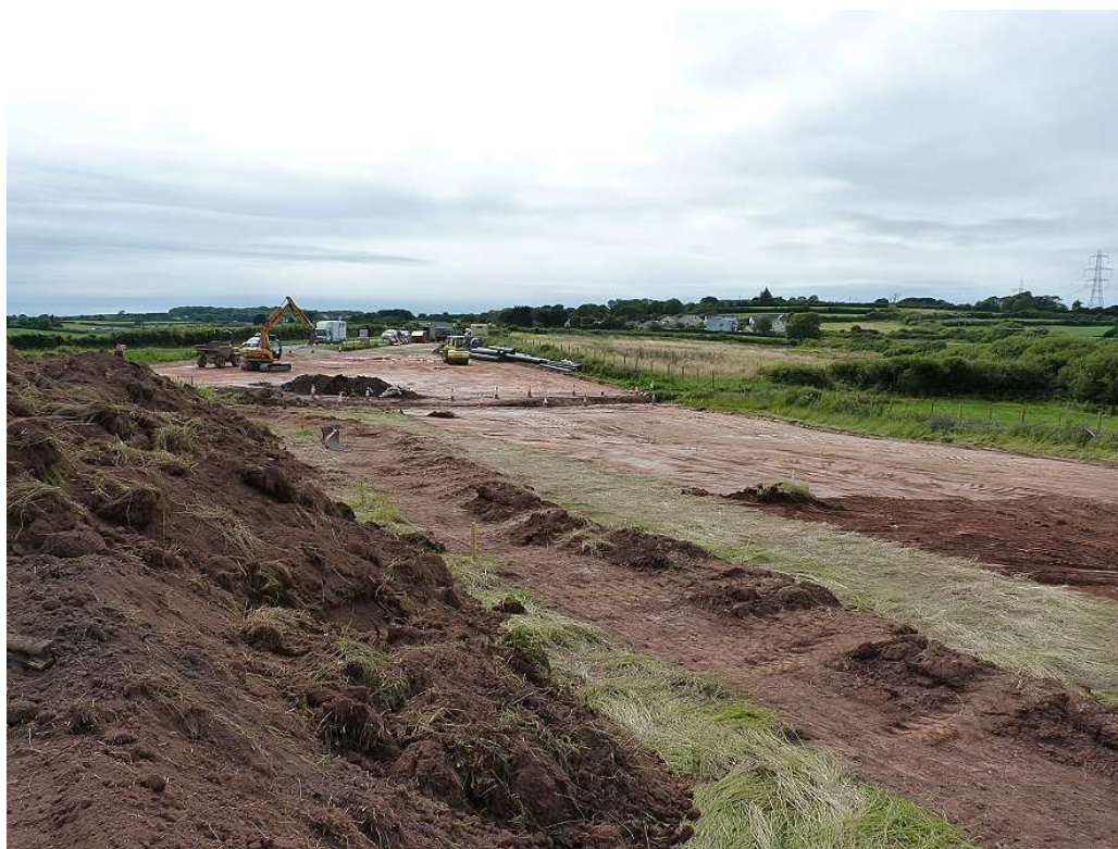
Photo 4: Looking WSW across site during topsoil strip, onsite spoil heap shown on left
