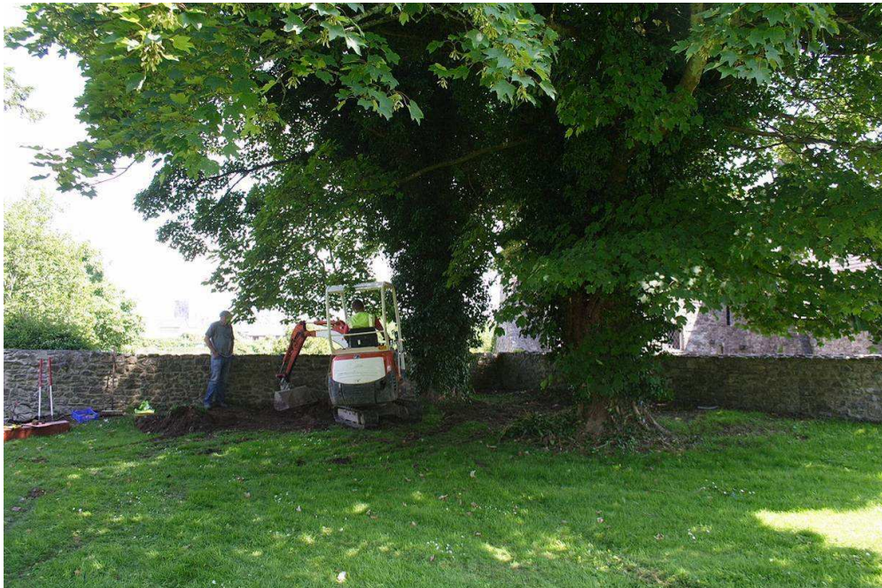
Photo 4: Excavation of the investigation pits around the base of the two mature trees thought to be causing disturbance to the churchyard boundary wall
