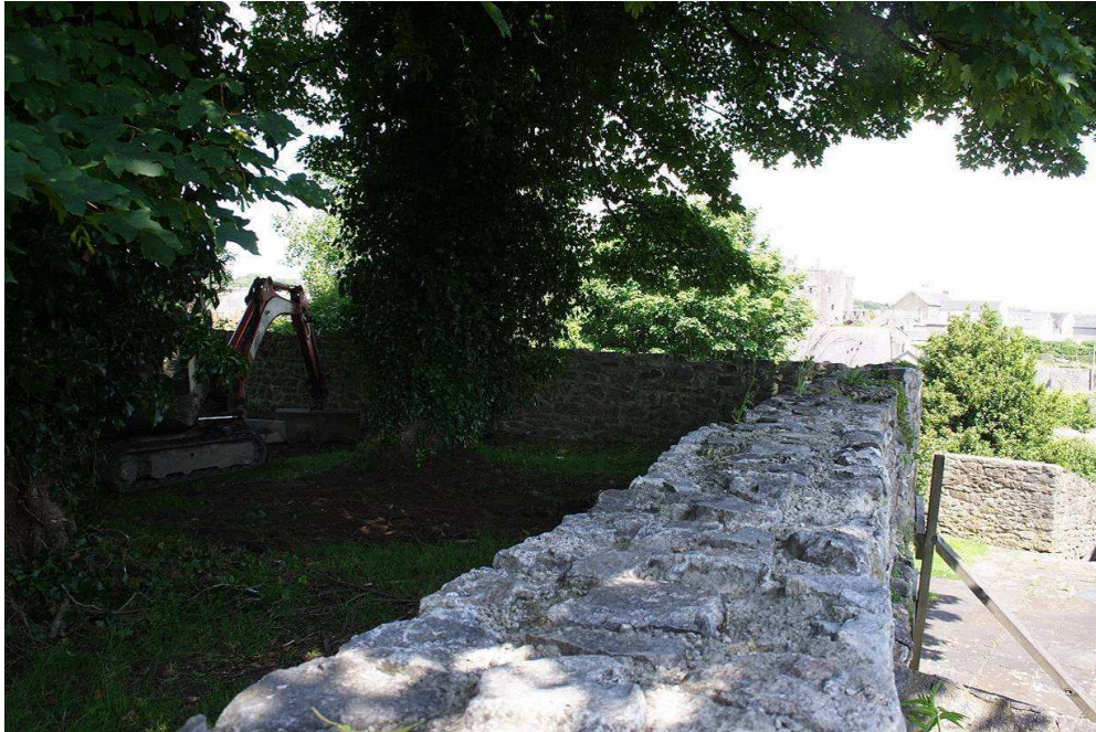
Photo 5: View along the southern boundary wall, showing the bowing in the wall structure and temporary shoring.
