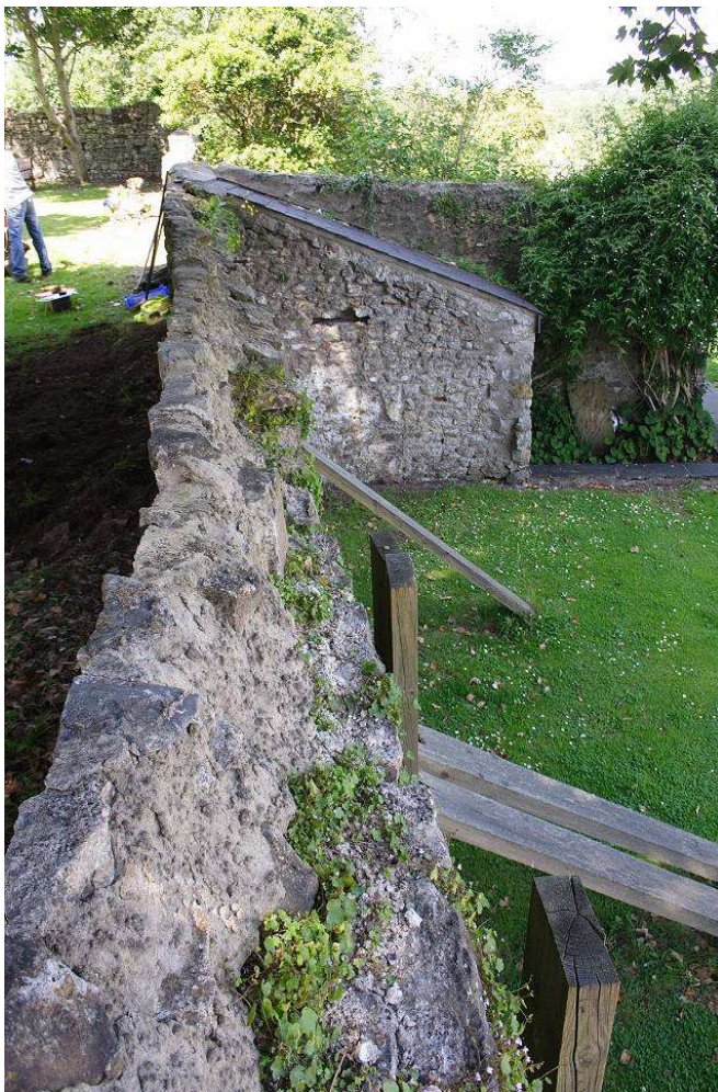
Photo 5: View along the southern boundary wall, showing the bowing in the wall structure and temporary shoring.
