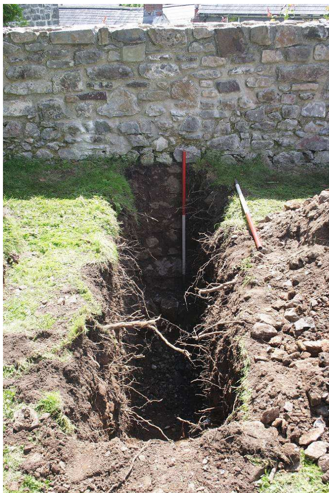
Photo 9: Typical section of investigation pits examining spread of tree roots, 1m & 0.5m scale
