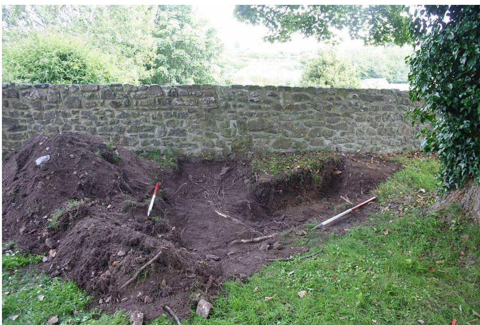
Photo 8: View looking east at two of the investigation pits examining the extent of the root action, 1m scales
