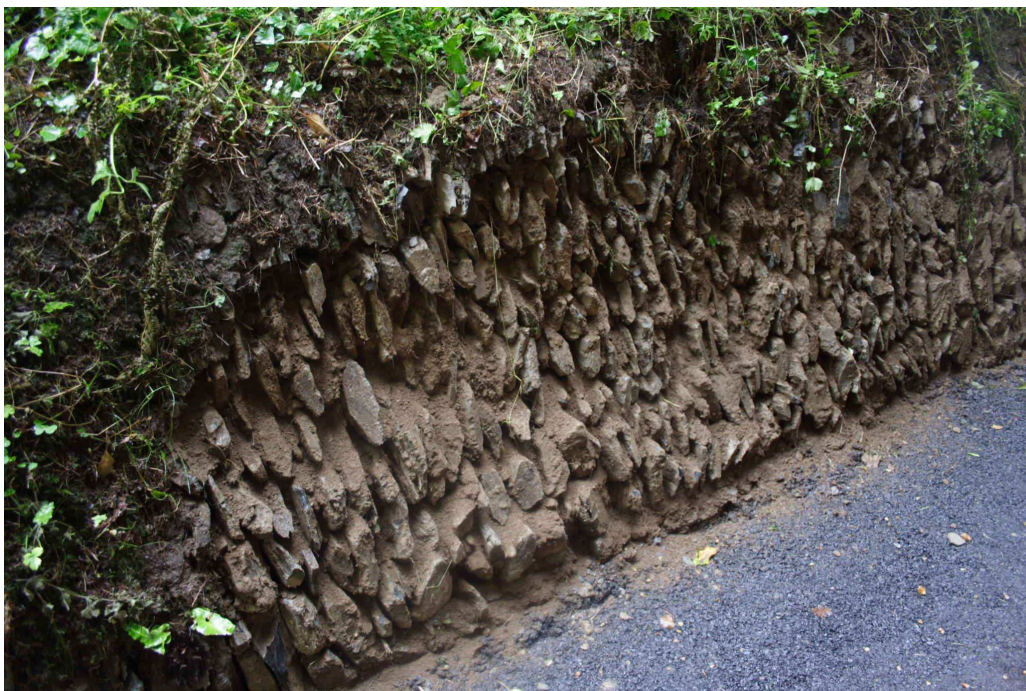
Photo 4: Detail of boundary bank stone revetting
