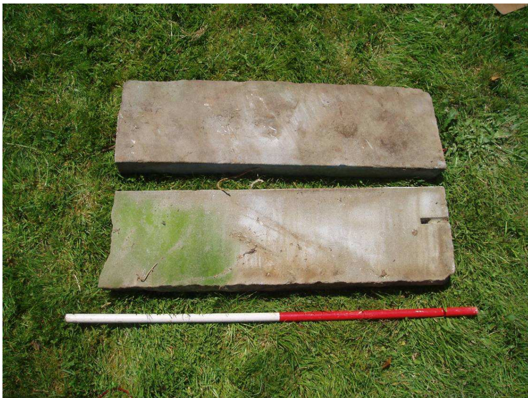
Photo 7: Dressed sandstone former window sills
