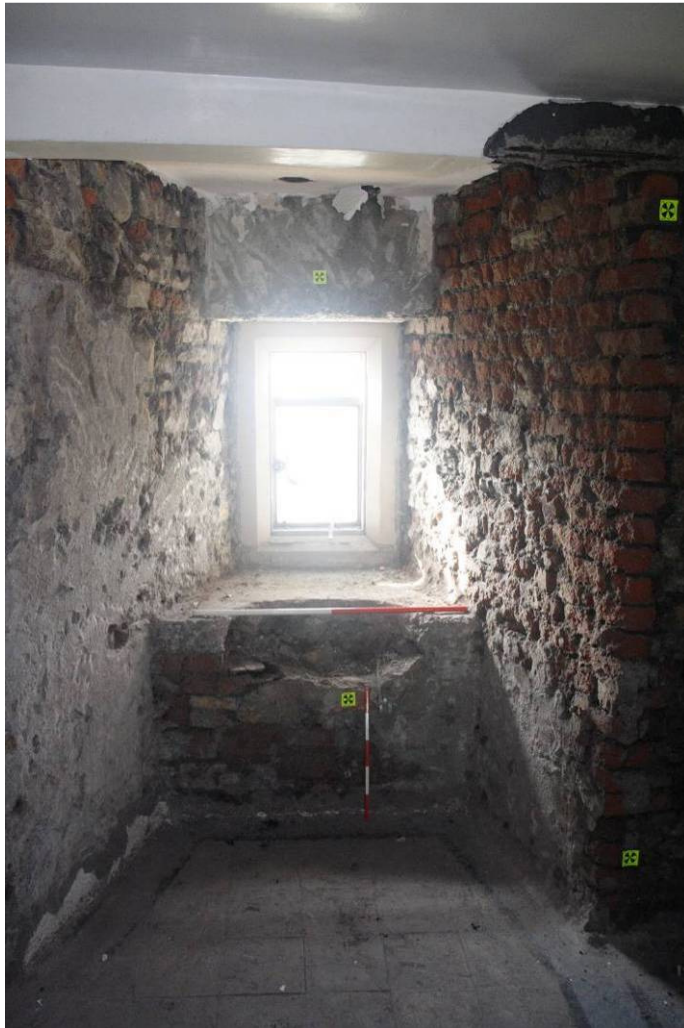
Photo 49: Window in western wall of southern room of Second Floor showing brick infill and repairs
