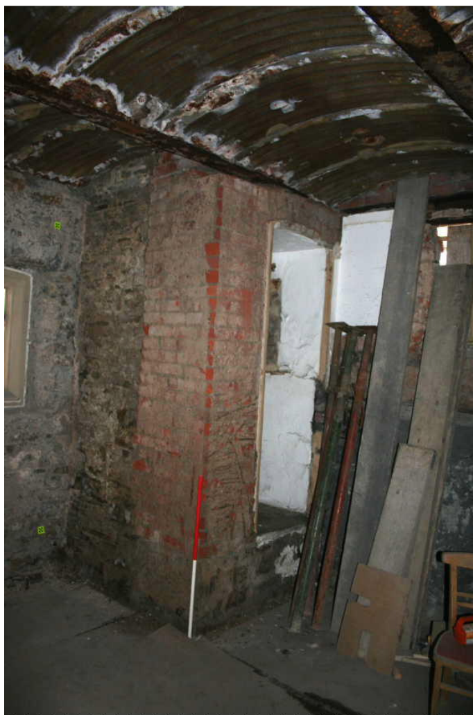
Photo 64: Northwest corner of southern room of Third Floor Level showing brick and stone projection
