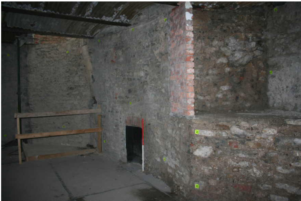
Photo 65: Southern wall of southern room of Third Floor Level showing increased wall width and step
