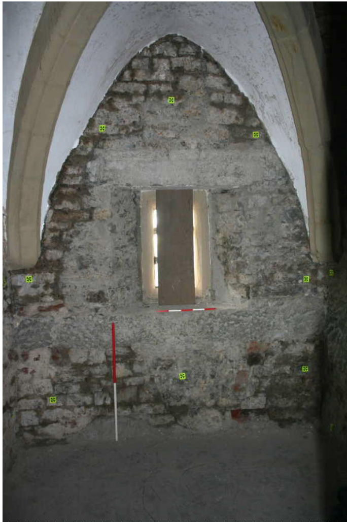
Photo 57: Window in southwestern wall of Middle Floor of Square Tower, showing concrete lintel and cill
