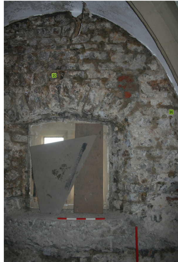
Photo 56: Window in southeastern wall of Middle Floor of Square Tower, showing stone arch and concrete cill
