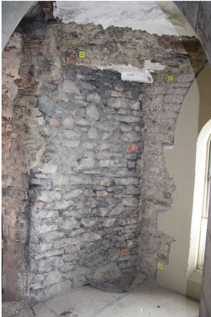
Photo 40: 1901-1904 northeastern wall blocking of possible former garderobe
