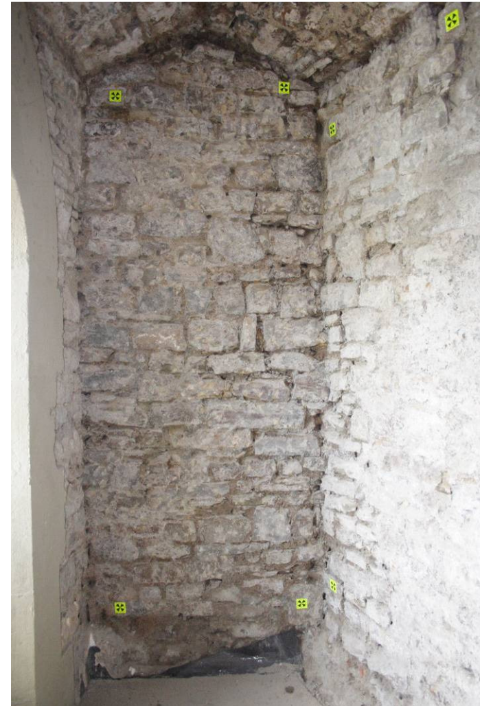
Photo 41: Possible blocked passageway, which may have led to the First Floor of Square Tower
