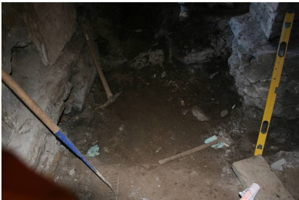
Photo 90: Excavation through floor levels below Northern Extension showing depth of make-up (not bedrock at top of photo)
