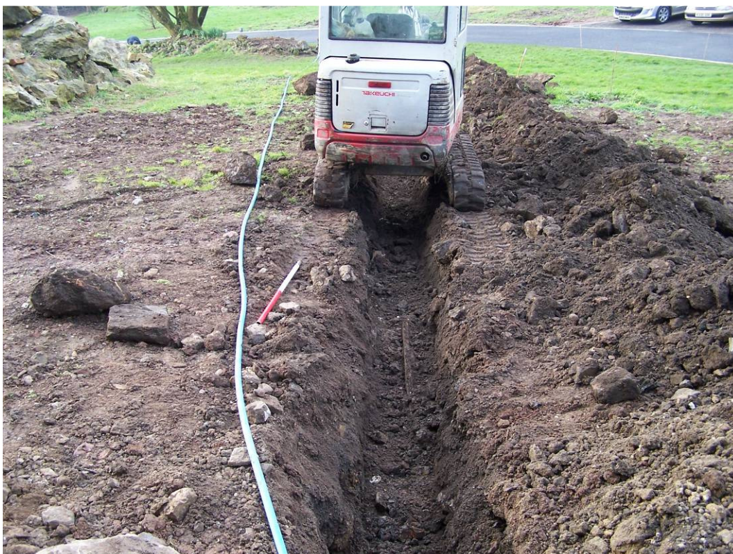
Photo 94: Service trench excavated across lawned area to west of castle (viewing southwest down-slope)
