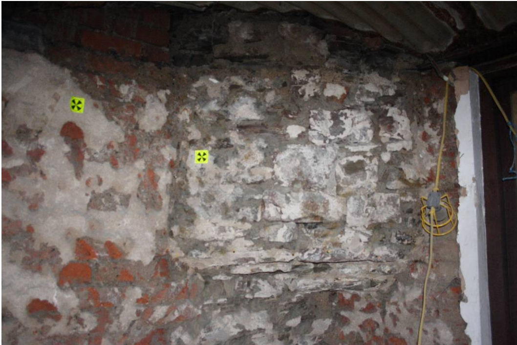
Photo 60: Corbelled base of turret projecting into northeast corner of room
