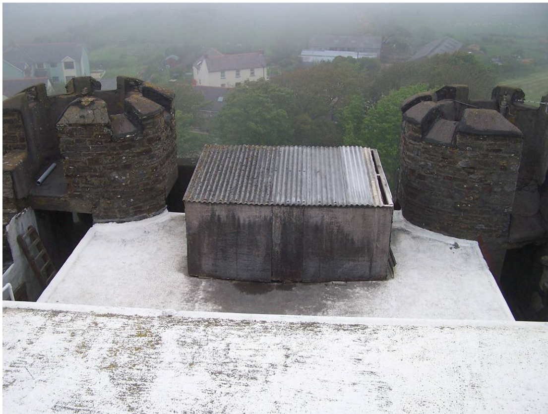
Photo 73: Southern roof layout of D-Shaped Tower and turrets prior to renovation work (asbestos roofed structure housed a water tank)
