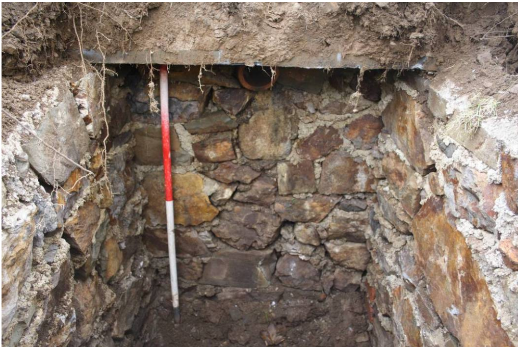
Photo 102: Stone chamber to east of castle showing drain pipe on western side
