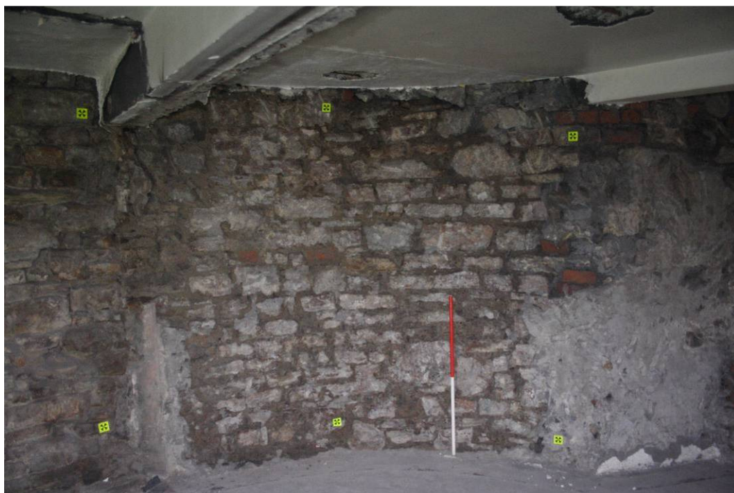
Photo 48: Southern wall of southern room of Second Floor (bricks and plastered area to west mark the reveal of the western window)
