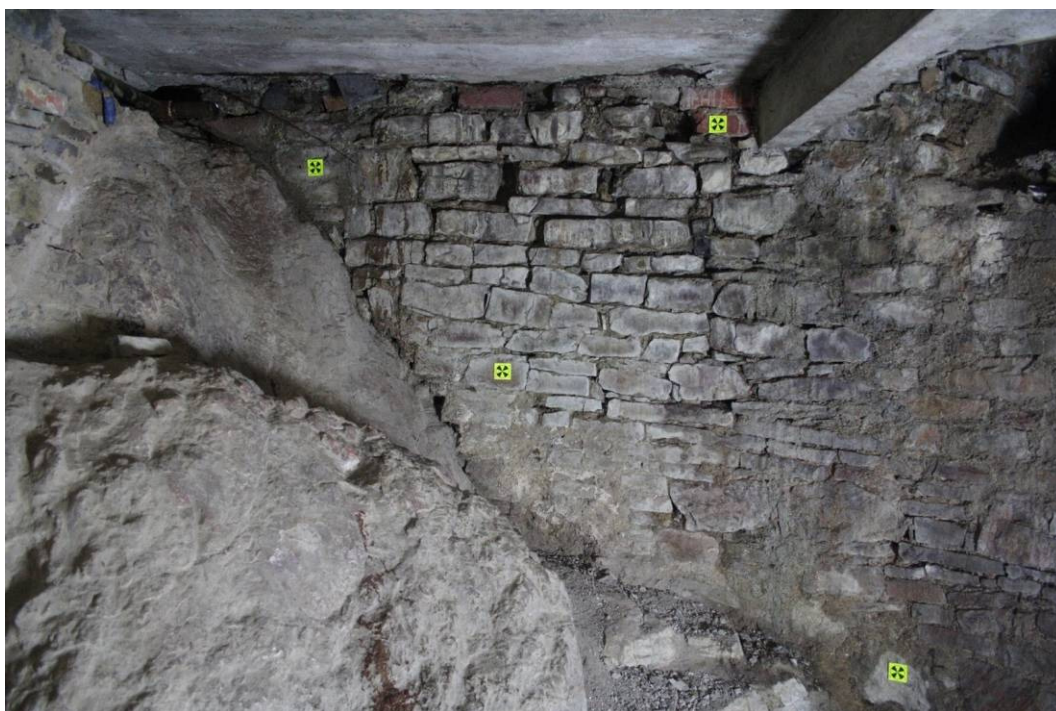
Photo 14: Southwestern outer wall of the castle built directly upon rock outcrop in southwestern part of basement (window light visible in top right)
