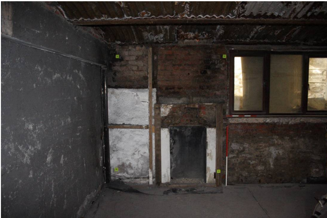
Photo 61: Southern concrete wall and western wall of brick with lower parts of stone construction, and fireplace
