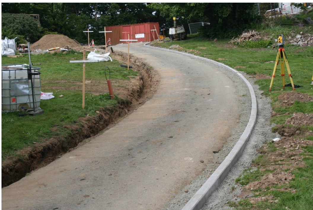
Photo 100: View north along driveway following insertion of kerbing along eastern trench, with western trench still open
