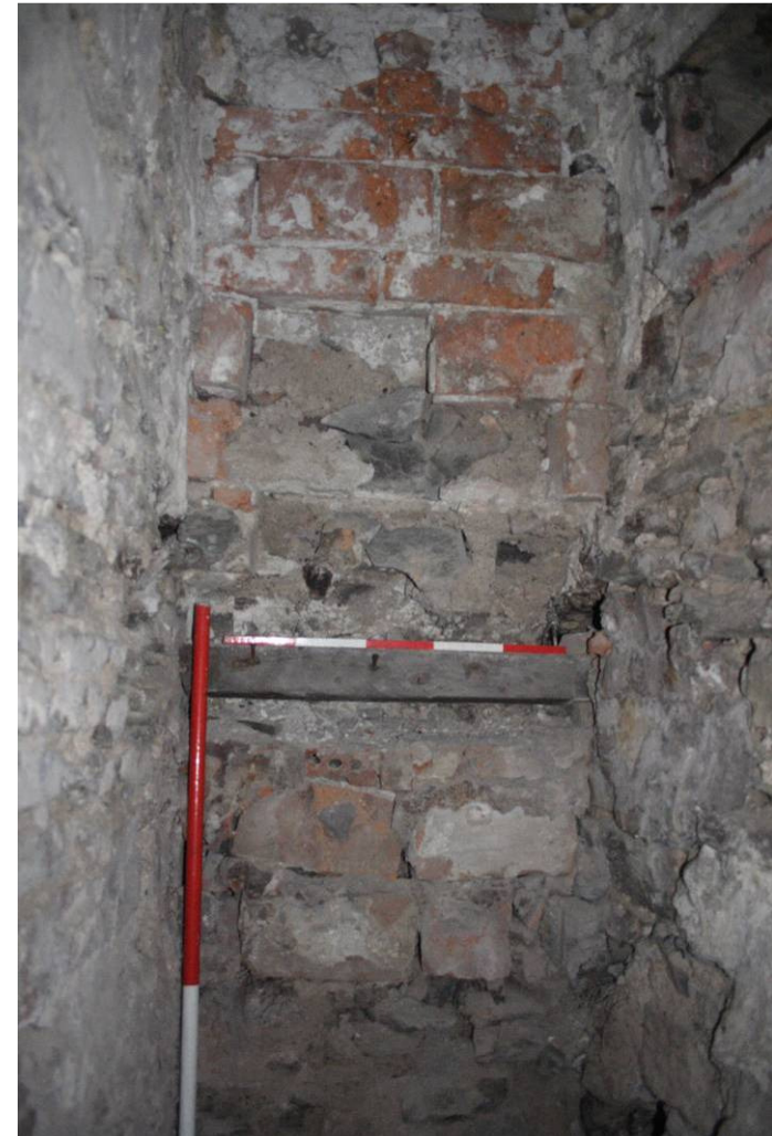
Photo 53: Northern wall within Garderobe in Stair Extension showing brick patched walling, with small vent to east
