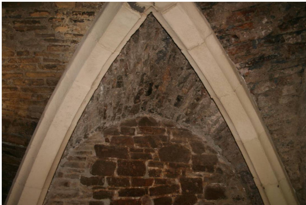
Photo 54: Part of ribbed and vaulted ceiling of Middle Floor of Square Tower
