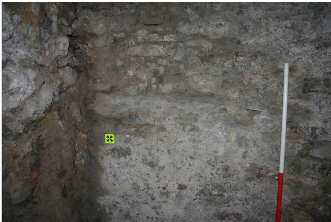
Photo 68: Stone lintel and blocked aperture below above step on southern wall
