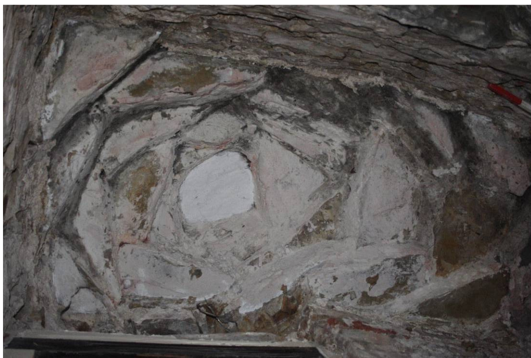
Photo 51: Corbelling forming small stone domed ceiling within garderobe
