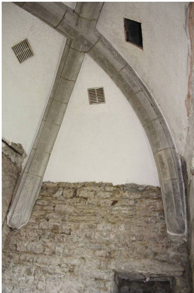
Photo 34: Part of the replica ribbed and vaulted ceiling of the Lower Floor of the Square Tower, facing northeast with small alcove below
