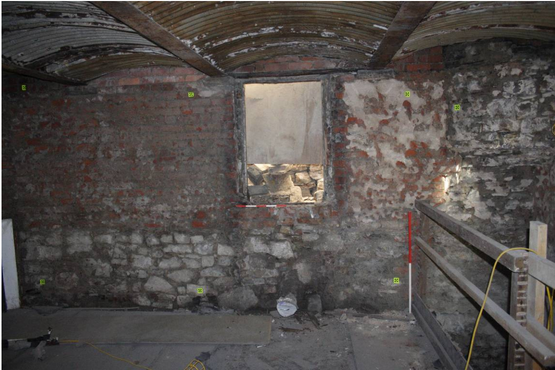
Photo 62: Northern wall of northern room showing stone and brick built walls, with stone turret base in northeast corner
