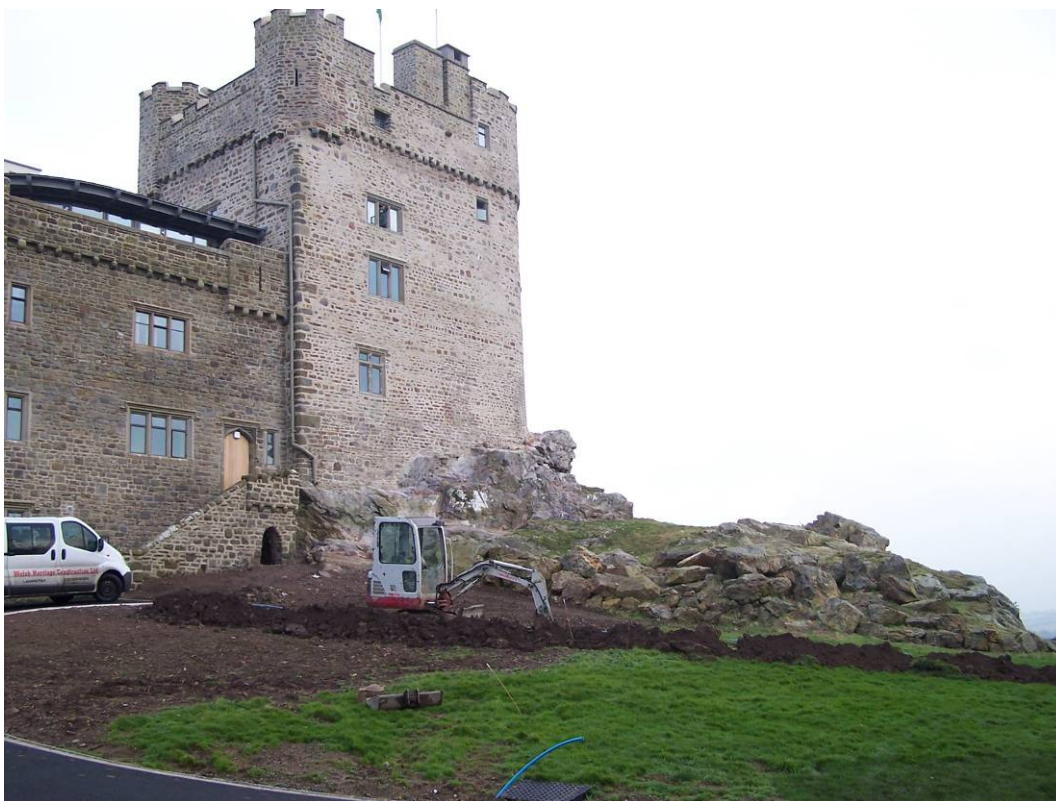
Photo 93: Service trench excavated across lawned area to west of castle with rock outcrop behind
