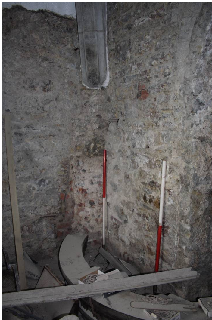
Photo 37: Northwest corner of Lower Floor of Square Tower showing projecting stonework
