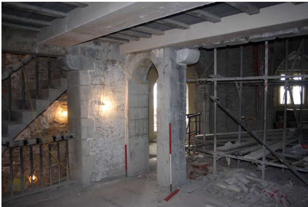
Photo 24: Wall segment on the inside of the stair way from the Basement / Ground Floor level showing stone corbels and archway
