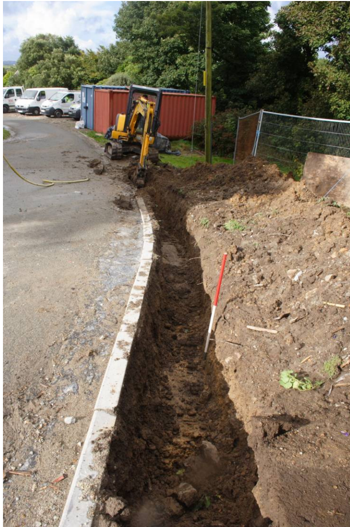
Photo 92: Service trench around perimeter of driveway
