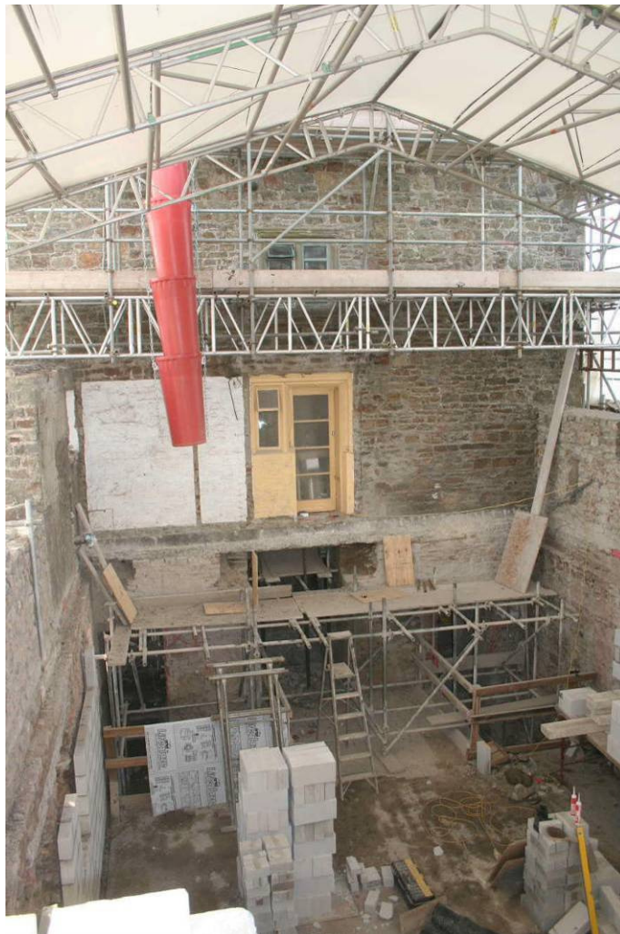
Photo 81: External view of northern facade of castle showing doorway from First Floor Level of D-Shaped Tower and opening below (taken following removal of roof structure for Northern Extension)
