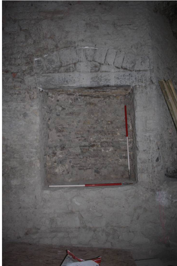
Photo 31: Rectangular recess within south wall of first floor
