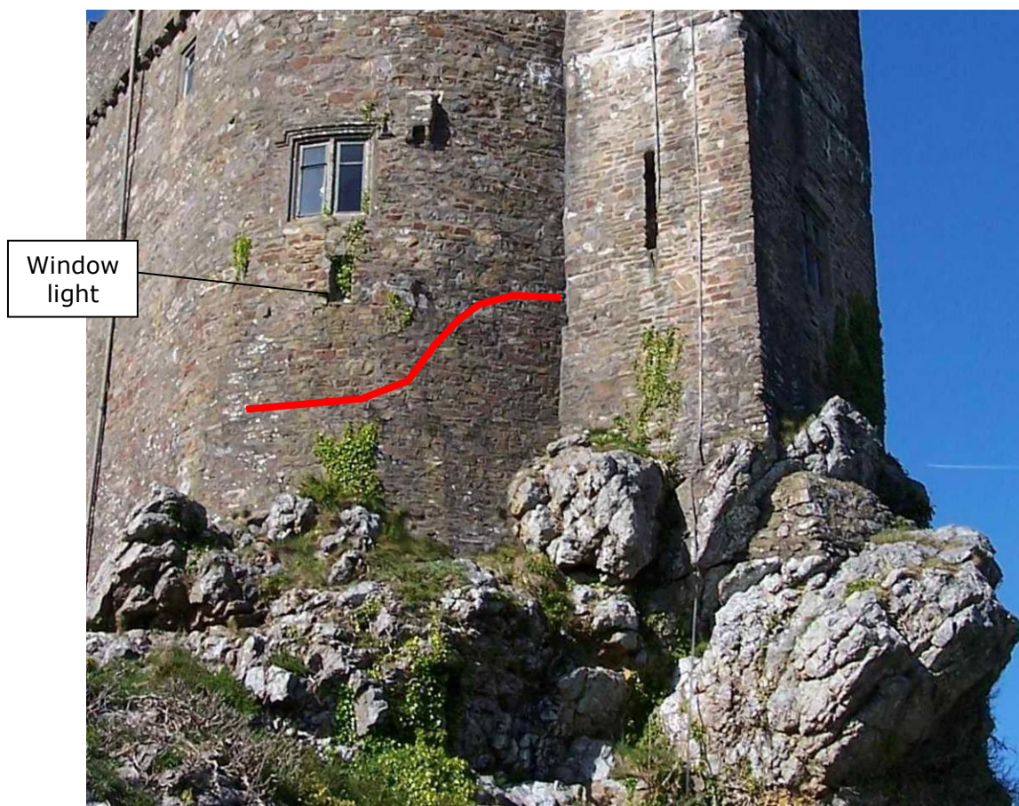
Photo 15: Approximate height of basement floor and rock outcrop (red line) in relation to the exterior southwestern wall of the castle
