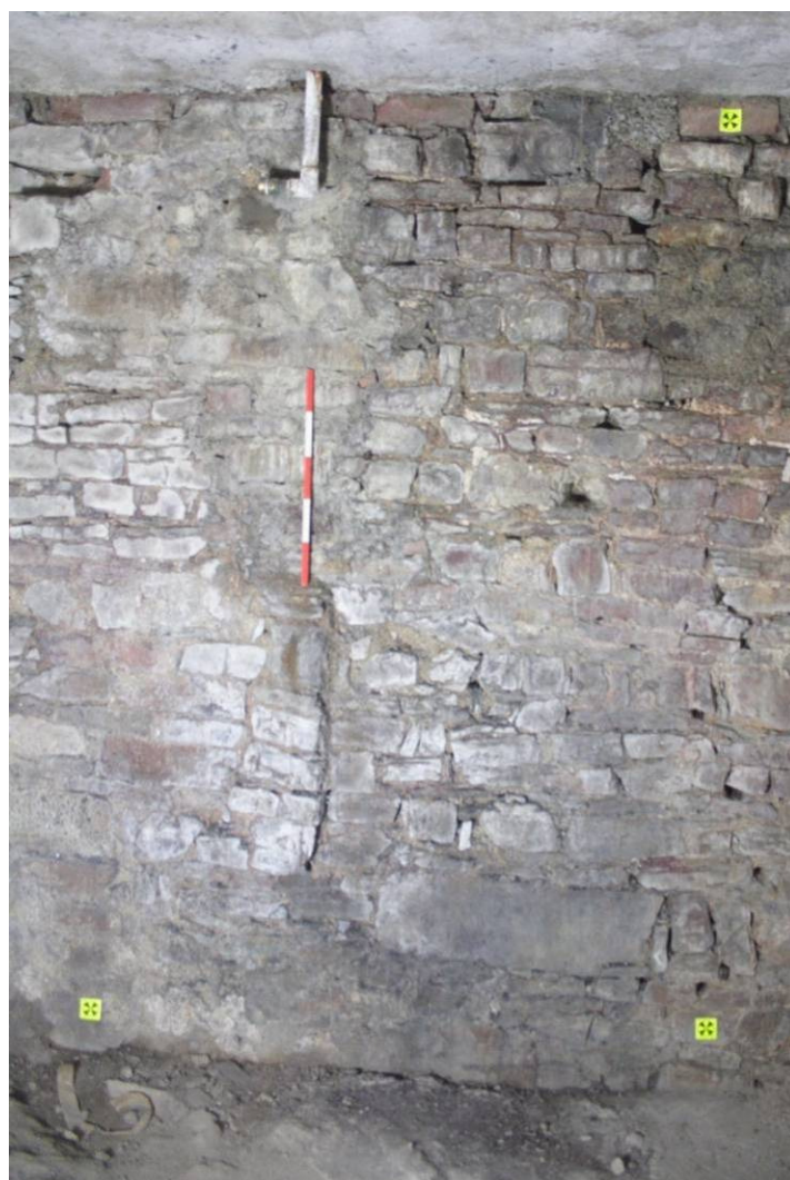
Photo 16: Small area of projecting stonework on eastern internal wall (located directly below 0.5m ranging rod)
