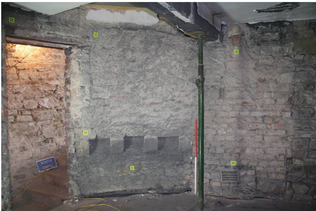
Photo 47: Southeastern part of southern room of Second Floor showing corbels and section of brick infill
