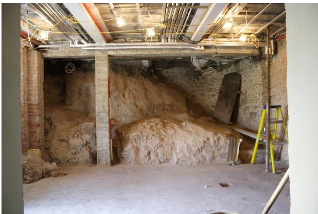
Photo 17: Rock outcrop in southern part of Basement / Ground floor following removal of dividing walls (2m ranging rod against retained concrete pillar support)
