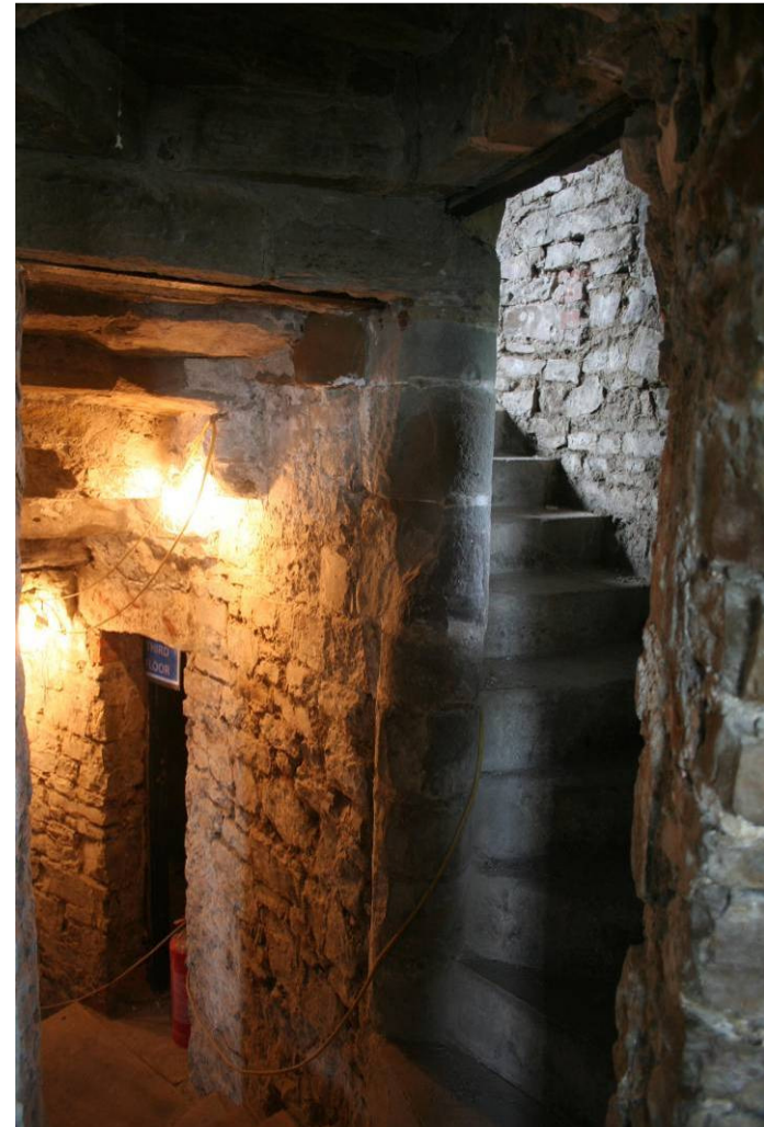
Photo 58: Curving stone stairs and newel from Second to Third Floor of the D-Shaped Tower
