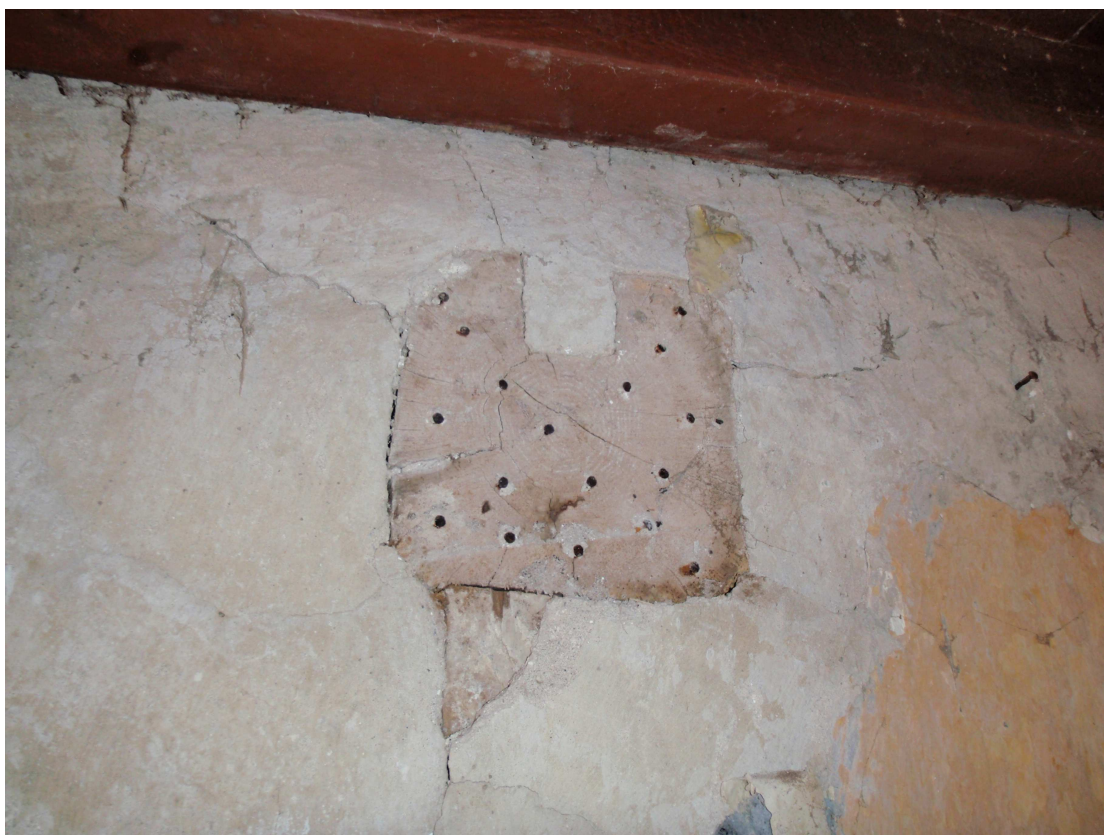
Part of a cruck truss visible in the front (south) wall.
