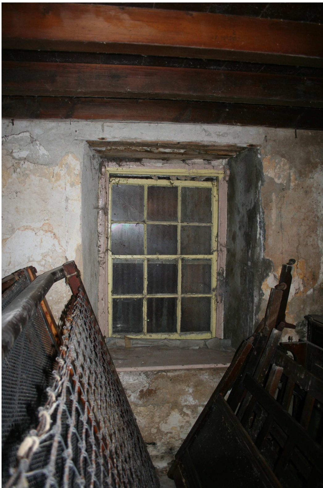
Sash window – the absence of horns probably indicates a c. pre-1840 date.
