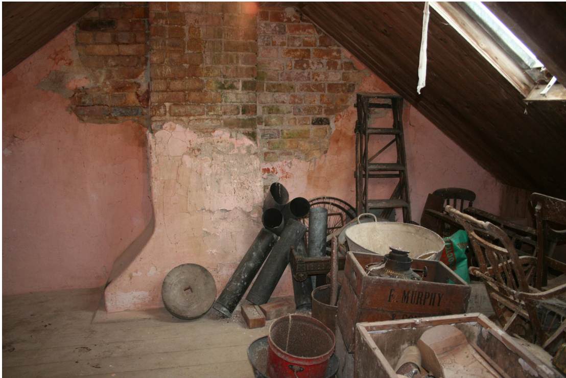
The brick chimney shaft above the main inglenook fireplace replaced an earlier wicker hood recorded by Peate.
