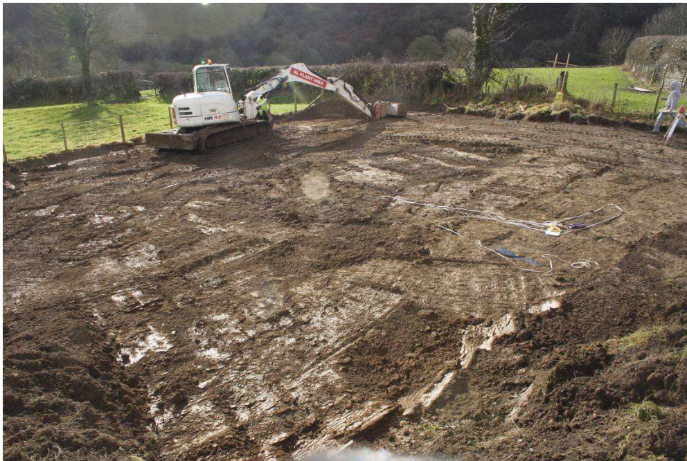
Photo 6: South east view of development area following topsoil stripping
