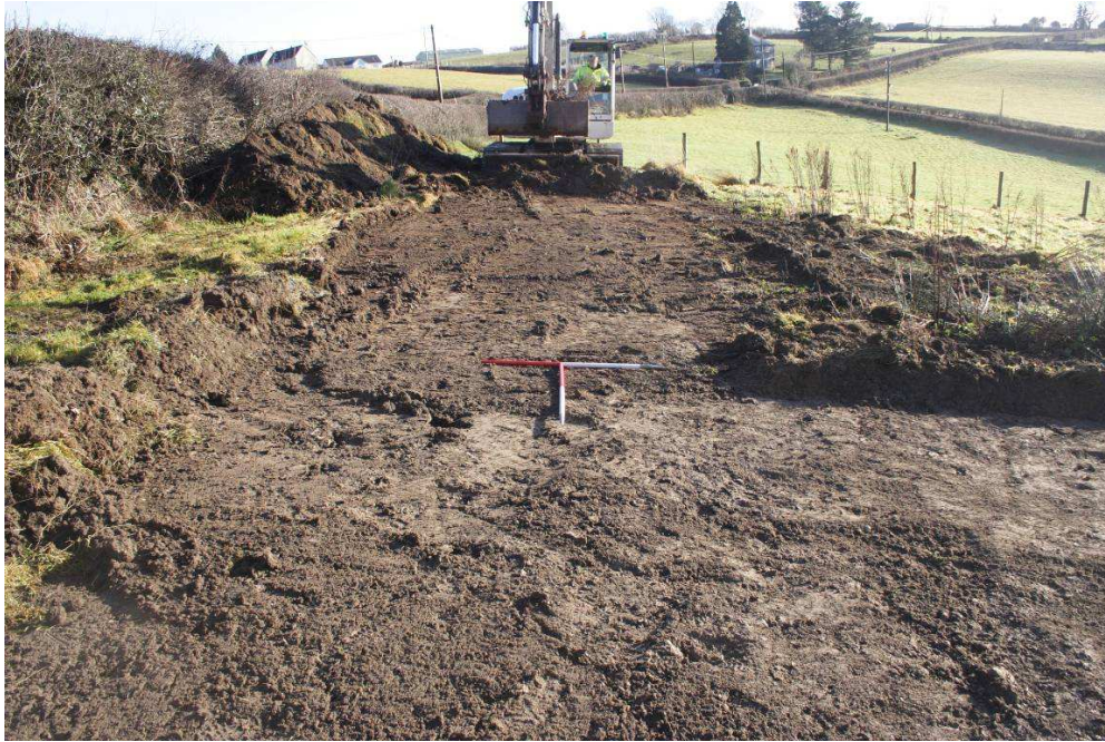
Photo 5: East facing view of development area during topsoil stripping
