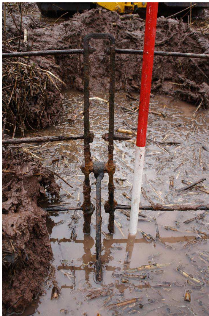
Photo 8: Detail of fixing metal post and brace
