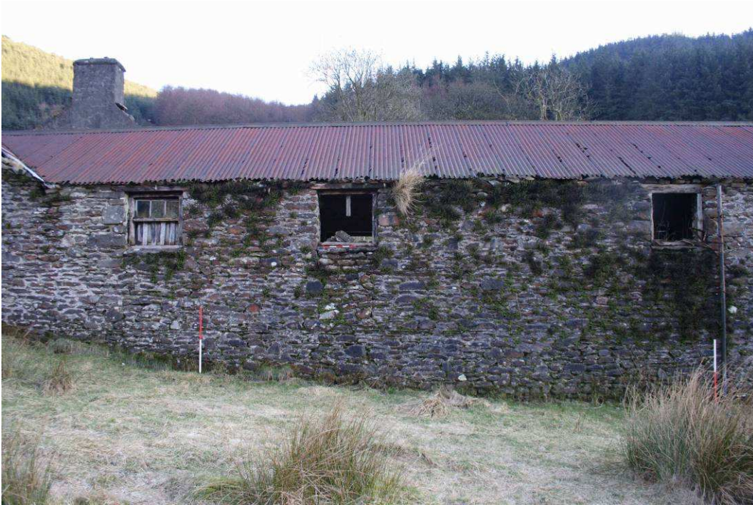
Photo 14: NW facade of animal sheds showing windows and raised level of structure
