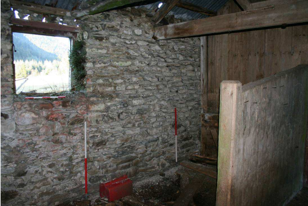
Photo 21: Inside of animal pen showing window and partition walls
