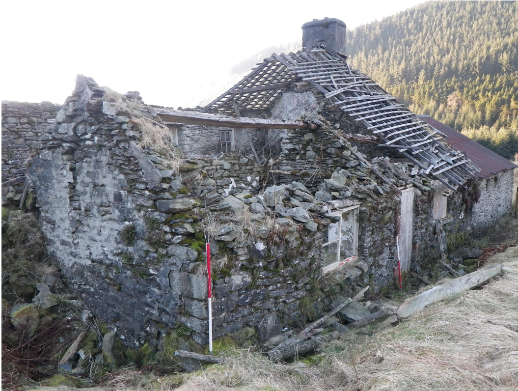
Photo 6: SE end of extension area showing separate gable end and ridge beam
