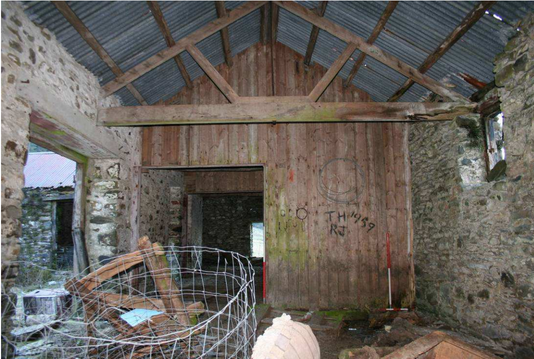
Photo 19: Timber partition wall in middle of animal shed, showing exposed roof truss
