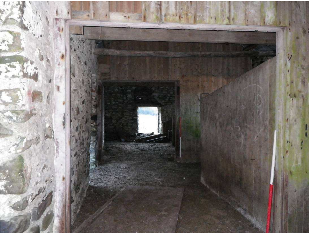
Photo 20: Second timber partition wall and lower timber wall forming an animal pen in the central part of the animal shed
