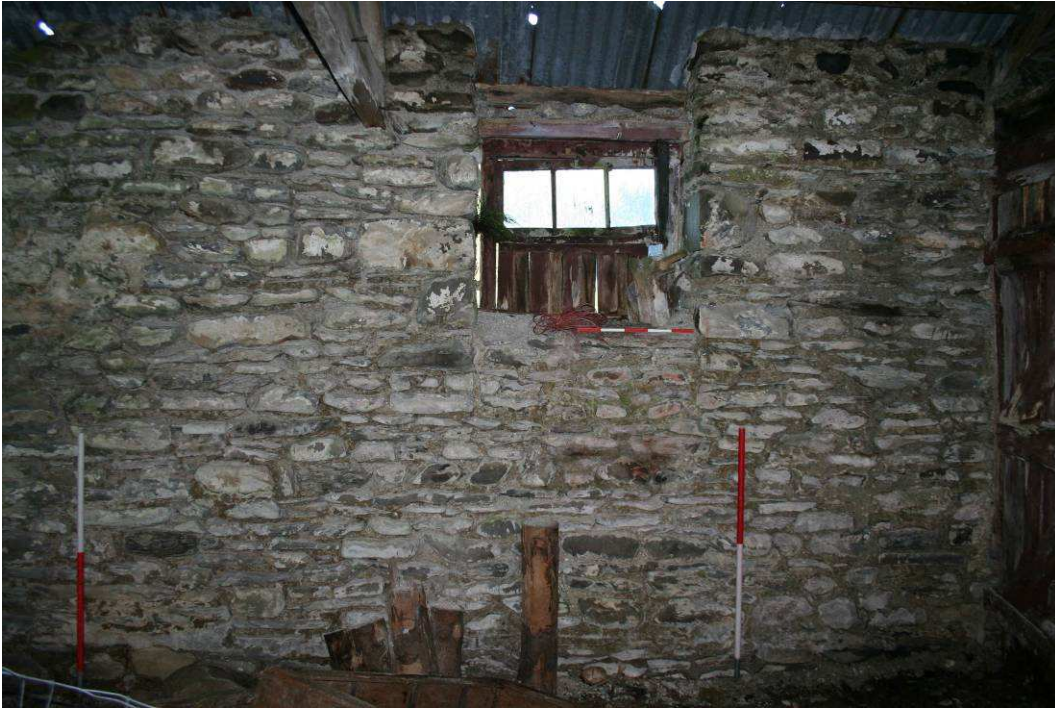
Photo 16: Internal view of surviving louvered window, and showing partially blocked opening below
