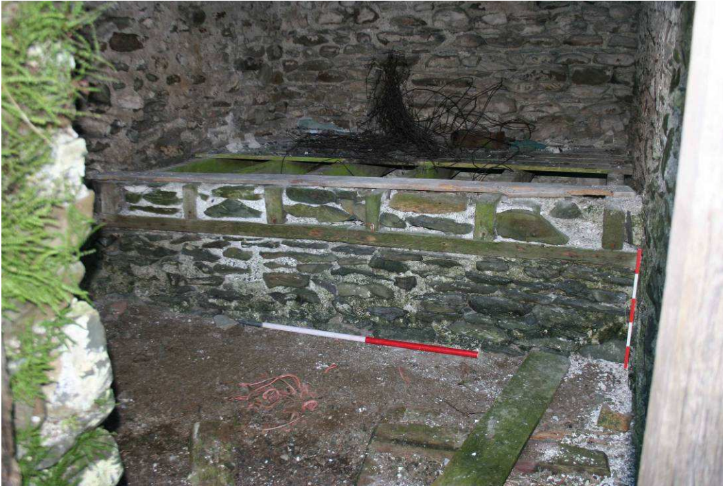
Photo 28: Raised area within store shed, providing access to pigsty below
