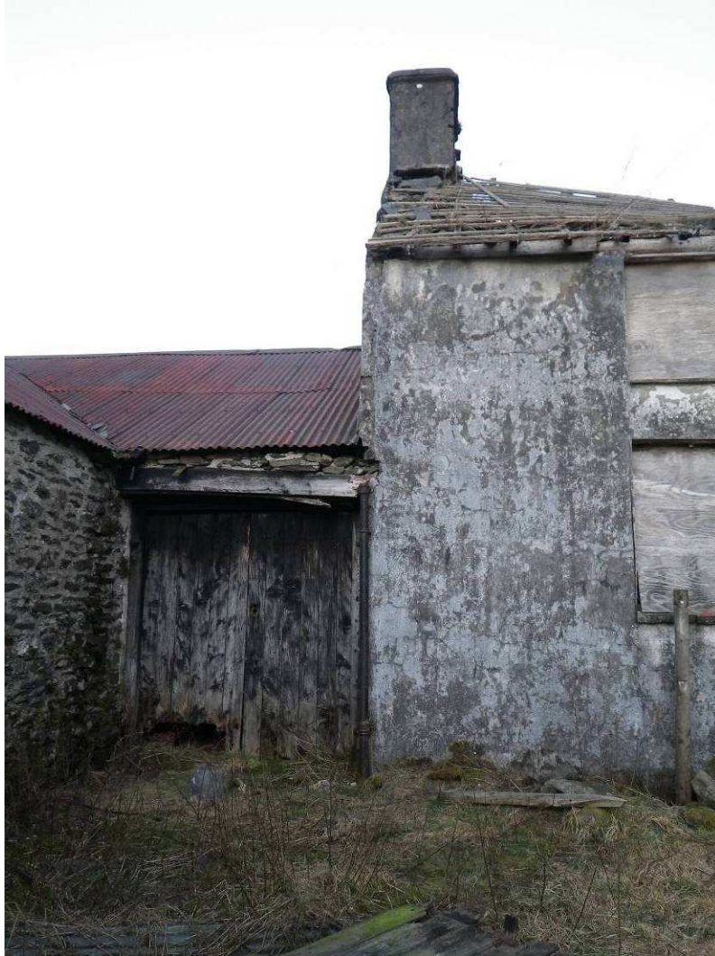
Photo 7: Doorway into barn extension on NW facade, with the main farmhouse to the right, clearly showing the difference in wall heights
