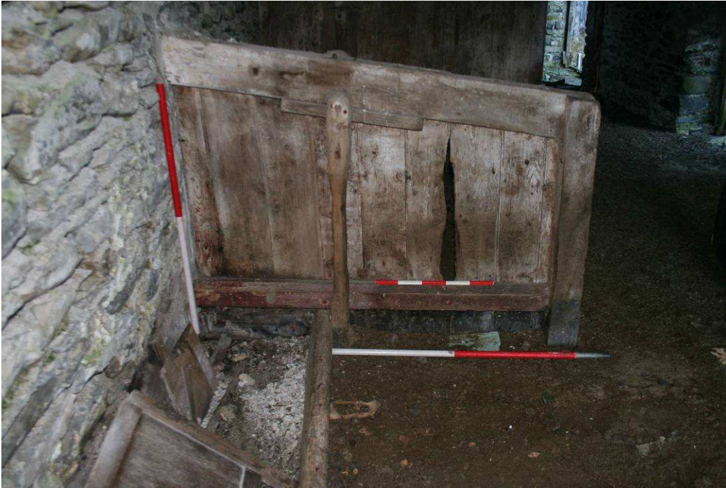
Photo 25: Detail of low level stall partition, tethering post and remains of timber trough
