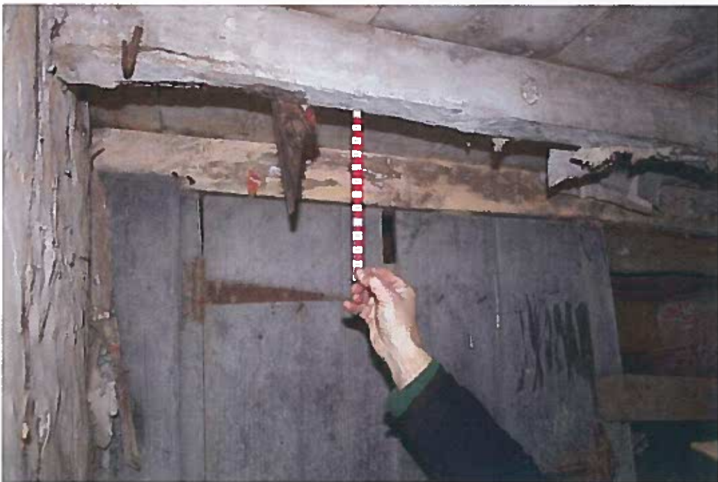
Photo 24: Detail of peg and notch to hold door open, Room 3.
