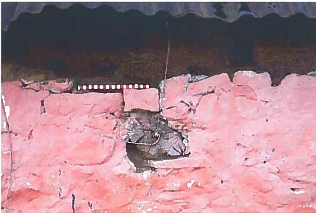
Photo 10: Protruding timber ceiling beam, NW wall.
