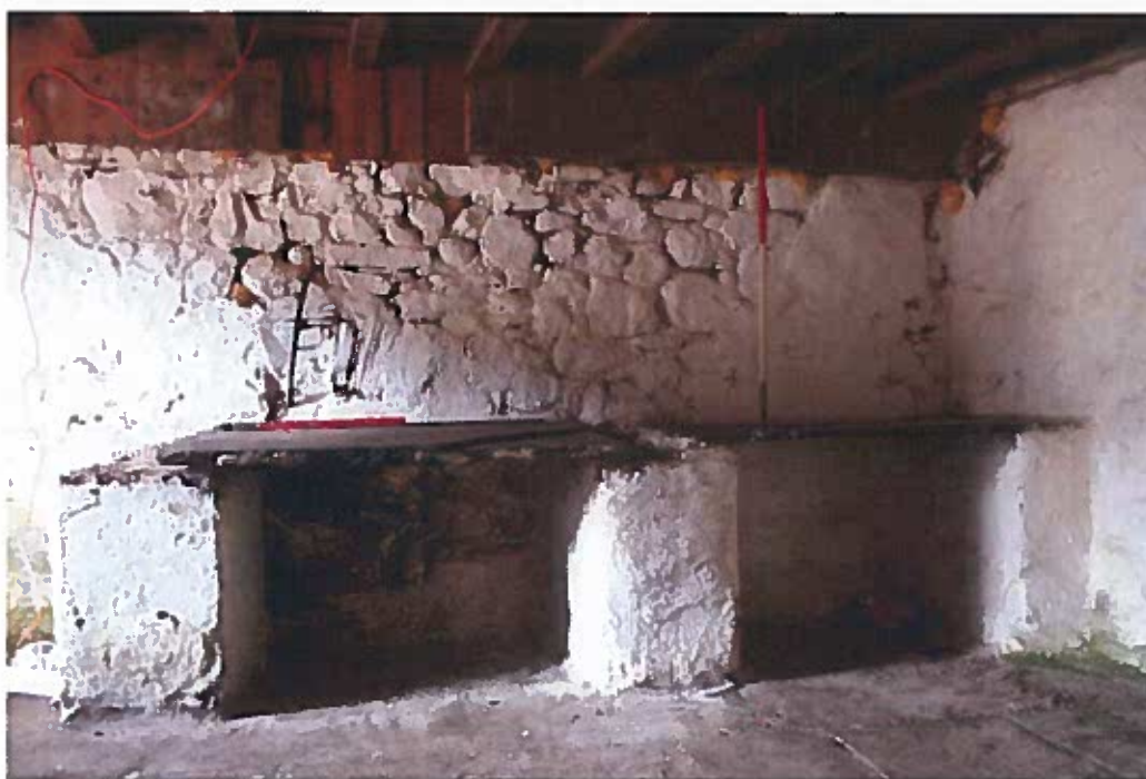
Photo 15: Slate top work area with retaining arch of fireplace visible.
