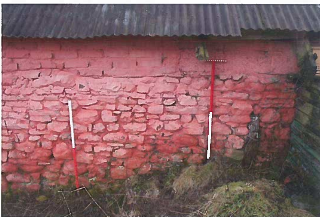
Photo 12: Protruding cruck, with inserted concrete blockwork above, NW wall.
