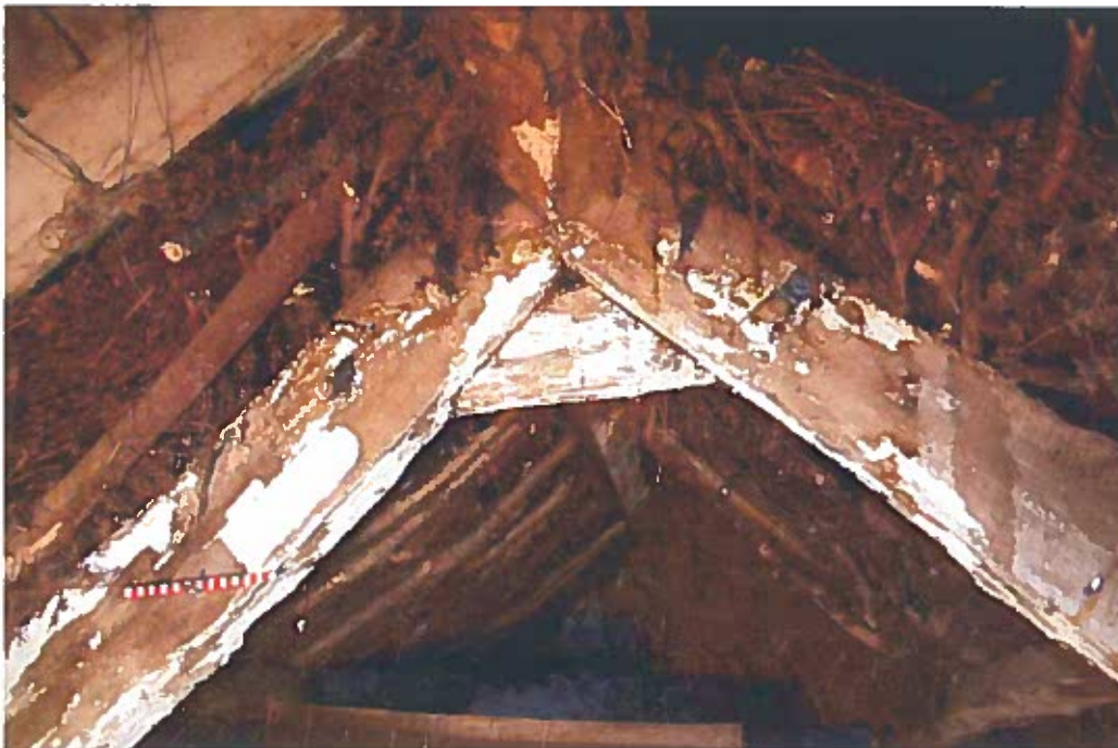
Photo 37: Detail of top of cruck, Room 7.
