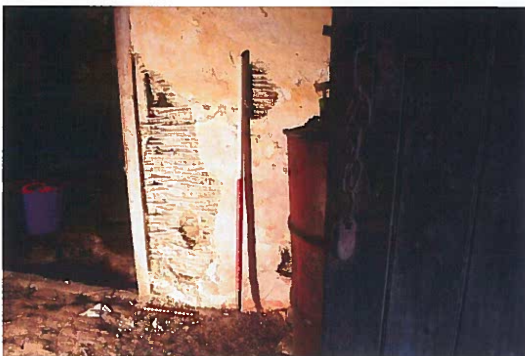
Photo 26: Detail of wattle and plaster partition wall between Rooms 3 and 4.
