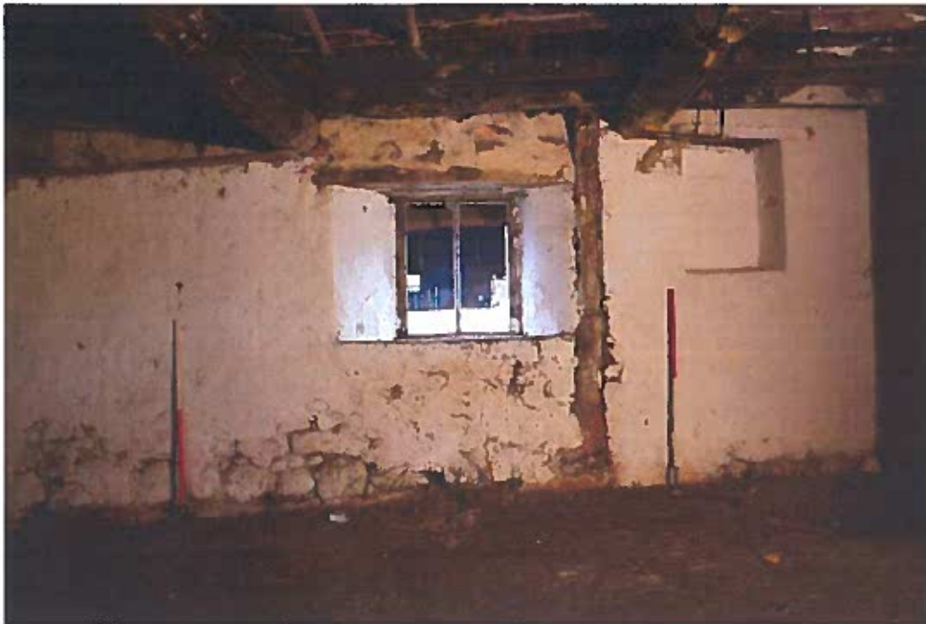
Photo 17: Window, cruck and cupboard within NW wall Room 2.
