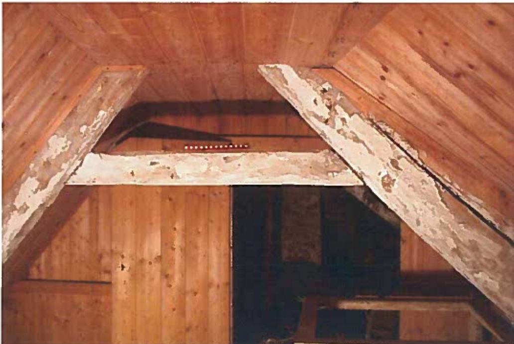
Photo 43: Cruck frame within Room 8.
