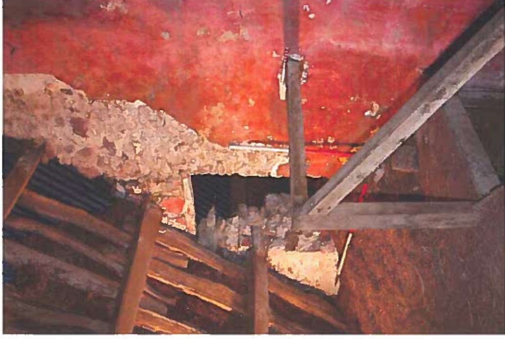
Photo 33: Doorway inserted into former cottage gable end, Room 5.
