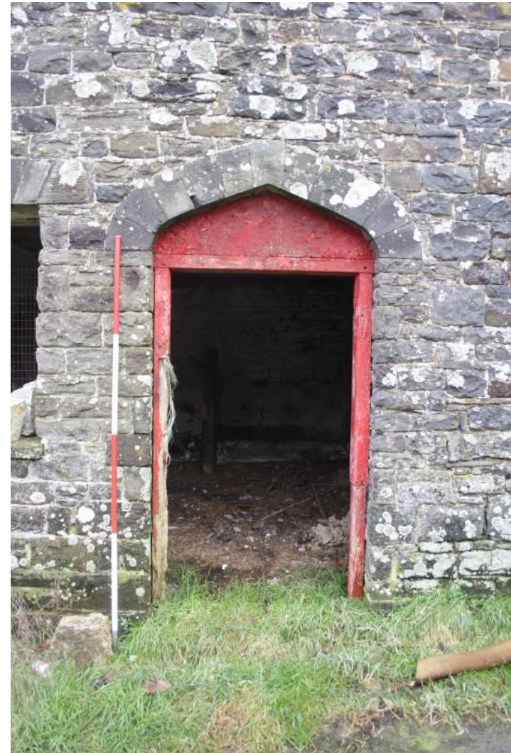
Photo 23: Detail of 'Tudor' style four centred arch headed doorway, NE wall Building 5
