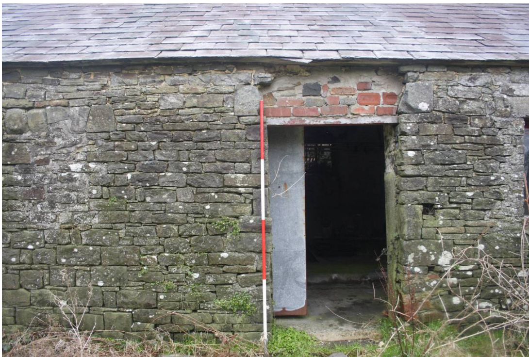
Photo 14: Detail of opening with brick replacement head, SW wall Building 3
