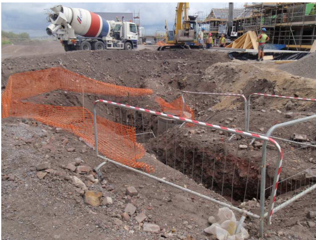
Photo 1: Excavation for sewer, in which tunnel was discovered
