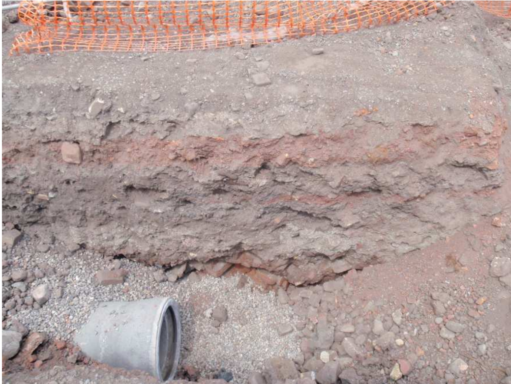
Photo 3: Made ground overlying the buried structures
