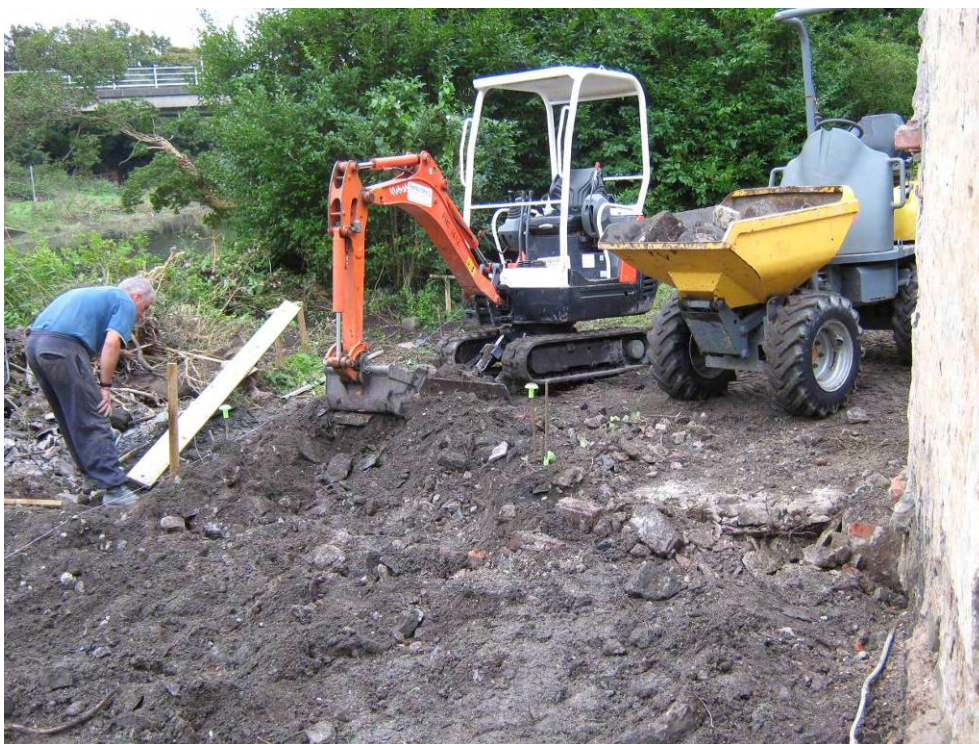
Photo 7: Site area, viewing south-east, following demolition of former sheds and removal of upper overburden (flooring and concrete) and insertion of piles
