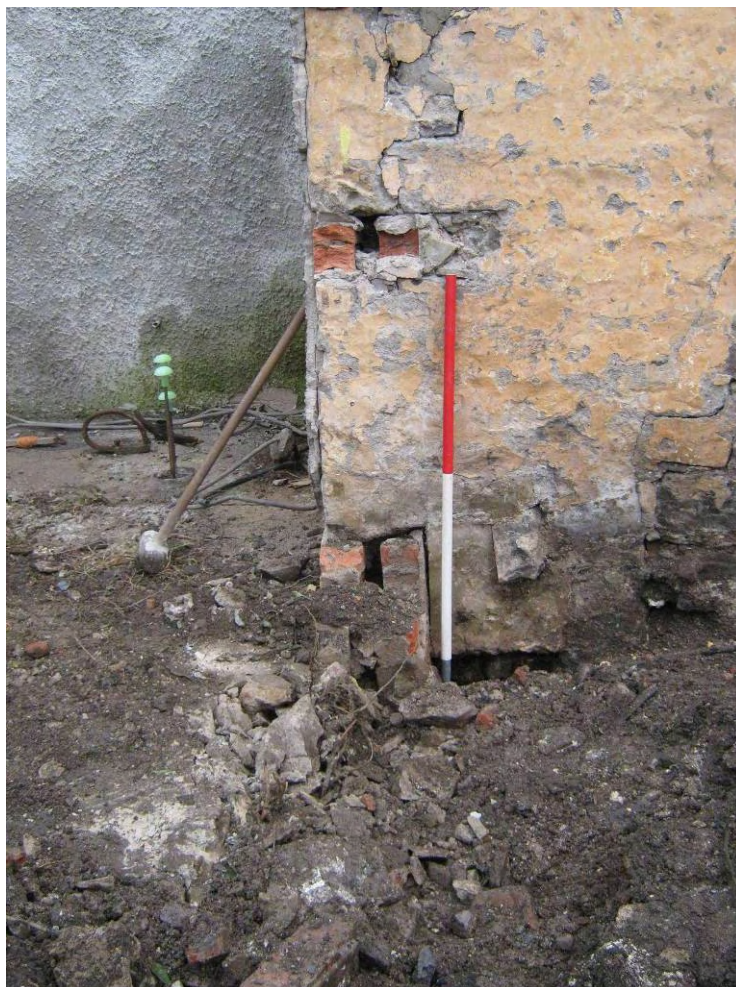
Photo 5: North-east facing end wall of 52 Hanover Quay, showing bricks inserted into stone wall to key in former extension
