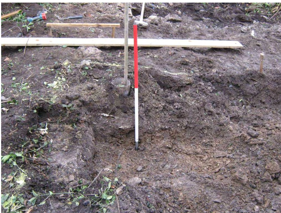
Photo 8: North-western corner of excavation area following excavation to required depth for new extension. Section shows heavily disturbed upper layers, with redeposited clays and stone (lighter fill) towards base
