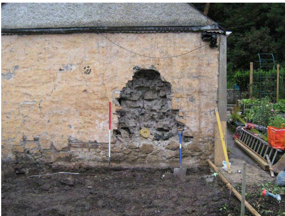
Photo 6: North-west facing wall showing partial breach in wall, which wall form access into new extension. Note the stone rubble construction of the wall, with some earlier brick inserts to the lower left
