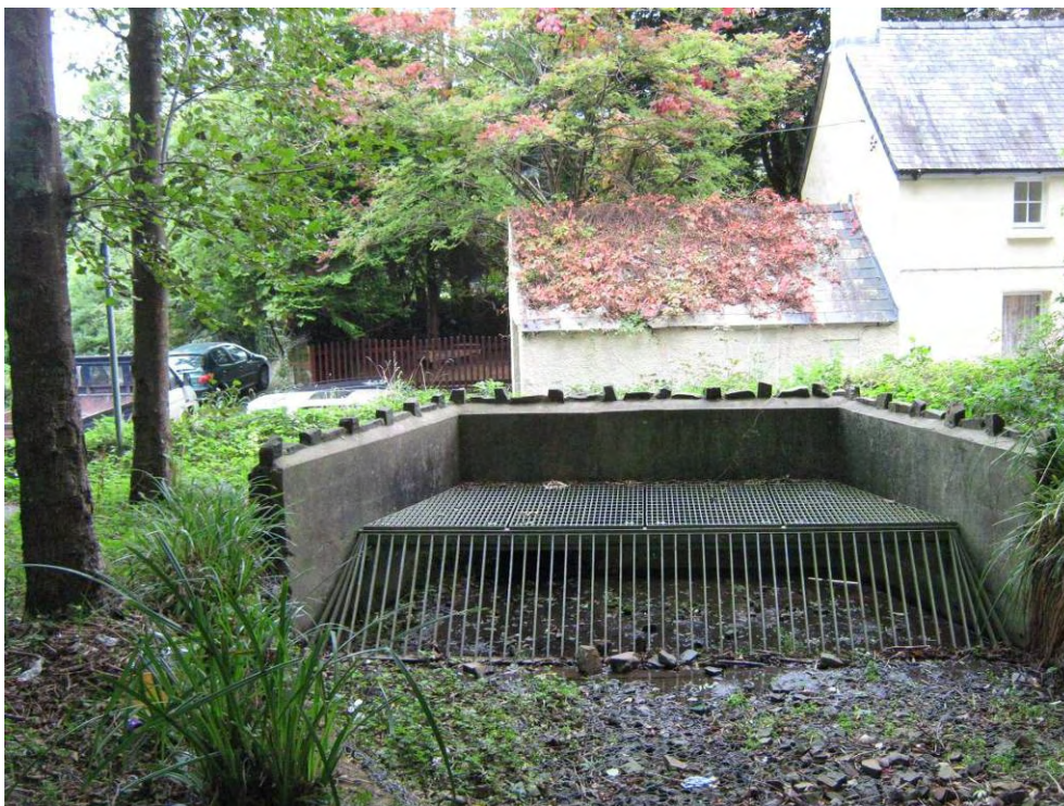
Photo 3: Culvert cover taking stream under Quay Street (viewing east)
